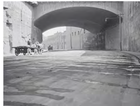
Hickson Rd, Munns St bridge, 1930s. Source: City of Sydney Archives
