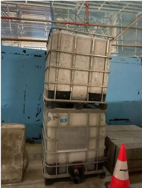
Plate 11 – Chemical containers on not properly stored / banded.
