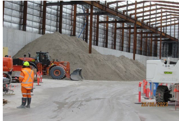
Figure 1 2 Ongoing cladding of the frame of the spoil shed. (The Bays). Use of the shed for storing spoil from the TBM.
