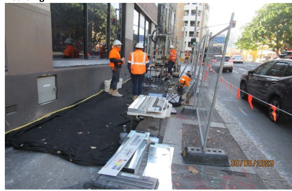
Figure 4.4 Hunter St West: Borehole drilling for monitoring
