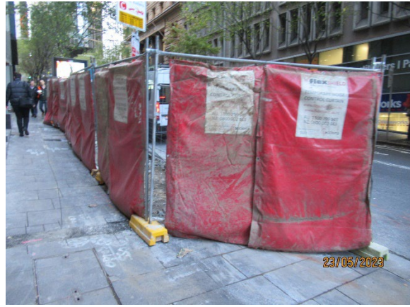
Figure 4.6 Hunter Street East: Driveway construction conducted OOHs.
