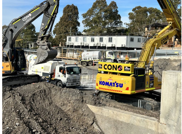
Figure 3.2: Westmead site – Spoil load out with street sweeper cleaning hard stand
