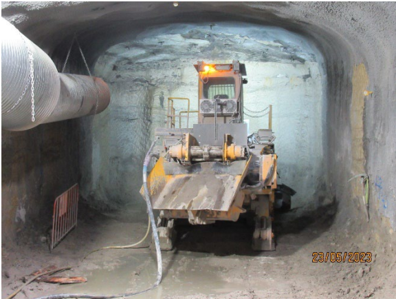
Figure 4.5 Tunnel decline: Ongoing excavation by road headers.
