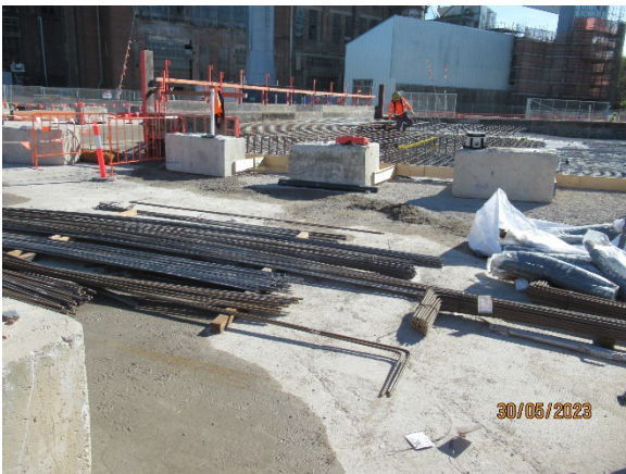
Figure 4.7 The Bays: Concrete works for base of the WTP
