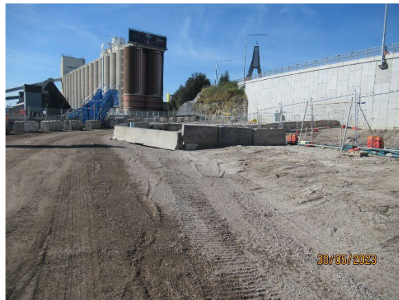
Figure 4.8 The Bays: General site establishment activities
