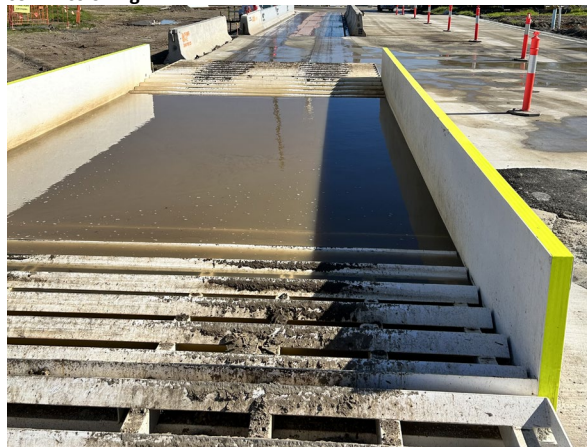
Figure 3.10 – Clyde MSF Site – Wheel washing prior to entering Wentworth Street
