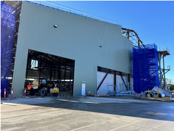
Figure 3.7: Rosehill Site – Spoil storage and loading shed nearing completion
