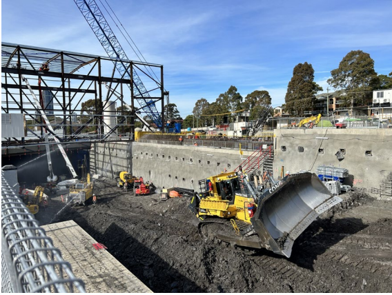
Figure 3.1: Westmead Site – Station Box excavation with acoustic shed construction
