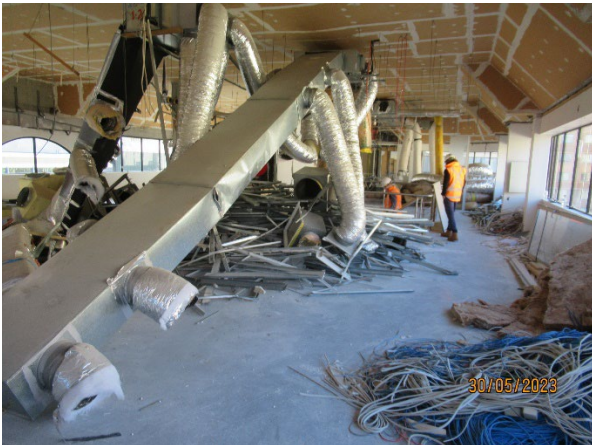
Figure 4.1 Pyrmont East: Ongoing soft strip of building interiors
