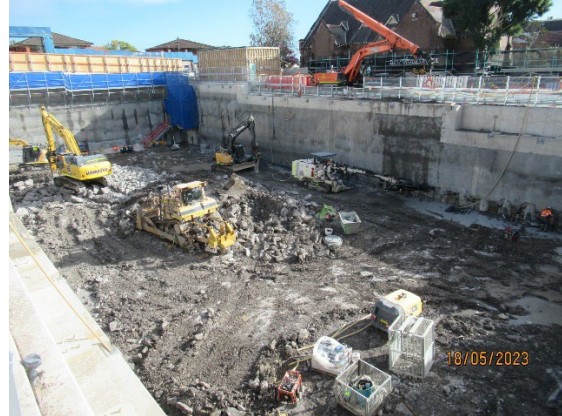
Figure 1 6 Ongoing excavation of the west shaft (Five Dock-west).
