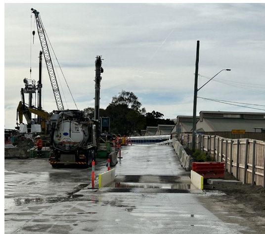
Figure 3.6: Clyde Dive site – Wheel wash in place and operational
