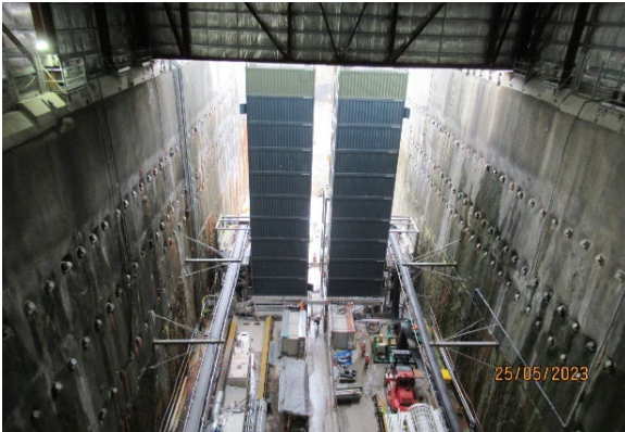
Figure 1 1 Vertical conveyor supports in the Station Box (The Bays)
