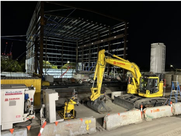
Figure 2.3: Westmead Site – Station Box excavation with acoustic shed construction evening works
