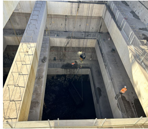
Figure 2.10: Rosehill Site – Launch Box excavation
