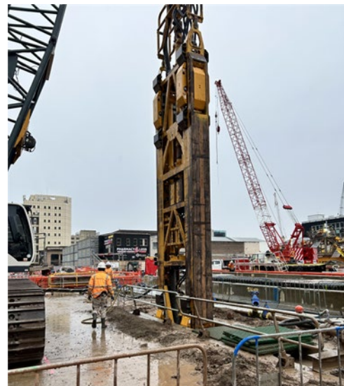
Figure 2.6: Parramatta Site – D-Wall excavation with grab
