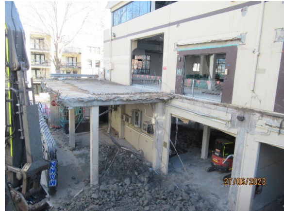
Figure 3.2 Pyrmont East: Hard demolition ongoing using pulverisers
