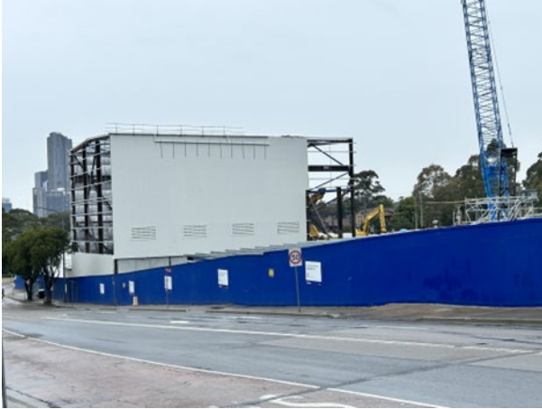
Figure 2.1: Westmead Site – Westmead hording and acoustic shed construction
