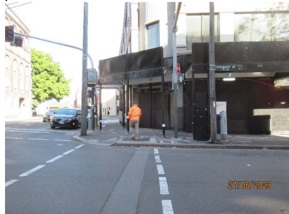
Figure 3.4 Hunter St West: B Class Hoarding Construction
