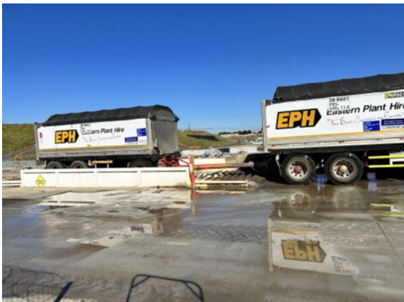
Figure 2.11: Clyde MSF Site – Stormwater Pit maintenance required on Unwin Street
