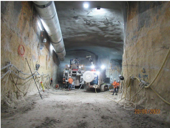
Figure 3.5 Tunnel decline: Ongoing excavation by road headers.
