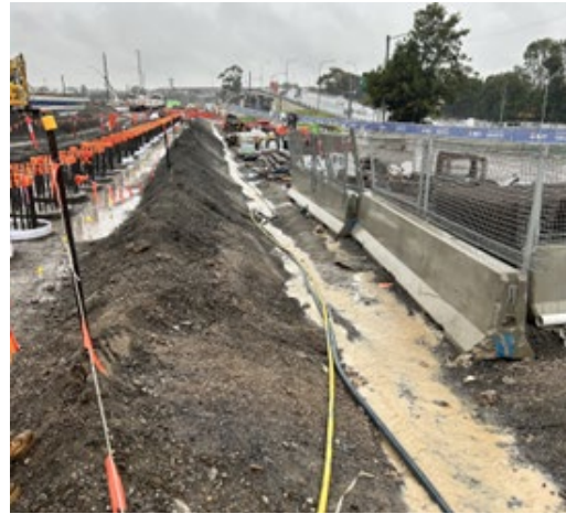
Figure 2.8: Clyde Dive site – Spoon drain down the centre of the site carry dirty water during rain
