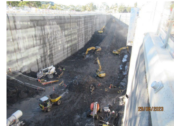
Figure 1.8 Excavation of the Station Box (SOP). Construction of nozzles in the western end.
