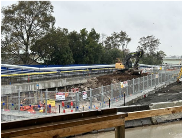
Figure 2.7: Clyde Dive site – Dive Structure excavation along the ATC boundary
