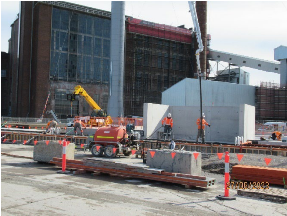
Figure 3.7 The Bays: Concrete works for the WTP
