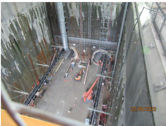
Figure 1 1 Both TBMs have left the Station Box (The Bays)
