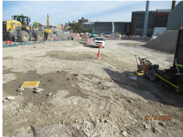
Figure 3.8 The Bays: General site establishment activities
