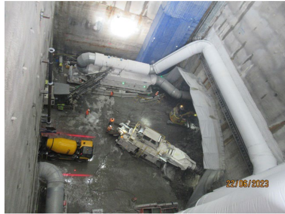
Figure 1.4 Cavern excavation works under the acoustic shed. (Five Dock)
