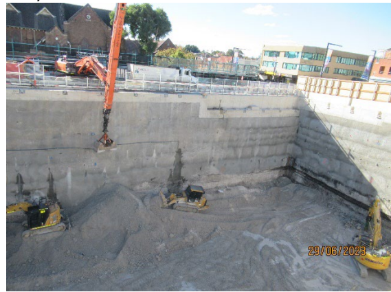
Figure 1.6 Ongoing excavation of the west shaft (Five Dock-west) utilising a surface miner as well as excavators with hammers.
