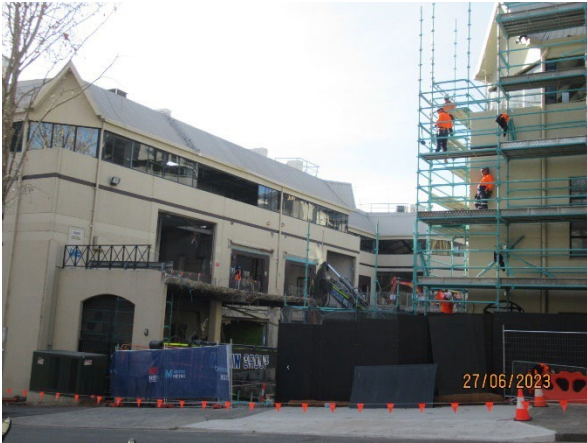
Figure 3.1 Pyrmont East: Commencement of hard demolition works from Edward Street
