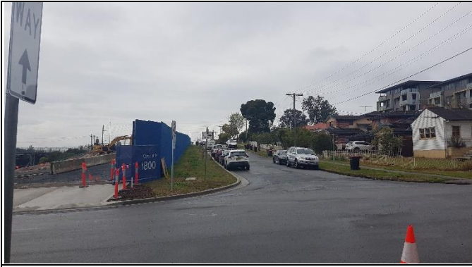
St Marys view east – Chesham St hoarding awaiting graphics.
