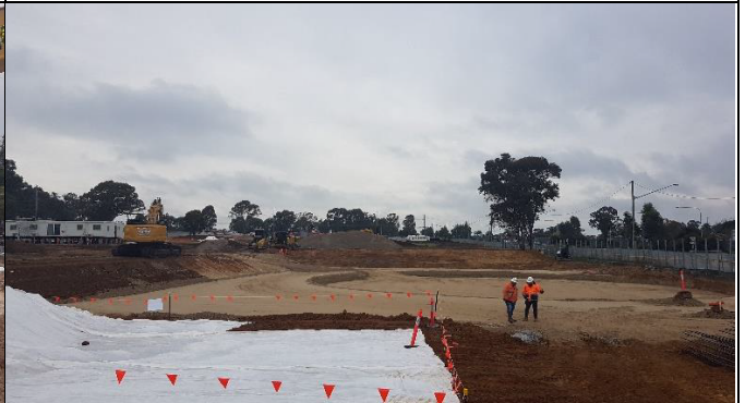
Claremont Meadows view south - Shaft pilling pad complete .
