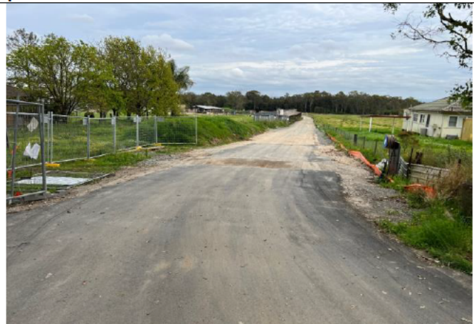
Power: Lawson Road compound handed back to the landowner
