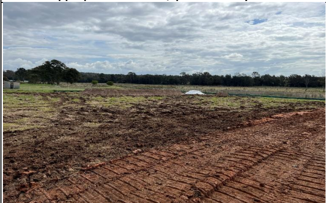
Bringelly Services Facility –.North west corner behind dam
