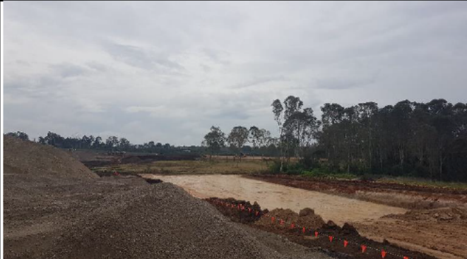
Orchard Hills view north: Excavation of tunnel portal access
