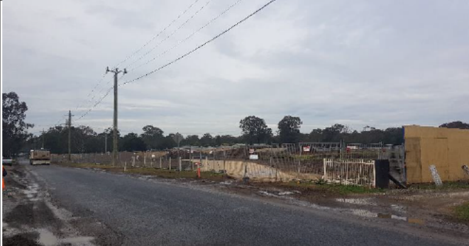
Orchard Hills – Lansdowne Rd diversion construction looking east from Kent Rd
