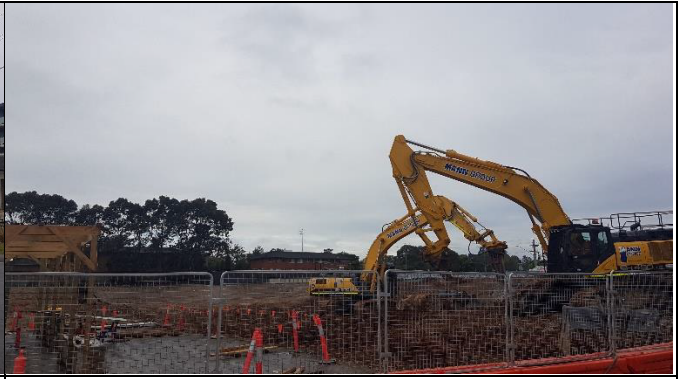
St Marys – Plaza demolition completed with concrete preparation for disposal offsite.
