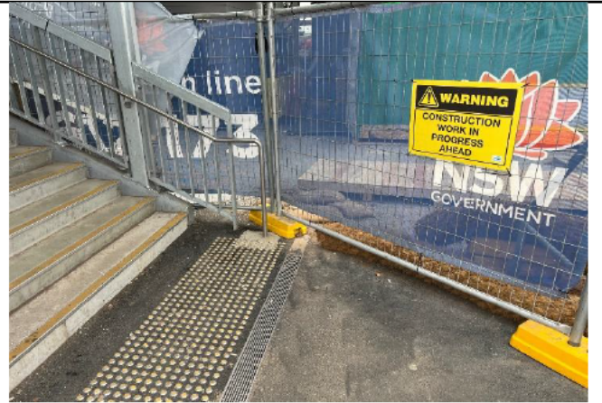
St Marys lift relocation– Erosion and sediment controls in place
