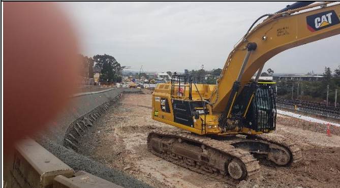
St Marys view west – Embankment shotcreting and soil nail installation underway
