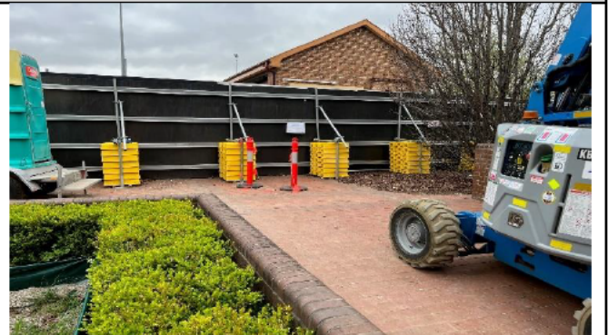
St Marys lift relocation – Hoarding west of (behind) goods shed
