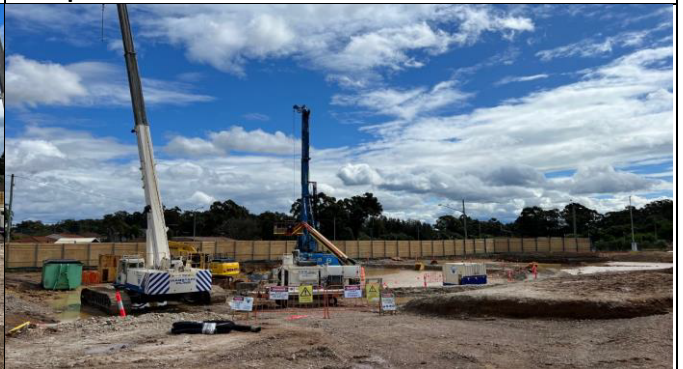
Claremont Meadows view southwest – shaft pilling establishment
