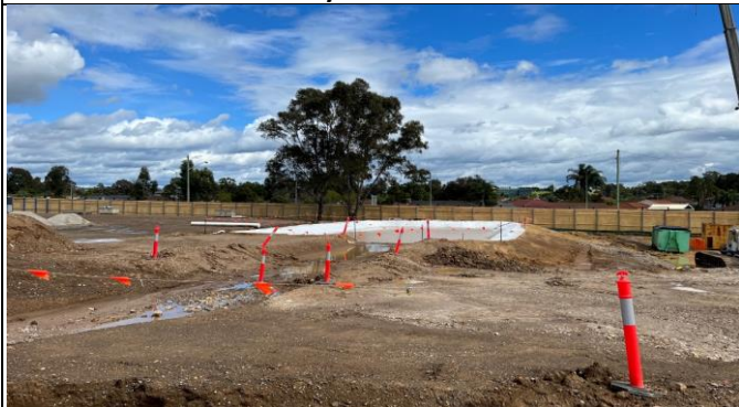
Claremont Meadows view west - inlet drains to be lined with an appropriate material / protective layer.
