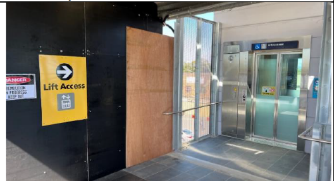
St Marys lift relocation – New lift shaft installed and operational
