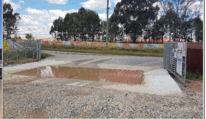
Claremont Meadows southern access - southern access includes wheel wash depression.
