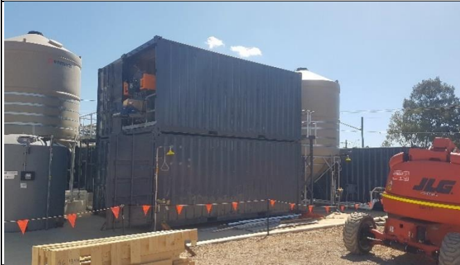
Claremont Meadows – Water Treatment Plant southern elevation
