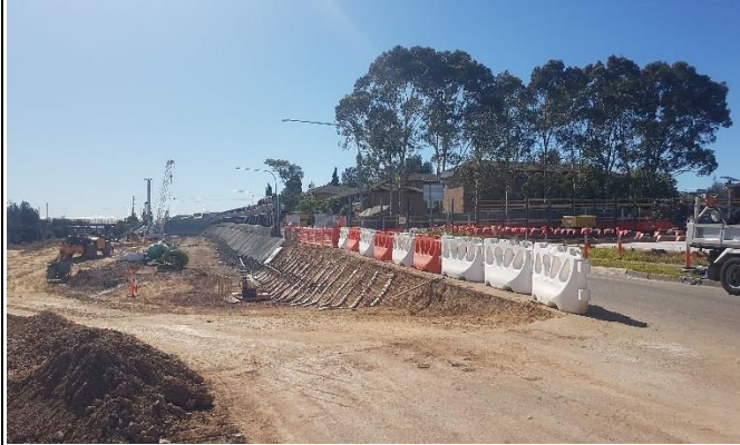
St Marys - View east from Station street at former Station Plaza.
