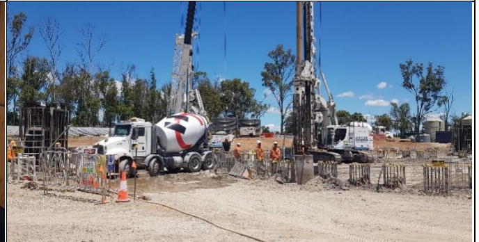
Bringelly Services Facility – View south west of shaft pilling
