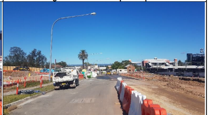
St Marys – Looking west along Station St.
