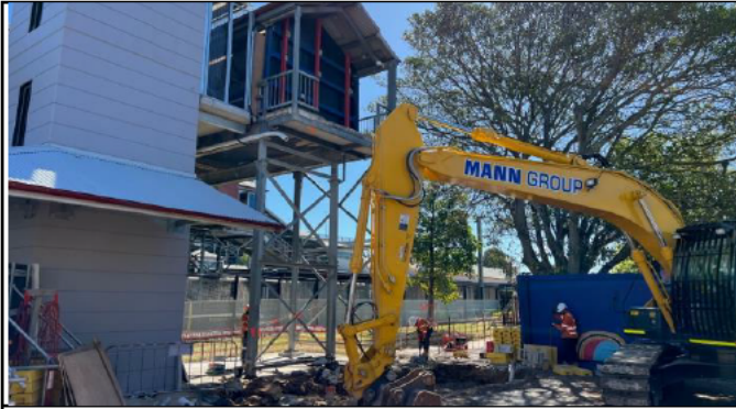
St Marys lift relocation – The old lift shaft has been demolished
