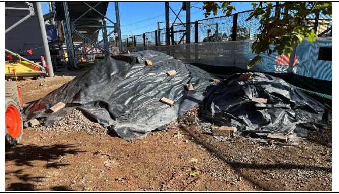
St Marys lift relocation rail side– Site won spoil
