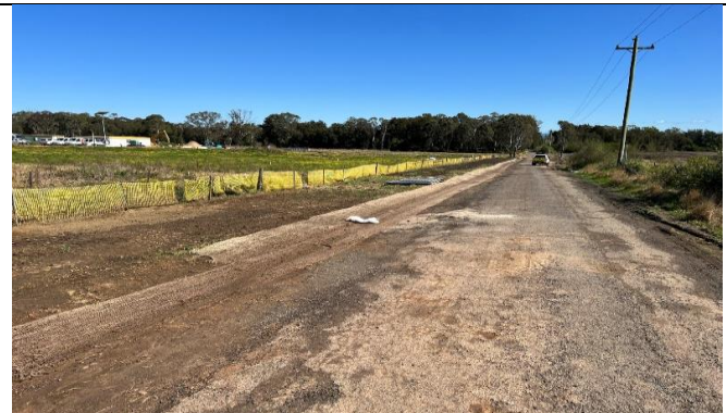
Power: Works on Pitt Street complete and reinstated
