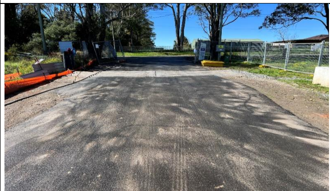
Power: wheel wash in operation at the Lawson Road compound exit
