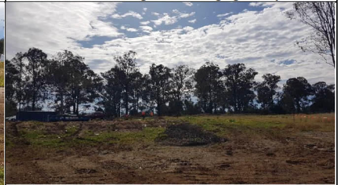
Orchard hills view north – Demolition of Kent Rd residences at completion
