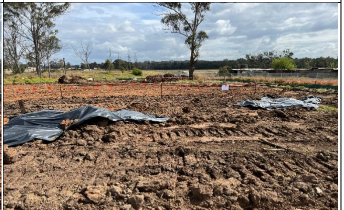
Bringelly Services Facility – View West to central dam after clearing.
