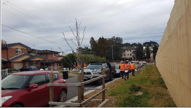
St Marys – Chesham St hoarding near completion.
