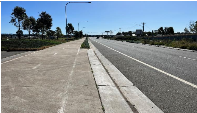
Power: Ares works along Gipps/Kent Road reinstated
