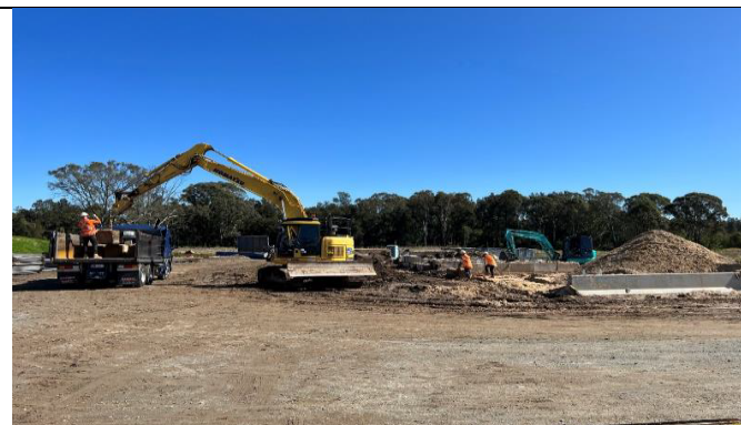
Power: Lawson Road compound is being demobilised
