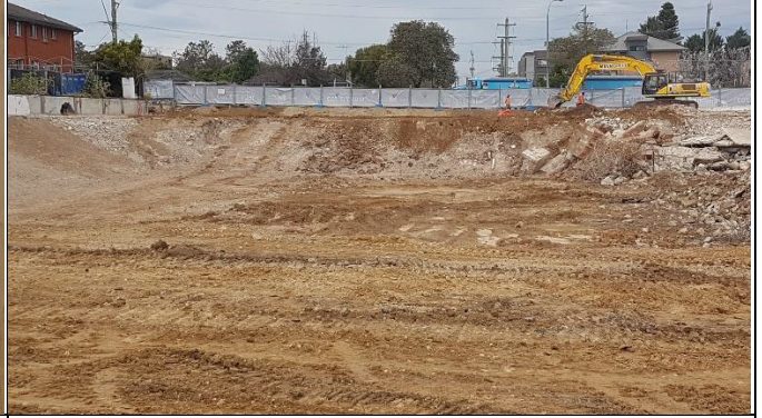
St Marys – Plaza demolition near completion.
