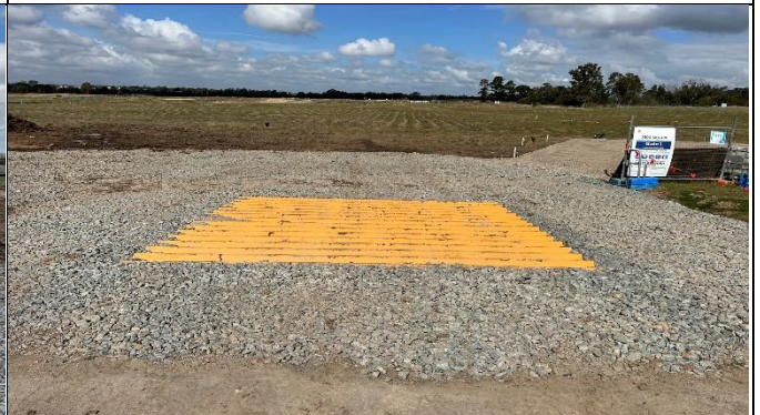
Aerotropolis – View south form site entry.
