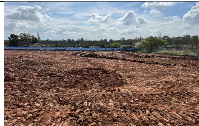
Bringelly Services Facility – View site leveling along Derwent Rd.
