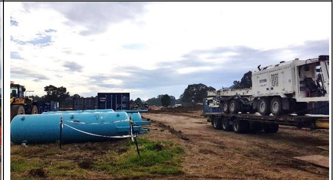
Claremont Meadows – View south at access Road excavation.
