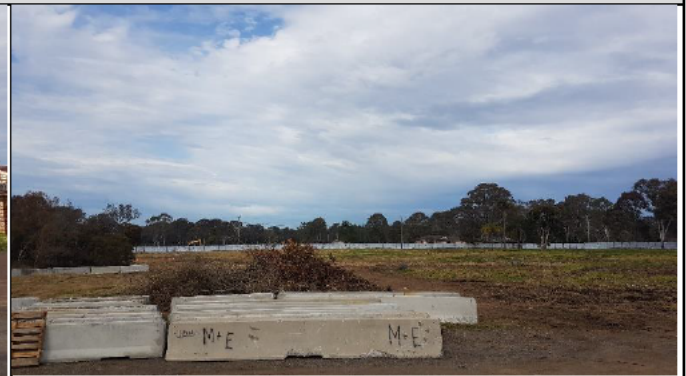
Orchard Hills view to Lansdowne Rd - Clearing with PCT areas and Moderate/High risk AEC segregated by barriers
