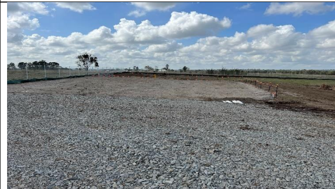
Aerotropolis – View West form site entry to carpark construction.
