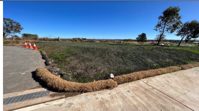
Power: Restoration works along Kent Road complete
