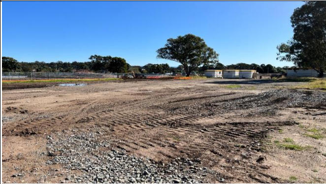
Power: the Gipps Street compound is being demobilised
