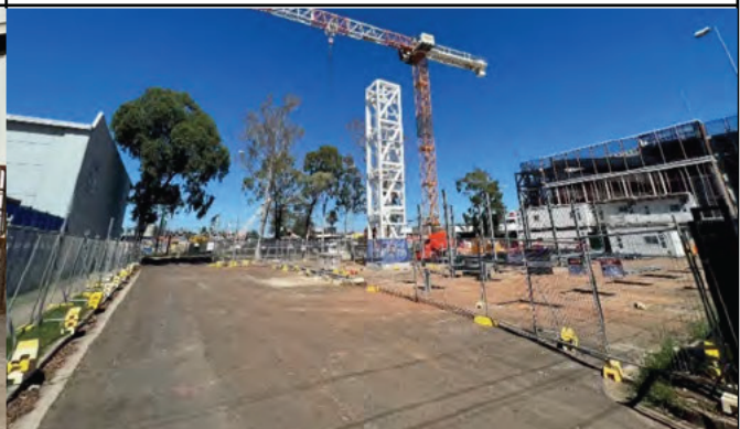
The tower crane and lift shaft were installed
