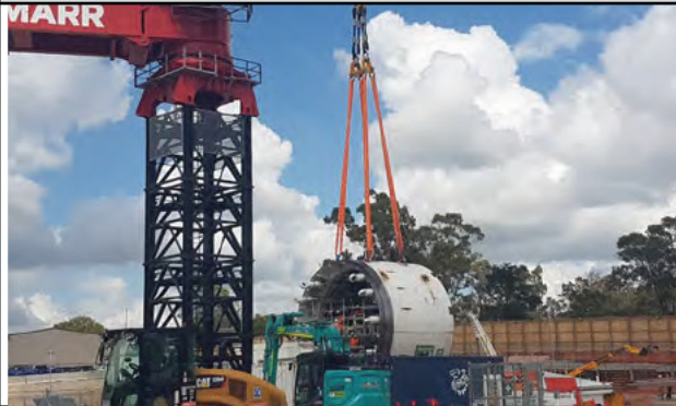
Orchard Hills Station box North – TBM segments being lifted into place
