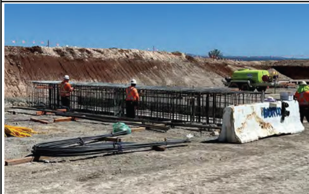
Elizabeth Drive – Steel fixing is occurring ahead of the concrete pours
