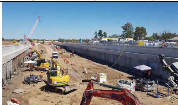
St Marys: Eastern station box excavation, shotcreting and anchor installation
