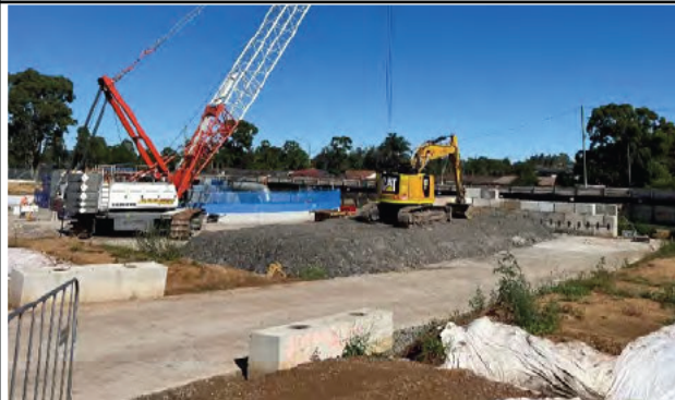
Claremont Meadows – Shale from the excavation is being stockpiled and sent to the adjacent development
