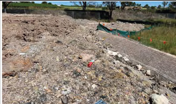
Claremont Meadows – Shale from the excavation is being stockpiled and sent to the adjacent development
