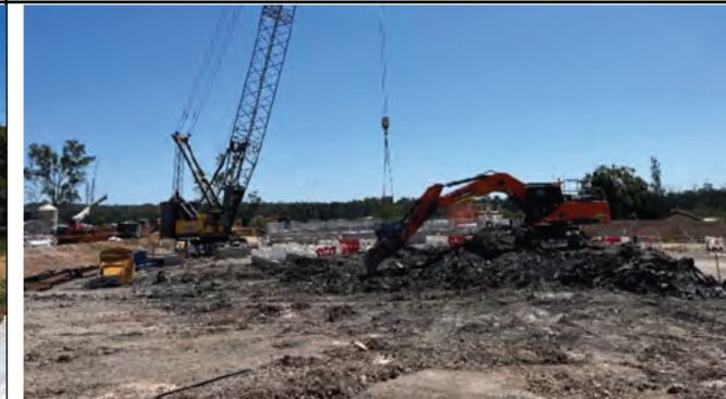
Bringelly Services Facility – Spoil loadout continues
