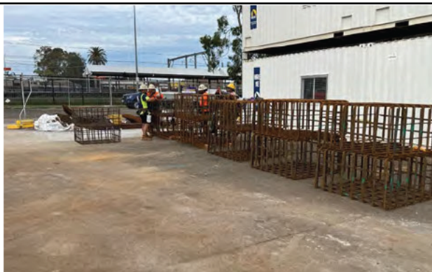
Reinforcing has been made off site and calculated to minimise any wastage during construction
