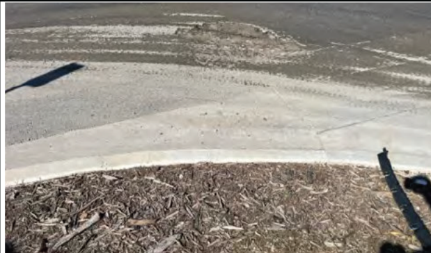
St Marys - A pot hole has opened up at the exit point from Gidley St and is causing mud tracking.
