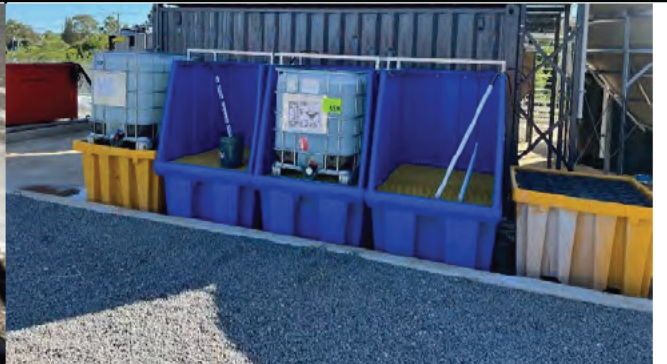
Claremont Meadows – The water treatment plant is in its commissioning phase
