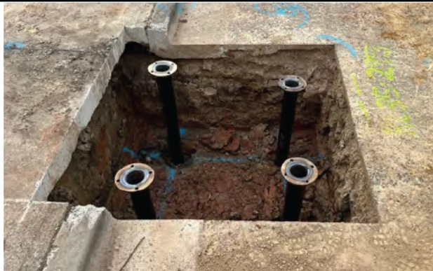
Screw piles installed in the excavations on site
