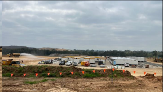
Elizabeth Drive - The site compound continues to be established
