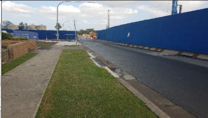
St Marys – Looking west along Station St.
