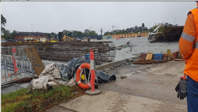
St Marys view south east to Station Plaza –laydown slab complete.
