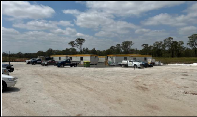
Patons Lane – The site compound is complete
