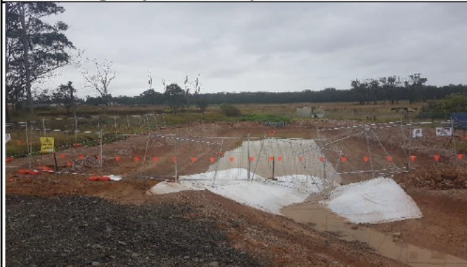
Bringelly Services Facility view north west–. Sed. Basin in operation
