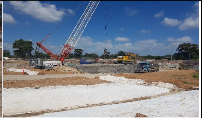
Claremont Meadows view northwest – Shaft excavation spoil.
