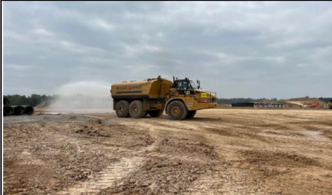
Elizabeth Drive - Moxy watercarts were in operation during the inspection
