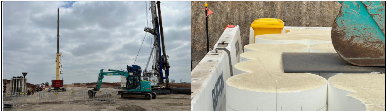
Elizabeth Drive - Piling has commenced at the northern piling pad
