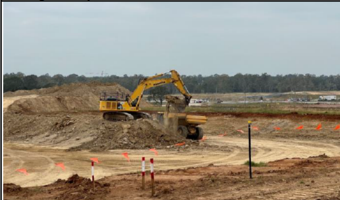
Elizabeth Drive – Earthworks continue to the south of the site compound
