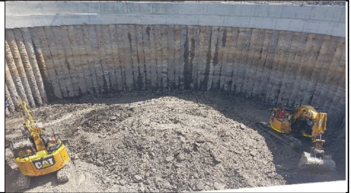
Claremont Meadows view west – Shaft bulk excavation
