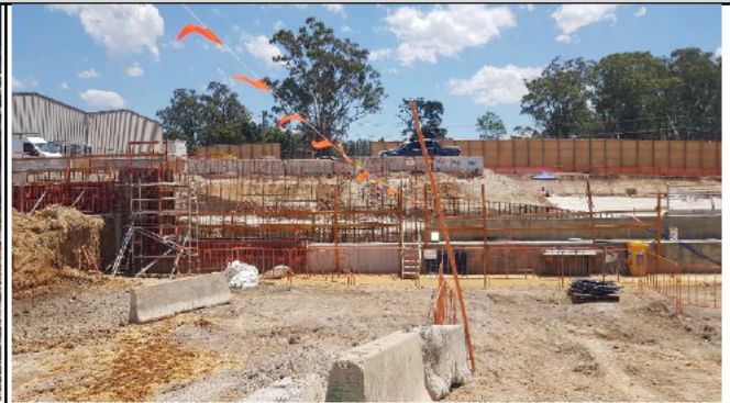
Orchard Hills central, view west – Capping Beam construction
