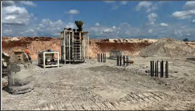
Elizabeth Drive – Piling commenced on the northern end of the project
