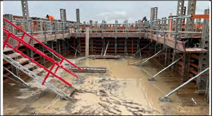
Elizabeth Drive –formwork installed for the upcoming concrete pours
