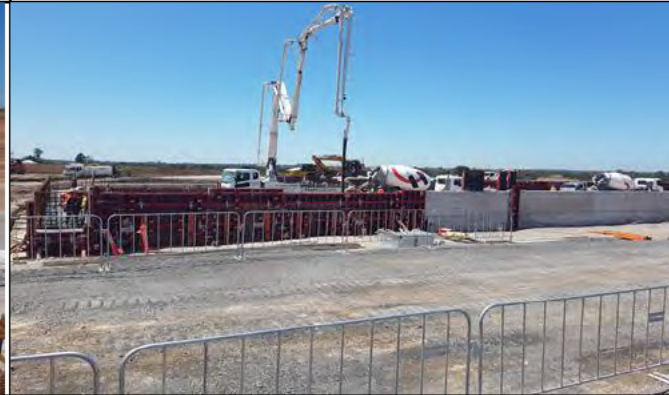
Aerotropolis : Station box north capping beam and upstand FRP.
