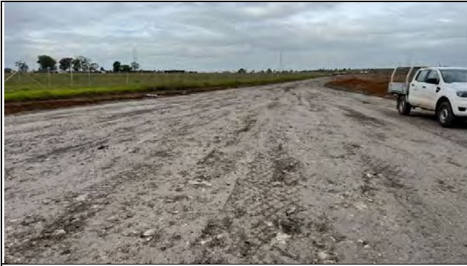
SMF - Sandstone has been placed along the access tracks to create all weather tracks
