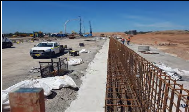
Aerotropolis : Station box south piling, blinding and western capping Beam FRP.
