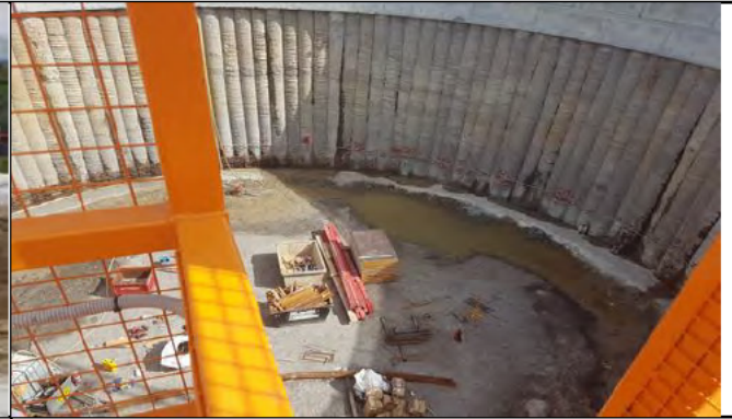
Claremont Meadows– Shaft excavation ring beam FRP
