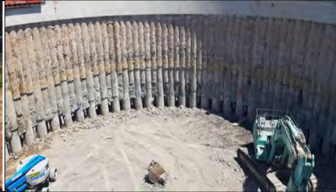
Bringelly Services Facility – Services shaft bulk excavation.
