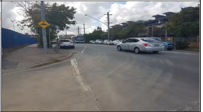
St Marys looking southeast from Gidley St: Negligible tracking noted at exit to Philip St
