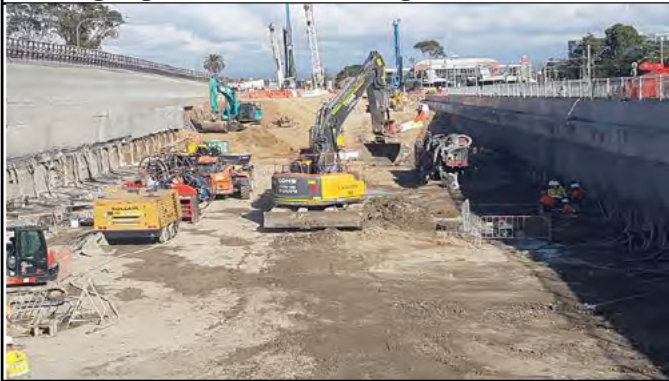
St Marys: Eastern station box excavation, shotcreting and anchor installation
