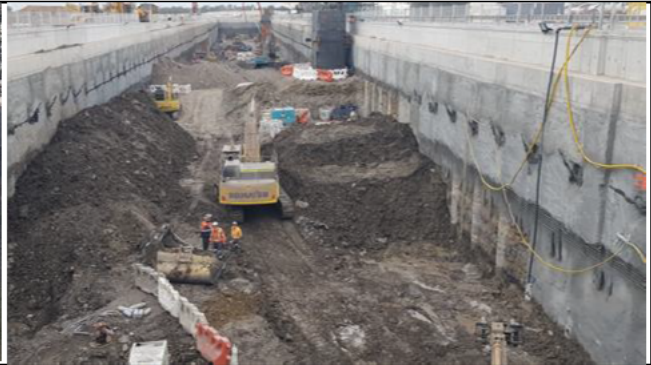
Aerotropolis station box: View south
