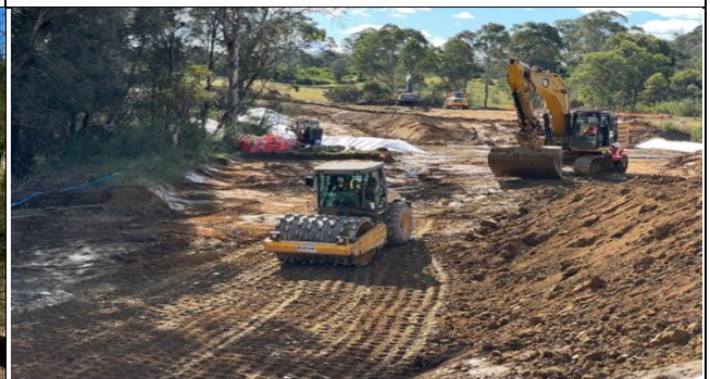
SMF - Works on the creek crossings at Blaxland Creek
