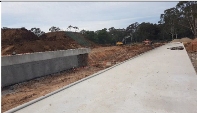
Orchard Hills: Dive excavation south of Lansdowne Rd.
