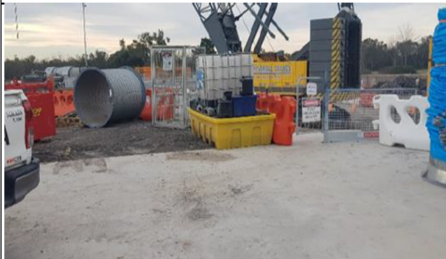
Bringelly Services Facility – Laydown area and maintenance compound very well managed.
