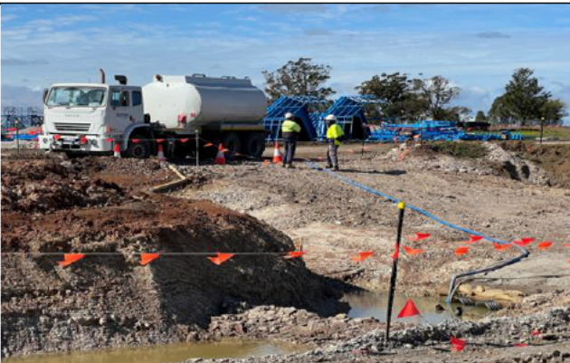
Luddenham station - Water collected in structures used for dust suppression
