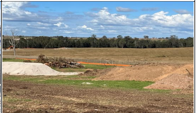
Luddenham South - Remaining felled trees to be mulched or disposed of.
