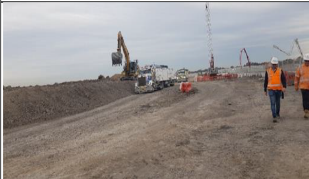
Aerotropolis view to southeast: excavated spoil haulage to M12 project
