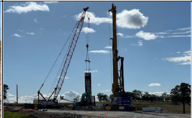
Luddenham south - Piling has commenced
