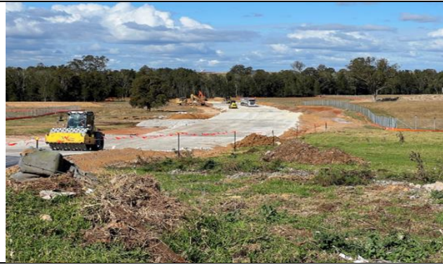
Luddenham south - Sandstone is being imported for use along alignment.
