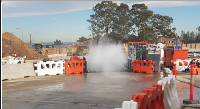
St Marys- Truck wash operating.
