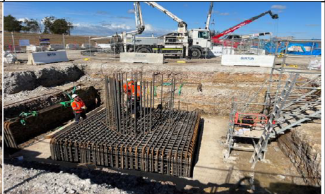
Luddenham station - Steel fixing for the base and column structures
