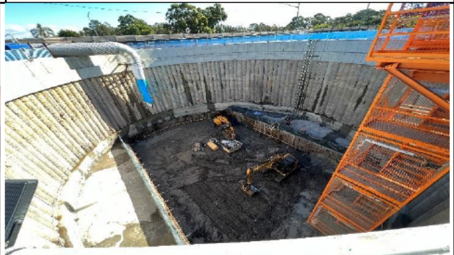
Claremont Meadows Services Facility: Services shaft excavation
