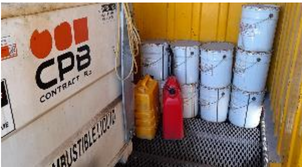
Plate 9 - Fuel jerry can store in bunded container post audit inspection
