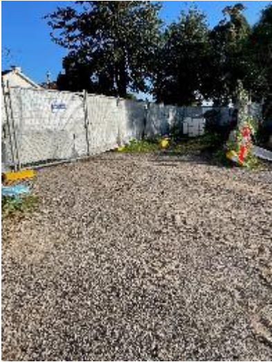
Plate 53 – Bounday fencing and hardstand work area
