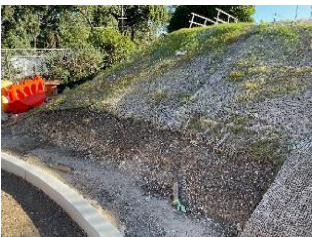
Plate 41 – Sediment control for access road to be sealed
