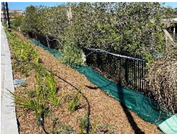
Plate 21 – Landscaped area with boundary sediment fence and control
