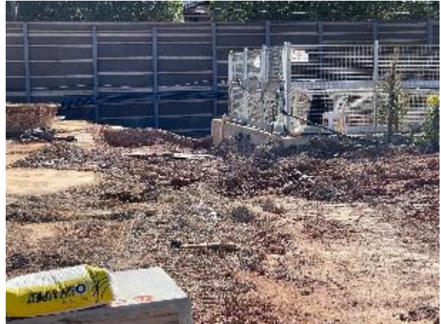
Plate 6 – Lower site boundary fence
