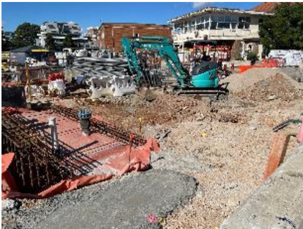
Plate 3 – Excavation and plumbing works
