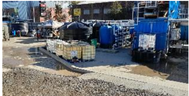
Plate 8 - Chemical containers placed in designated bunded area at Marrickville Dive
