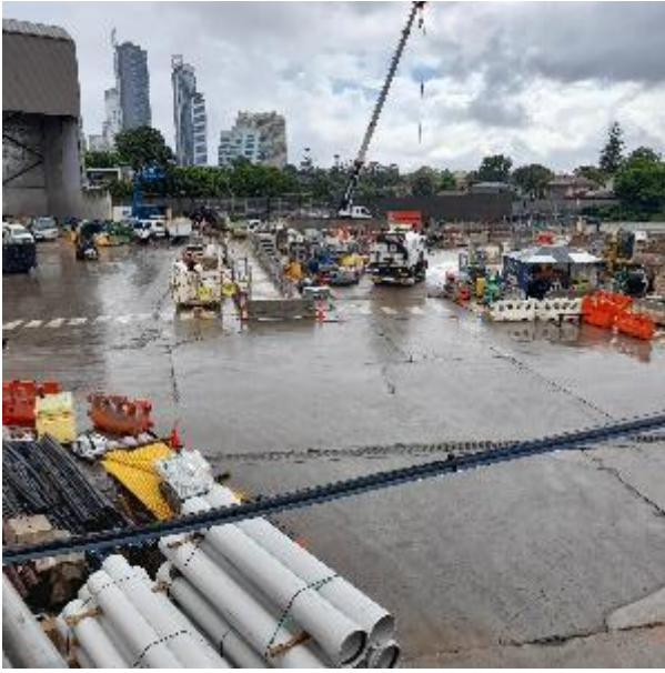
Plate 5 – Example of water spraying for dust suppression at Chatswood Dive
