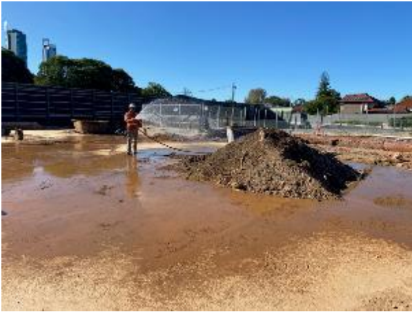
Plate 1 – Dust suppression of stockpiles post audit inspection at Chatswood Dive
