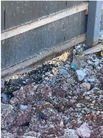
Plate 7 – Gaps below lower boundary fence with no sediment control – potential for sediment to erode / track offsite onto road during heavy rain
