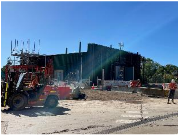
Plate 1 – Dive site service building – civil and M&E works and concrete breaking
