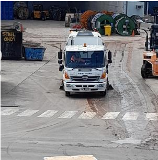
Plate 3 – Example use of sweeper and water cart for dust suppression at Chatswood Dive
