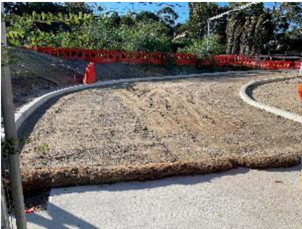
Plate 41 – Sediment control for access road to be sealed
