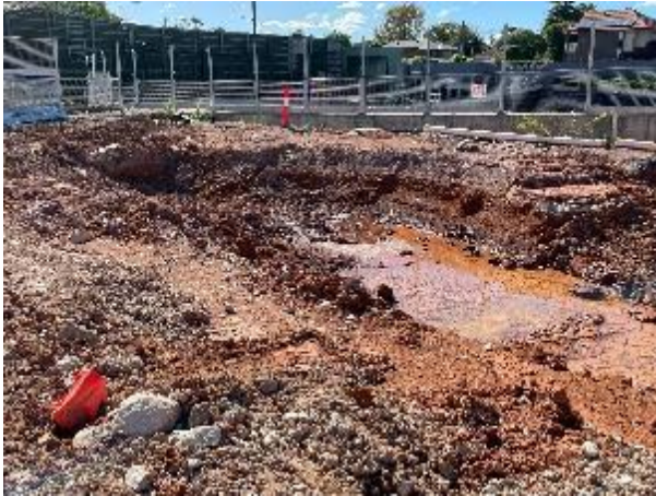
Plate 5 – Temporary detention basin
