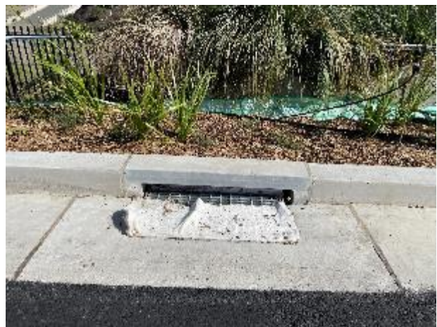
Plate 22 – Freshly sealed access road with curb and gutter drainage
