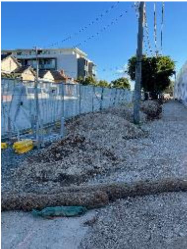
Plate 55 – Erosion control public domain works
