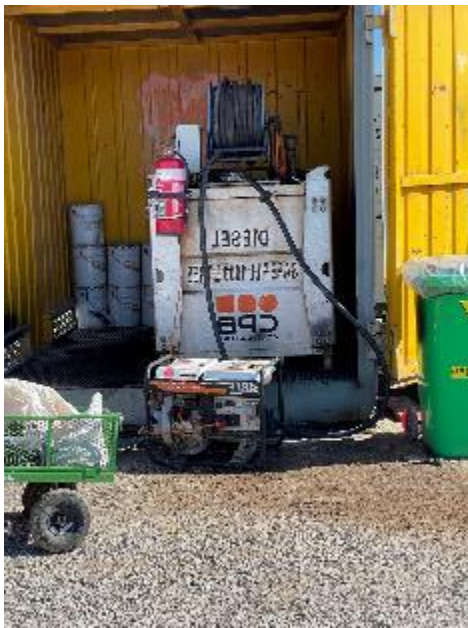
Plate 38 – fuel storage container and filling station with signs of spills outside the container
