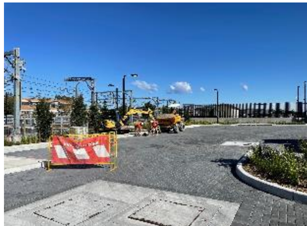
Plate 22 – Freshly sealed access road with curb and gutter drainage
