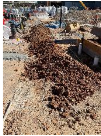
Plate 4 – Excavated material for re-use on-site or offset disposal
