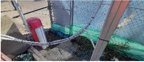
Plate 11 – Sediment fence repaired at end of Sydney Steel Road adjacent Gate S2 post audit inspection
