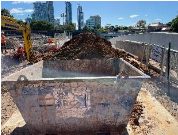
Plate 14 – Waste bins and earth stockpiles
