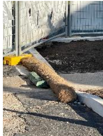
Plate 52 – Erosion control in public domain works area
