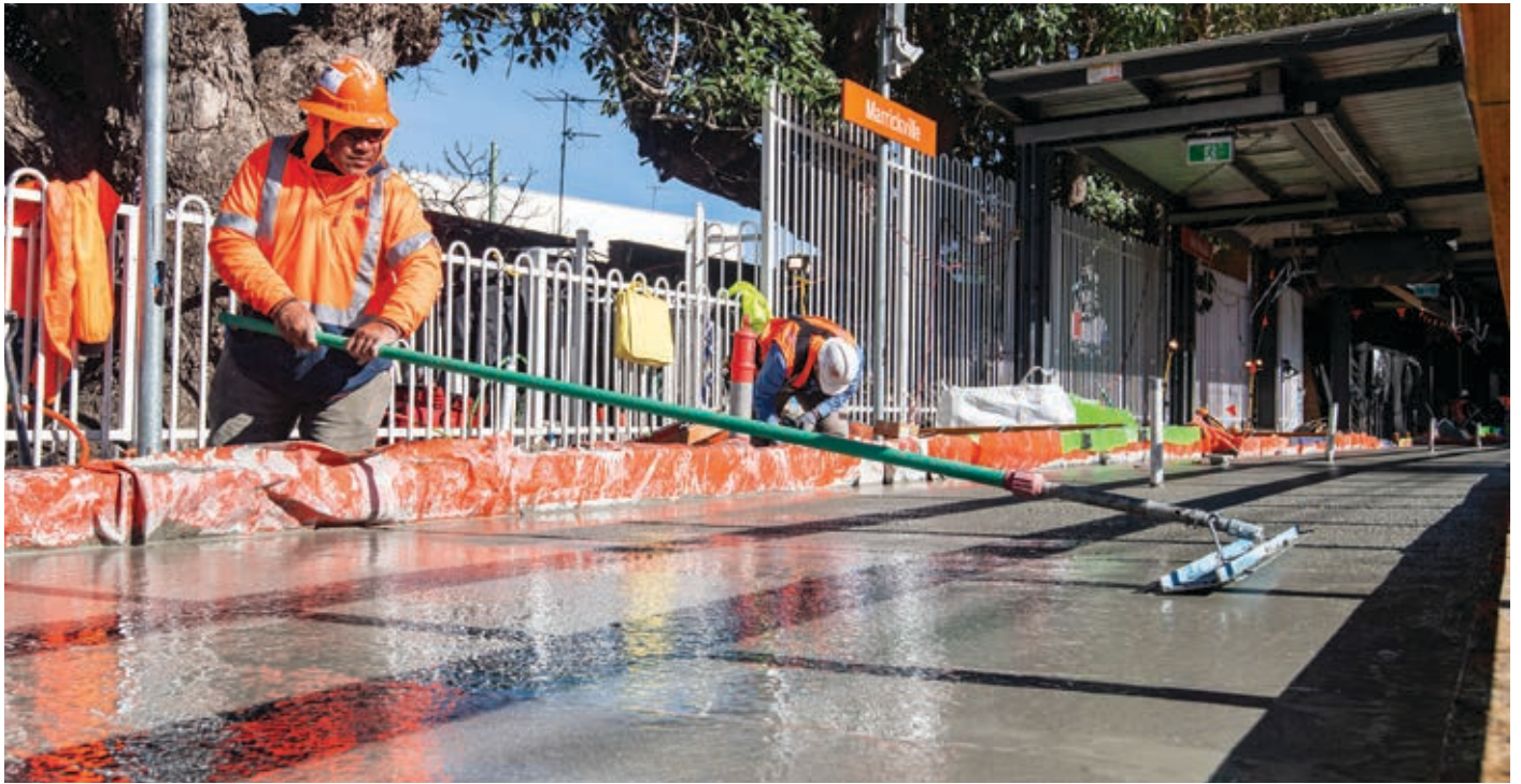
Concrete being cured for new platforms at Marrickville Station.
