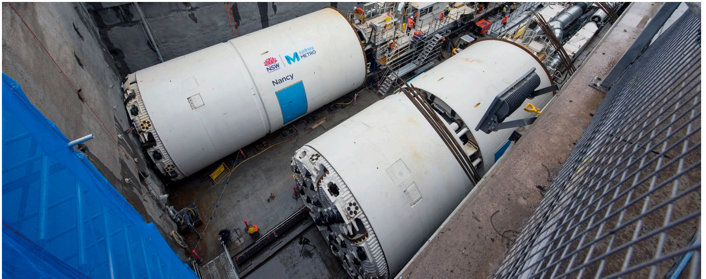
A tunnel boring machine at Marrickville.
