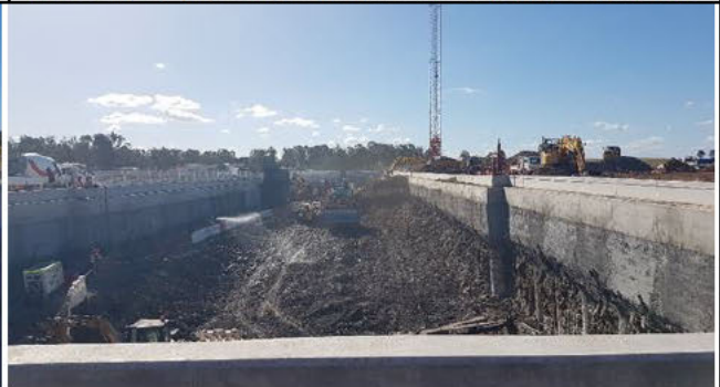
Aerotropolis station box: View north
