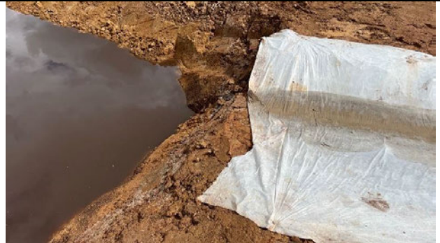
Patons Lane - The inlet to the recently dug sediment basin requires geofabric to extend down to prevent scour of the inlet
