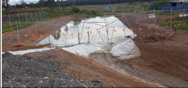
Bringelly Services Facility – shaft water was being discharged to the sediment basin
