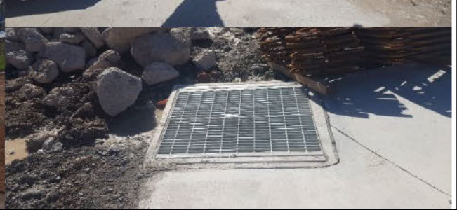
Bringelly Services Facility - Concrete washout and waste near pit connected to swale, and sed. basin
