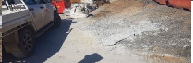
St Marys - Observed Sediment laden water, from wheels being hosed down, discharging to pits
