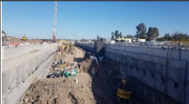
Aerotropolis station box: View south
