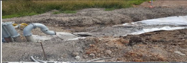
St Marys- Wheels hosed as truck wash at exit out of action - being replaced by new automatic wash.
