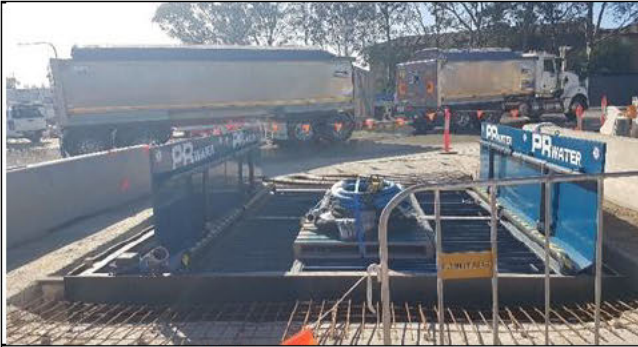
St Marys- Wheels hosed as truck wash at exit out of action - being replaced by new automatic wash.
