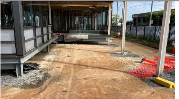
The main entrance point of the SPO is progressing
