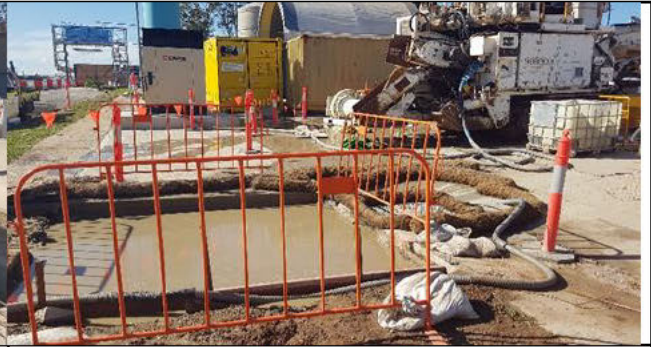
St Marys - Observed Sediment laden water, from wheels being hosed down, discharging to pits
