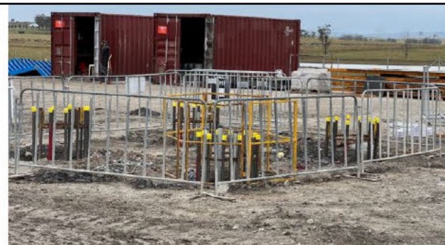
Luddenham station - Piling has commenced at the Luddenham station site
