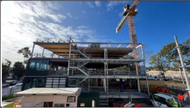
The superstructure is complete and façade elements are being installed
