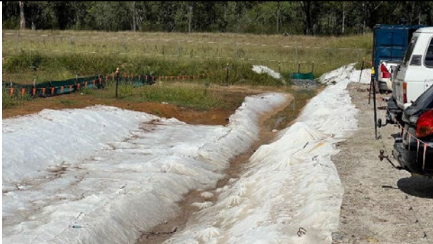
Patons Lane - ERSED controls around the perimeter of the compound have been effective in dealing with the recent rain
