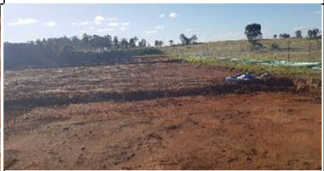
Aerotropolis : PFAs contaminated area has been broken up with earth berms to limit erosion
