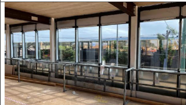
The façade is placed internally and provides a sound barrier
