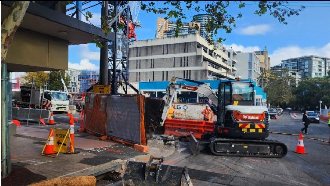
Clark Street utility works
