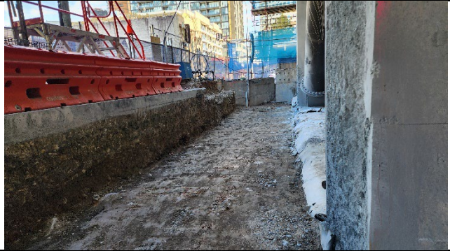
Site A Capping beam removal
