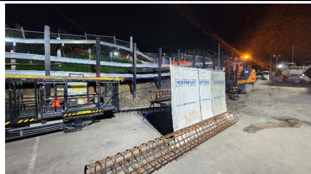
Canterbury Installation of noise blankets from piling cage cutting area
