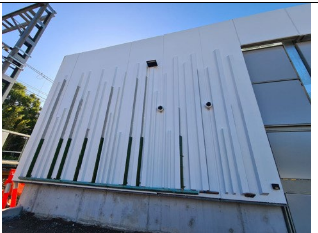
Canterbury TSS: Tiling works commenced (TSS façade)
