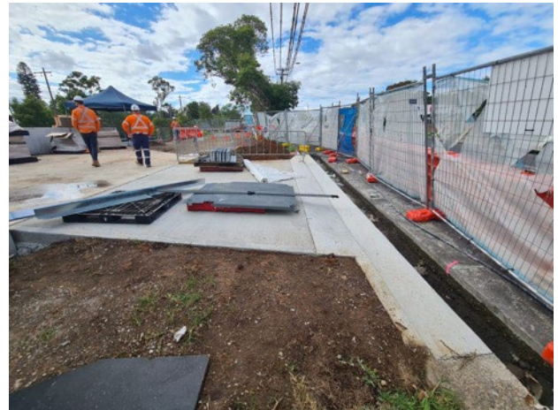
Lakemba TSS: Driveway poured
