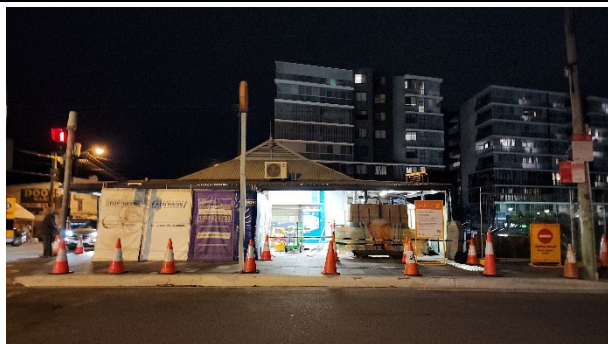
Canterbury Plaza – installation of noise blankets and pedestrian access was maintained
