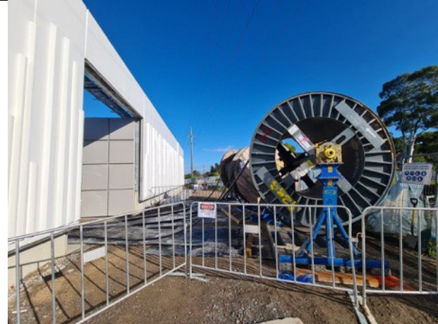
Dulwich Hill TSS: Cable pulling (from TSS basement to GST installed)
