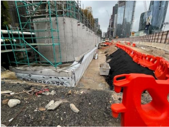
Ventilation pod installation ongoing; services mostly backfilled
