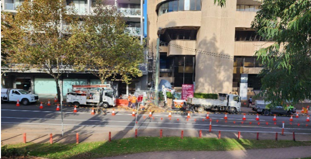
Clark St – Utility and public domain works
