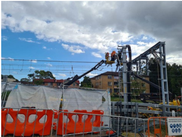
Campsie TSS: Dressing cables on OHW structure (possession related works)
