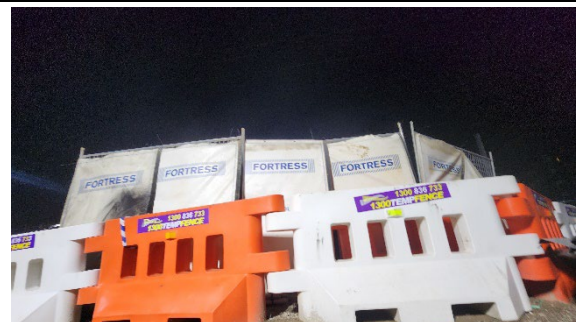
Canterbury Cess – noise mats installed adjacent to excavation works
