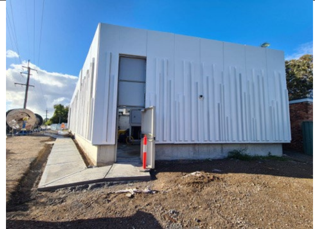
Dulwich Hill TSS: Anti-graffiti painting and footpath works around building completed
