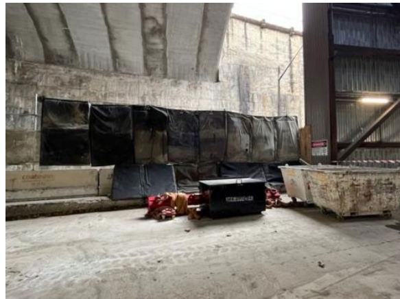
Material strip-out from the northern shaft and installation of noise blankets as per the CNVIS
