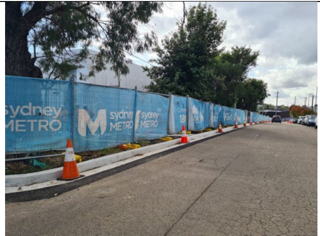
Campsie TSS: Streetscaping works – Kerb and Gutter works along (Lilian St)
