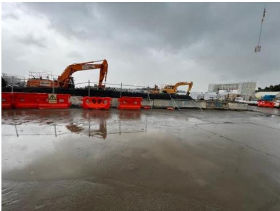
The site access and hardstand were clean and dust was controlled by light rain, and water cart and sweeper during dry weather
