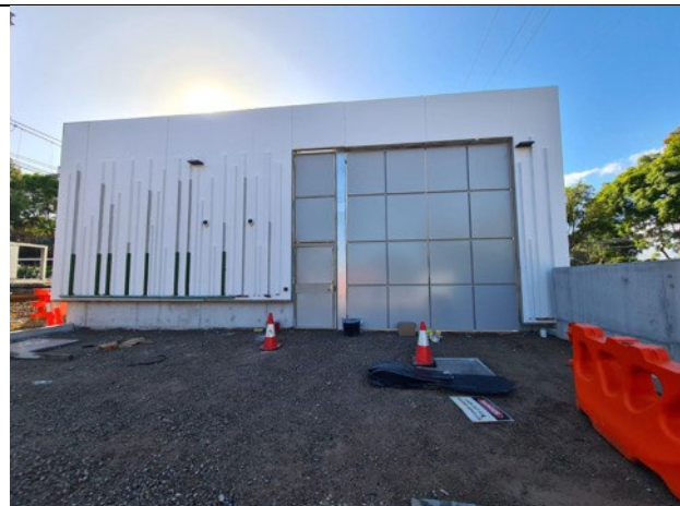
Canterbury TSS: Tiling works commenced (TSS façade)
