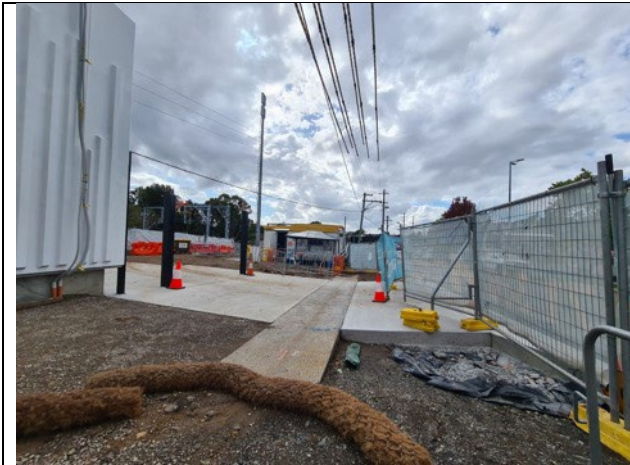
Campsie TSS: Streetscaping works – Driveway poured
