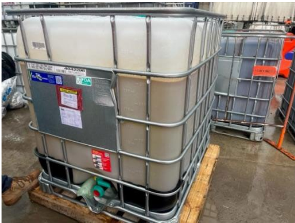
IBCs were unlabelled and adequate storage arrangements could not be verified
