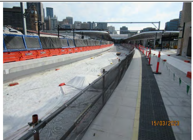
Platform 14: Ongoing tiling detail and fit out of the canopy.
