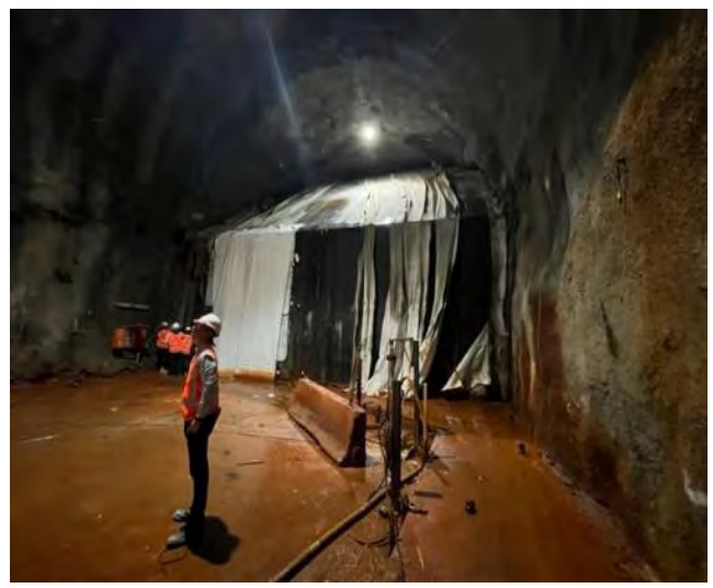
Ongoing installation of the ventilation pods in Zone 4
