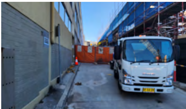
Clarke Lane South - Clarke Lane South and Site B scaffold
