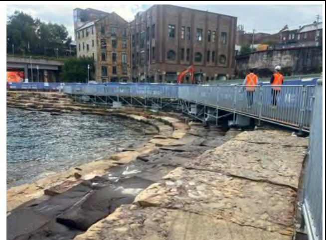
Pedestrian diversion scaffold bridge
