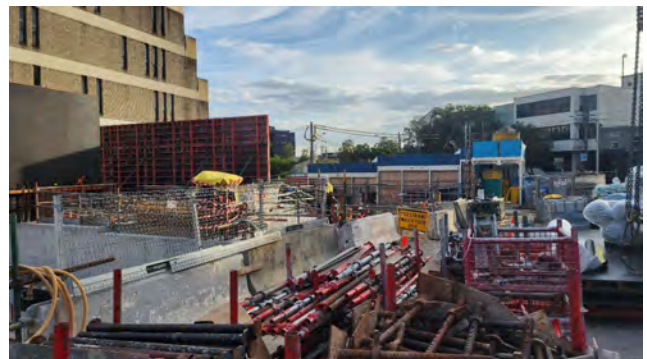
Site C: view northeast
