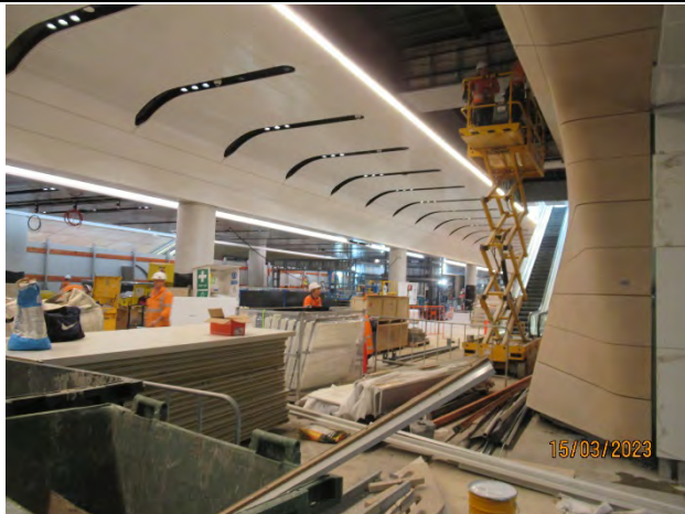
North/South Concourse: Ongoing fit out
