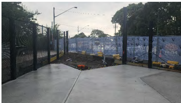
Marrickville MSB Driveway and fencing
