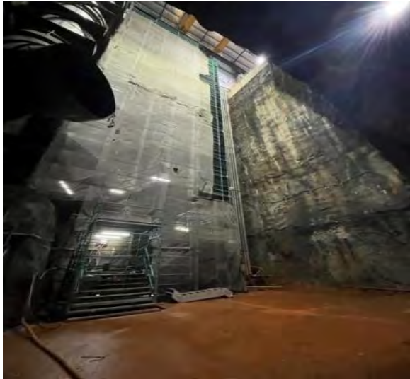
Northern shaft handed over to BESIX Watpac for backfill
