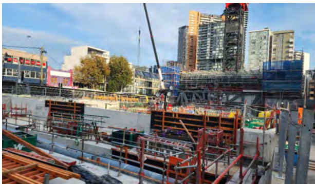
Site A view north: L2 FRP with Hume St FRP foreground
