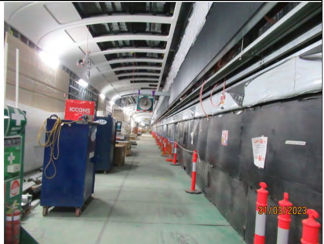
Martin Place - Platforms: Ongoing fit out works.
