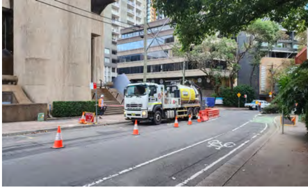
Clark St – Utility and public domain works
