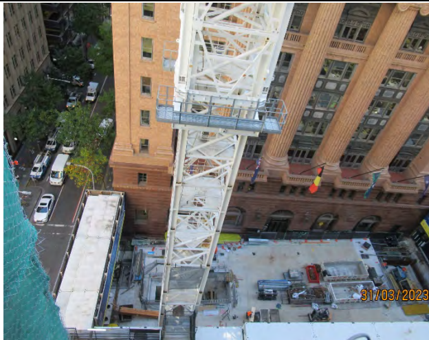
Martin Place: Concrete slab in place. Use of area for laydown.
