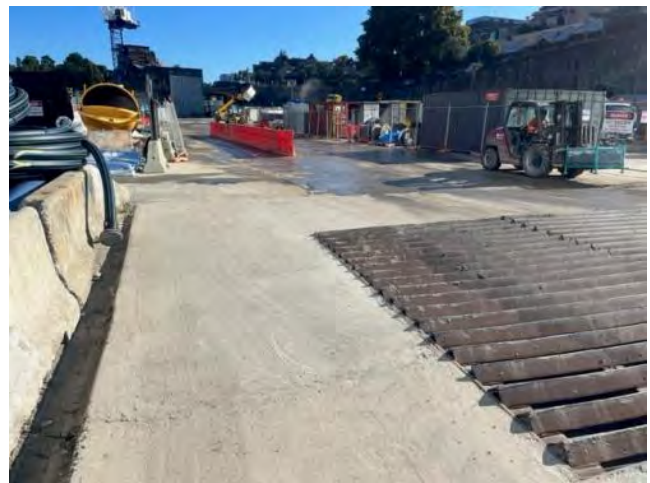
Well maintained site access
