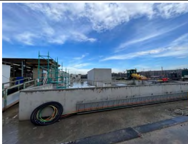
New bund for WTP
