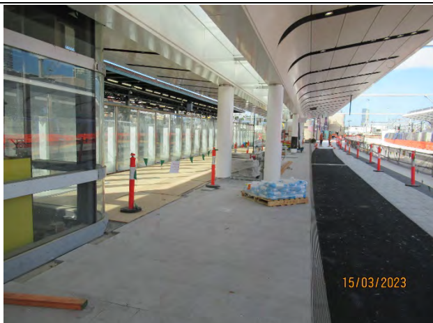
Platform 14: Ongoing fit out of canopy and other areas
