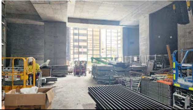
Pitt St South (PSS): Level 4 Preparation for louvre install
