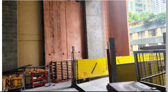
PSS: Level 5 podium/Level 6 façade walls adjacent to Princeton Apartments were sealed
