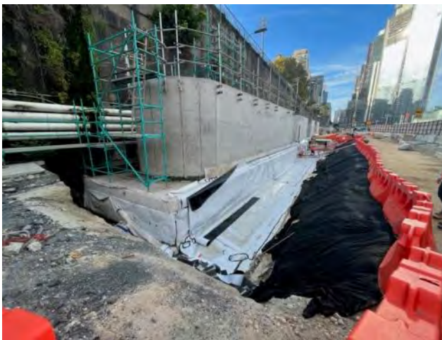
Construction of ventilation pods ongoing
