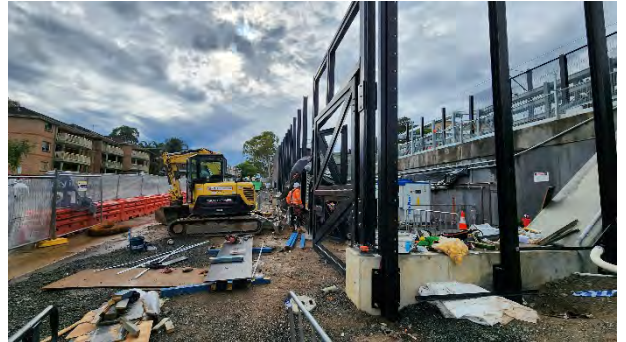
Lakemba Fence installation work
