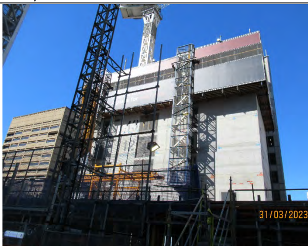
Martin Place South: Jump form use ongoing.
