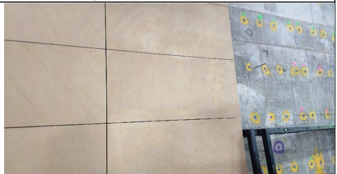
South Cavern – installation of reinforced glass panels
