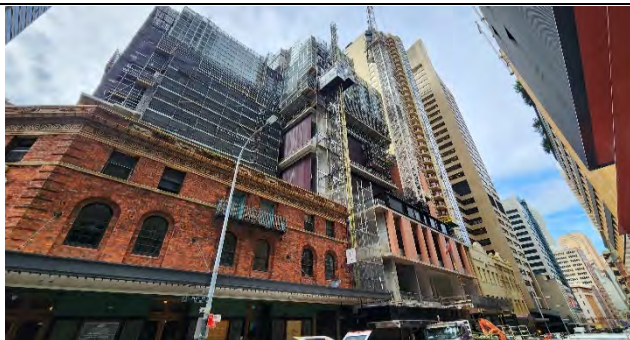
PSS view from Pitt St / Bathurst St
