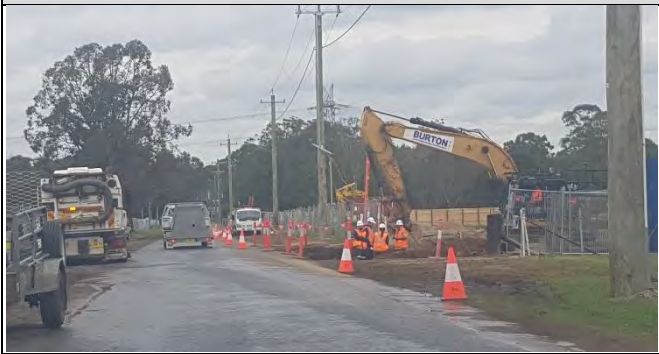
Orchard Hills – Lansdowne Rd diversion construction looking east from Kent Rd
