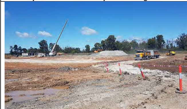
Aerotropolis : View north east to pilling pad and compound construction beyond.
