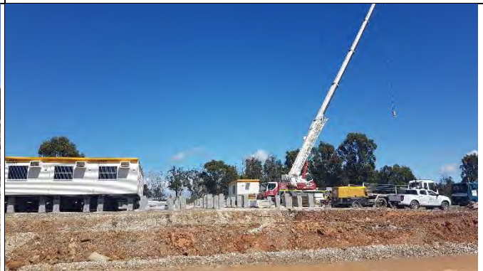
Aerotropolis : View east from pilling pad construction of site accommodation/compound.
