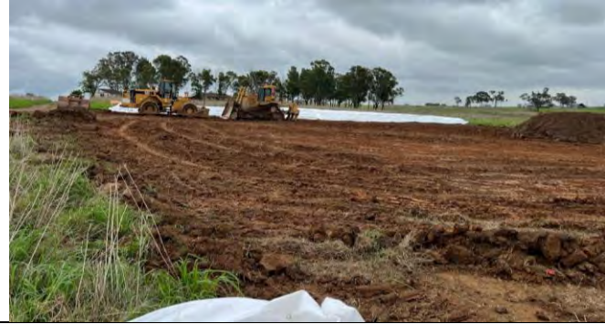
Elizabeth Drive - Topsoil stripping continues at the Elizabeth Drive site
