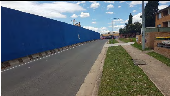
St Marys Station St view east: – Hoarding along Station St.
