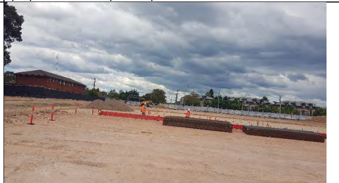
St Marys – Station Plaza earthworks completed.
