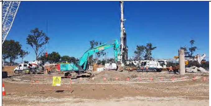
Bringelly Services Facility – View west of shaft pilling
