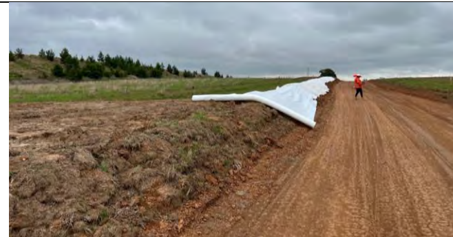
Patons Lane - Geofabric was being installed over the perimeter bunds
