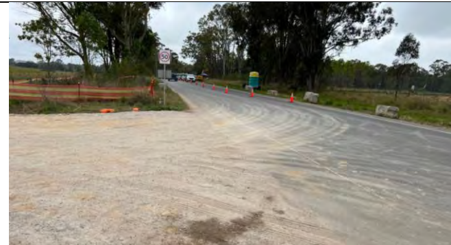
Patons Lane – The exit point had some dirt tracked onto the public road
