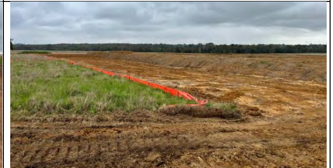
SMF - The SMF area is progressing well with perimeter controls installed
