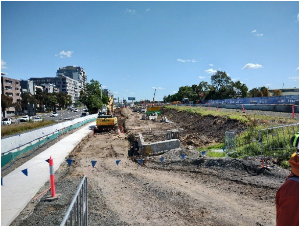
Figure 5-6: Clyde Dive earth works
