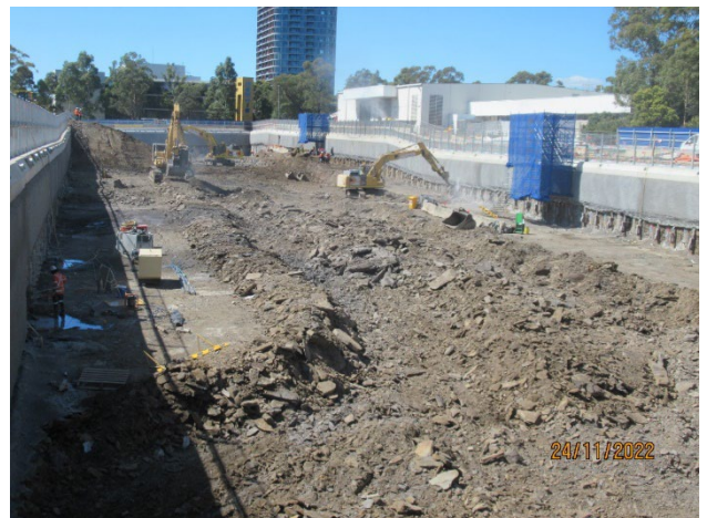
Figure 2-6 Ongoing excavation of the station box (SOP)
