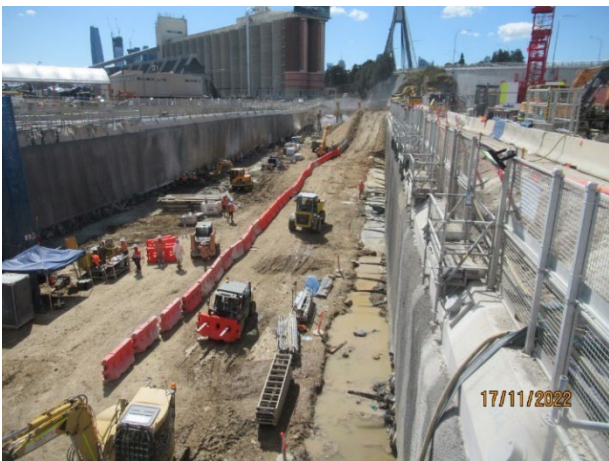
Figure 2-2 Ongoing excavation of the station box (The Bays)
