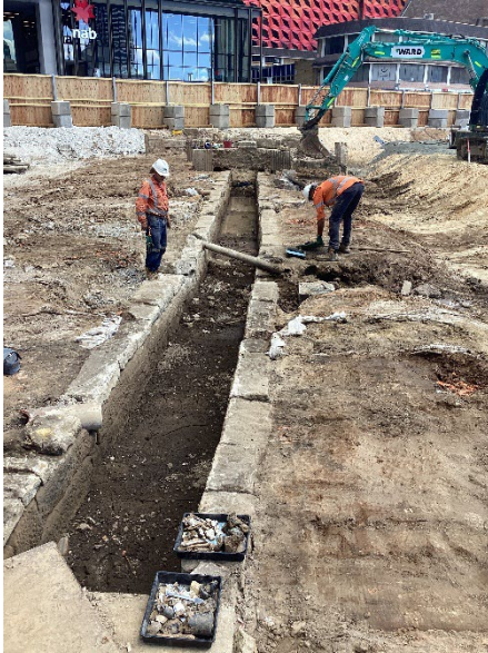
Figure 5-1: Convict Drain at Parramatta
