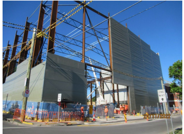
Figure 2-5 Ongoing construction of the acoustic shed (Five Dock-east)
