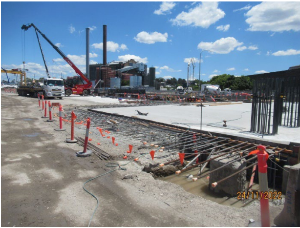
Figure 2-1 Concrete works for the Spoil shed foundations (The Bays)
