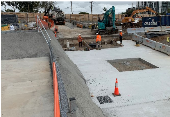
Figure 5-8: Westmead haul road construction
