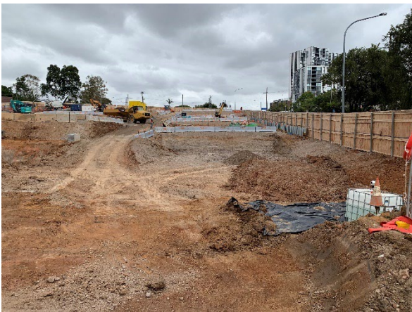
Figure 5-7: Westmead piling platform construction
