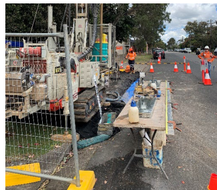
Figure 5-12: Geotechnical drilling outside EIS construction boundary
