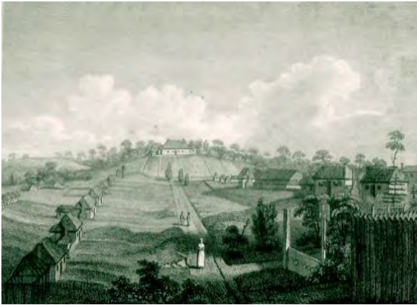
Figure 4.3 George Street, showing convict huts leading towards Government House (1798).
