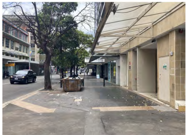
Photo 6.6 Approximate location of GALC-MW34 looking south along Marsden Street. Area of recent trenching indicated by strip of asphalt within the brick footpath.
