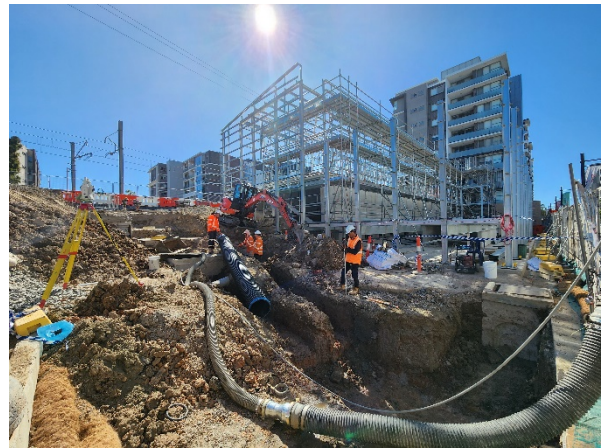
Canterbury MSB drainage installation
