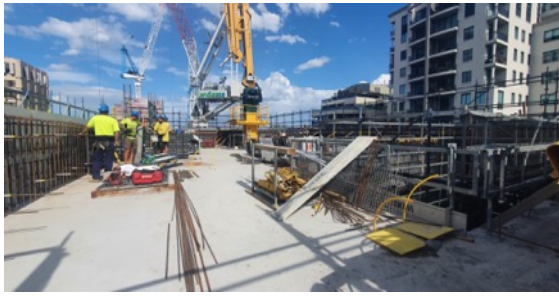
VCN – Level 4: VCN – Level 4 concrete pour completed.
