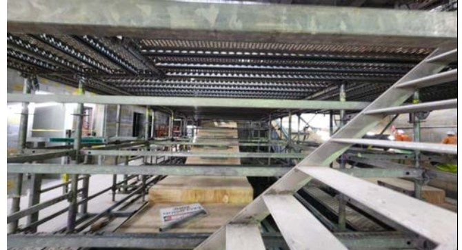
PSS: Escalator installation.
