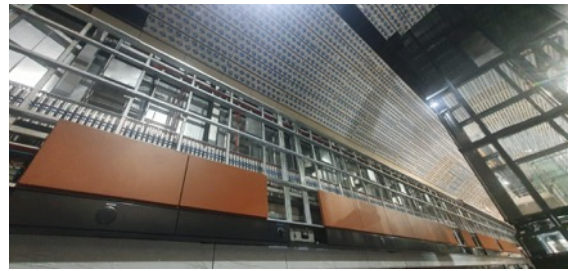
Station Cavern: Façade installation works progressing within Station Cavern.
