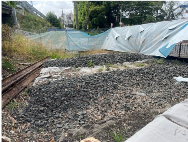
Ewart Street, Dulwich Hill: Robust ERSED controls well maintained on slope to stormwater inlet
