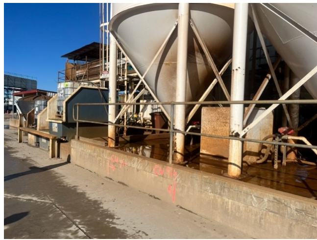
The Water Treatment Plant and surrounds were maintained in good condition
