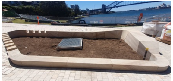
Blues Point Road – Streetscaping worksite: Installation of raingarden ongoing
