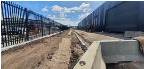
SMTF S: Drainage and landscaping works have commenced along fencing.
