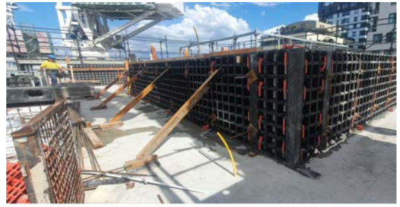
VCN – Level 4: Form and reo work for vertical wall underway.
