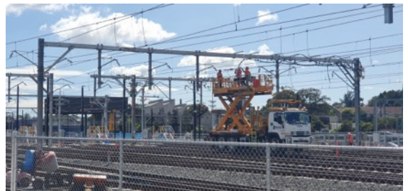
SMTF S – Stabling Yard: OHW works continuing.
