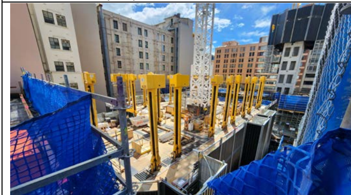
PSN south-eastern (Castlereagh Boutique Hotel) side : OSD level 6/7 Jumpform
