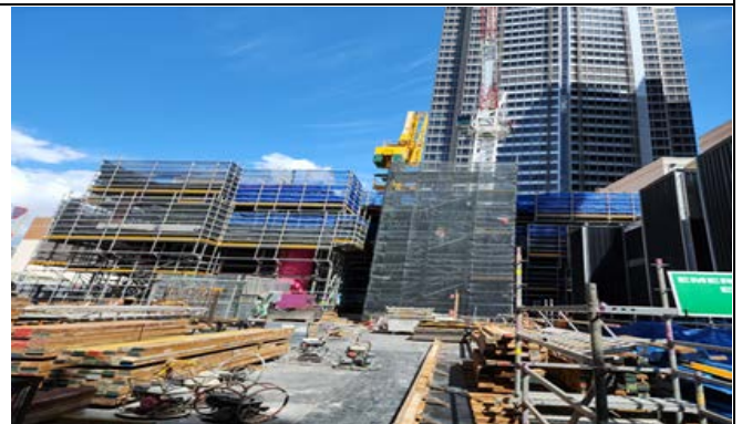
PSN south-western side: Level 6 FRP
