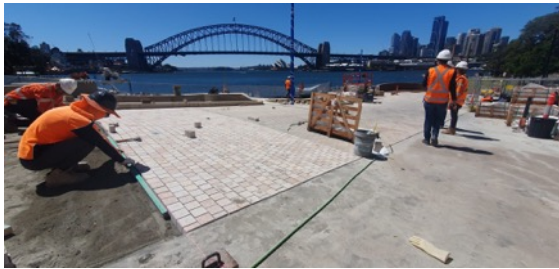
Blues Point Road – Streetscaping worksite: Paving works ongoing
