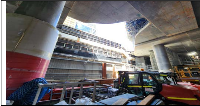
Pitt Street North (PSN): Level 00 Station Atrium.
