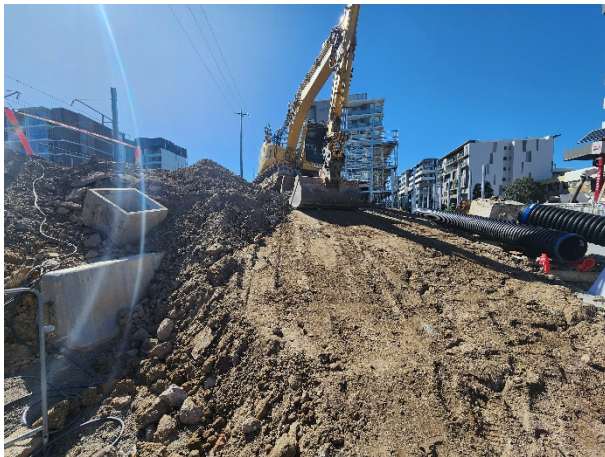
Canterbury MSB – New access ramp
