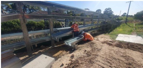
Dulwich Hill TSS: GST works progressing
