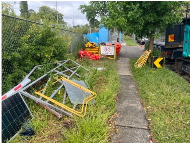
Material storage outside the corridor fence, Livingstone Road bridge, Marrickville
