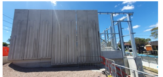
Punchbowl TSS: Partial façade installation works completed in WE19
