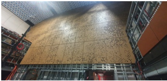
Station Cavern: Façade installation works progressing within Station Cavern.
