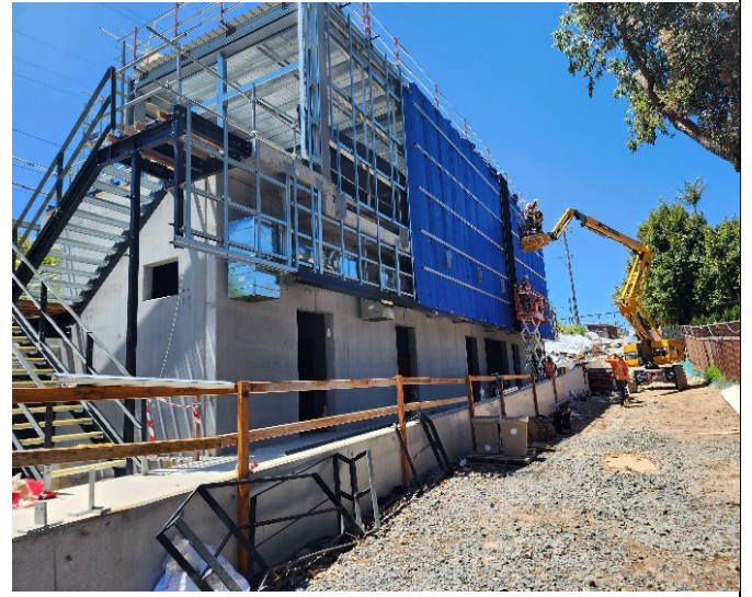
Hurlstone Park: MSB cladding installation
