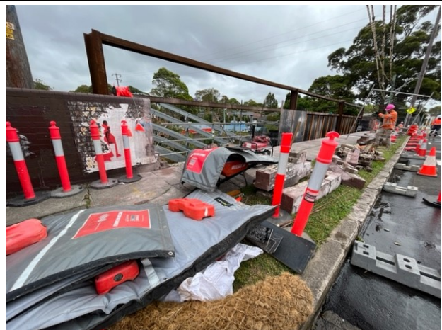
Parapet removal in preparation for throw screen installation, Livingstone Road Marrickville
