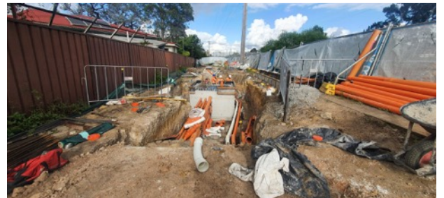
Dulwich Hill TSS: CSR pit installation (Pkg 630 CSR works) underway
