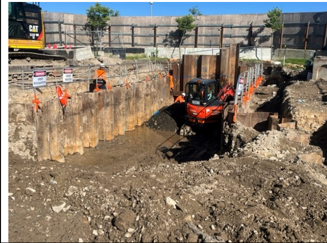
Excavation for the western civil pit had commenced
