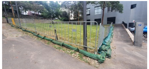
Surry Hills BPS Works - Frog Hollow Reserve: Grass trimming completed. Sediment controls remain.
