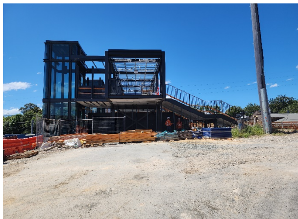
Dulwich Hill: Installation of the pedestrian bridge, stairs and lift shaft.
