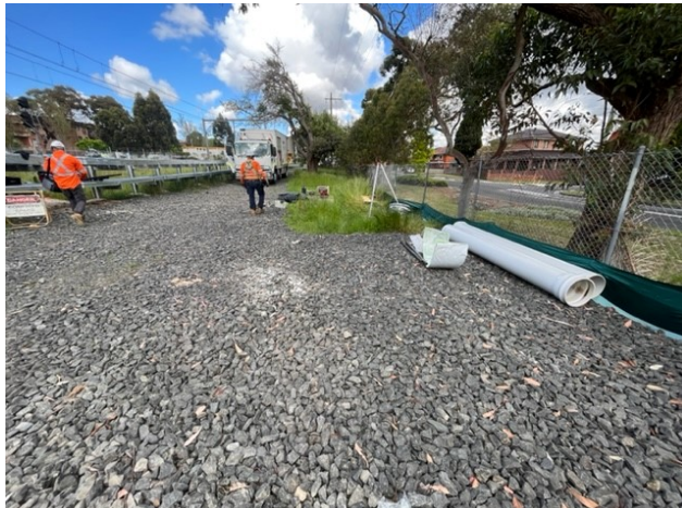
Culvert relining works at Rosemount Street, Punchbowl
