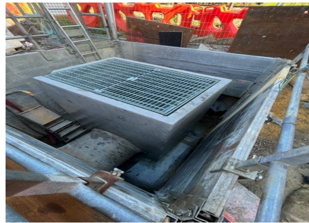
Stormwater pit installation at Hutton Street, Hurlstone Park
