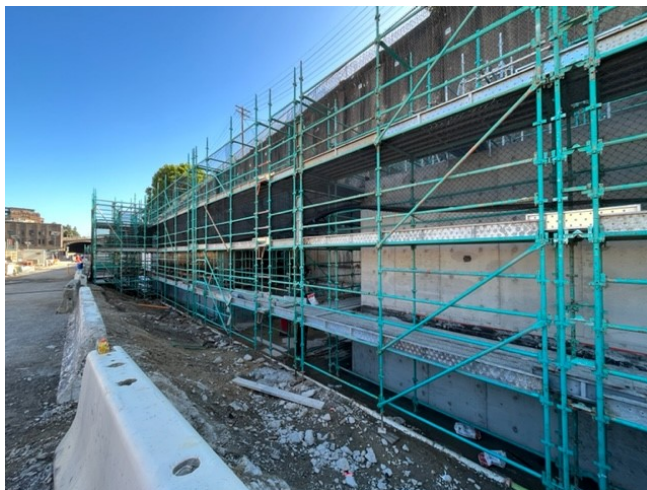
Construction of ventilation pods under the Hickson Road wall was ongoing
