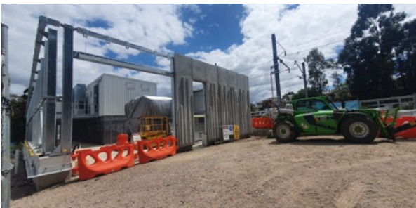
Punchbowl TSS: Partial façade installation works completed in WE19
