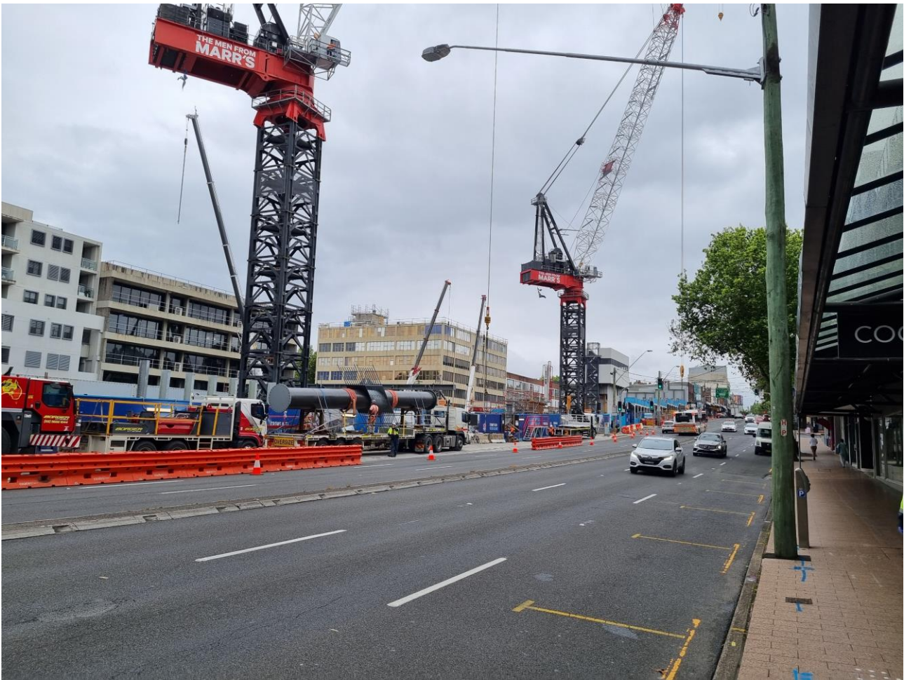
Plate 3 – Tower cranes over Station box site with Pacific Highway in foreground
