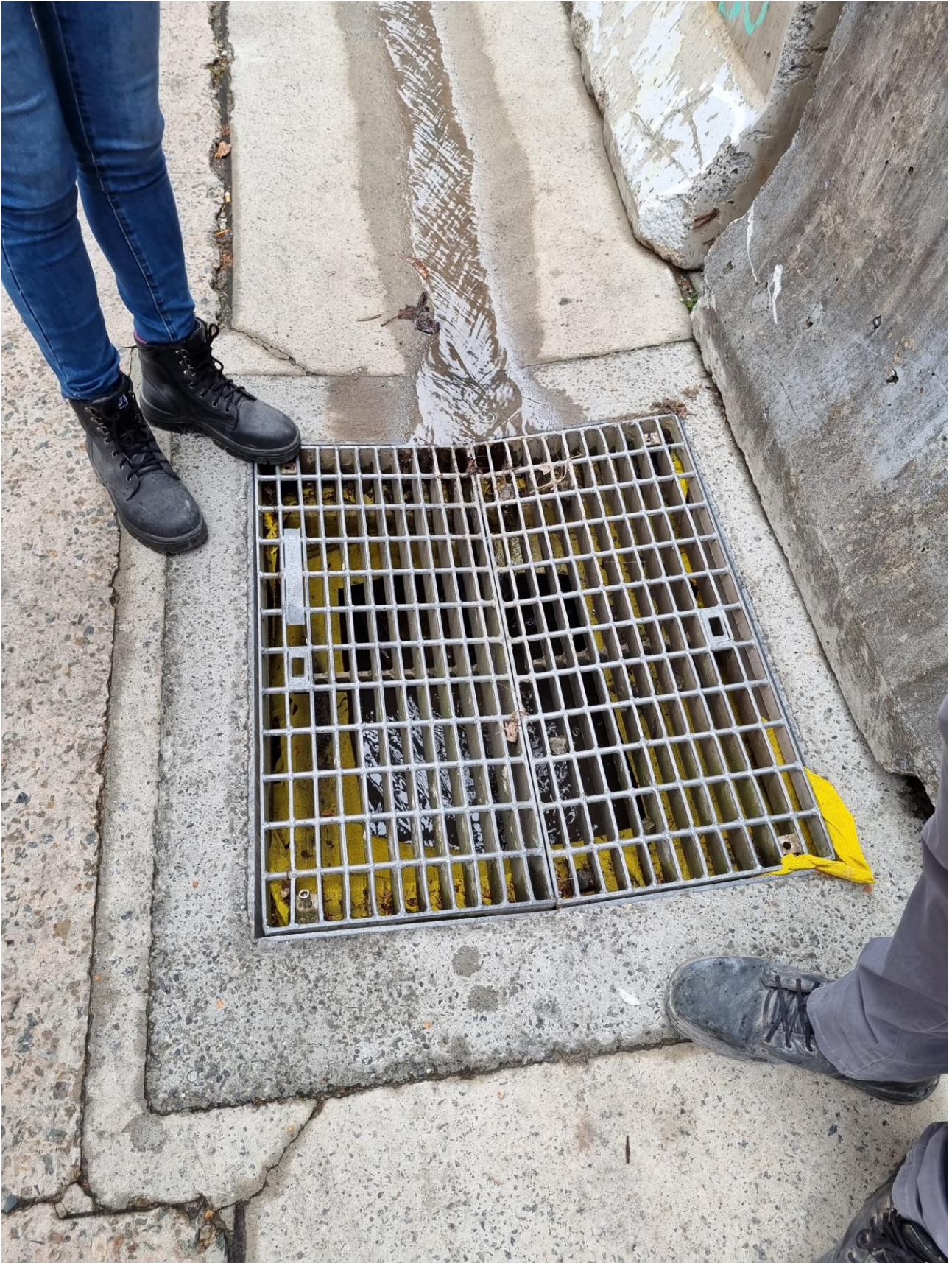
Plate 2 – Stormwater drain with internal drain guard installed
