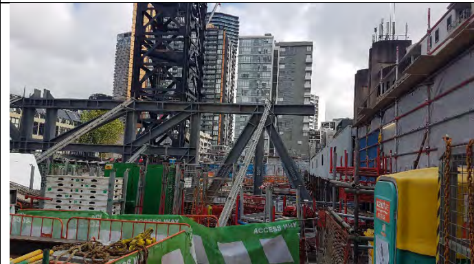
View north of B1/0 slab showing steel trusses in place
