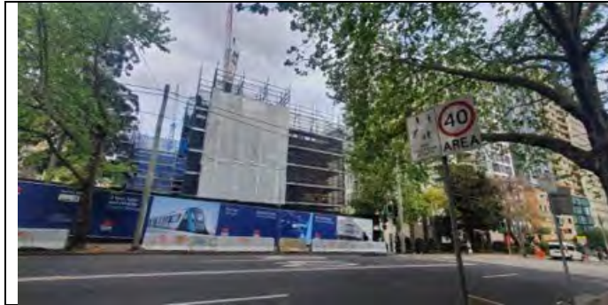
View of VCN (North Shaft area) from Miller St.
