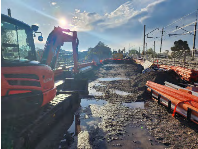
Marrickville CESS – ULX and shoring box installation
