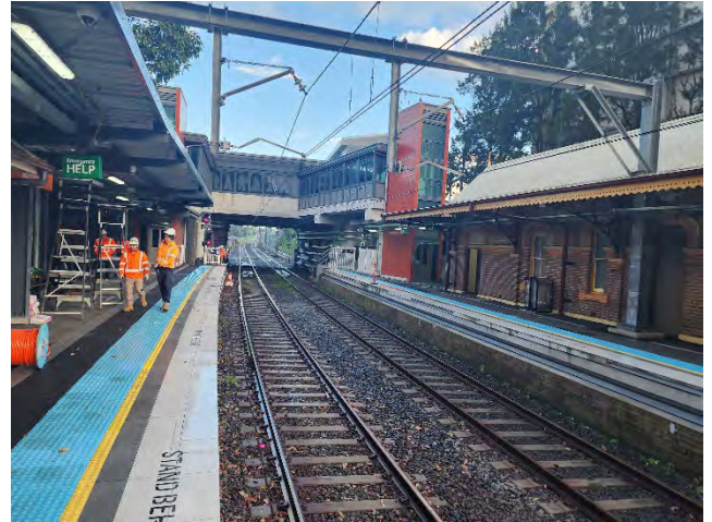
Marrickville platform electrical works and lighting pole installation
