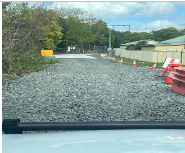
Belmore Triangle: New concrete driveway installed
