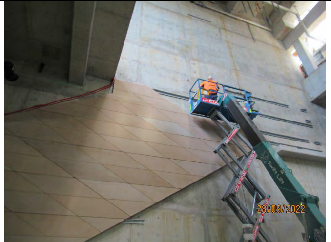
Fit out activities at the Eastern Entrance
