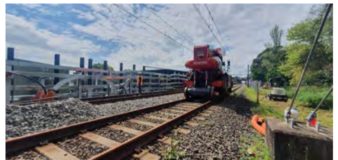
Zone 23.1 Wiley Park HV cabling – rollers set up on GST and running cable into GST.
