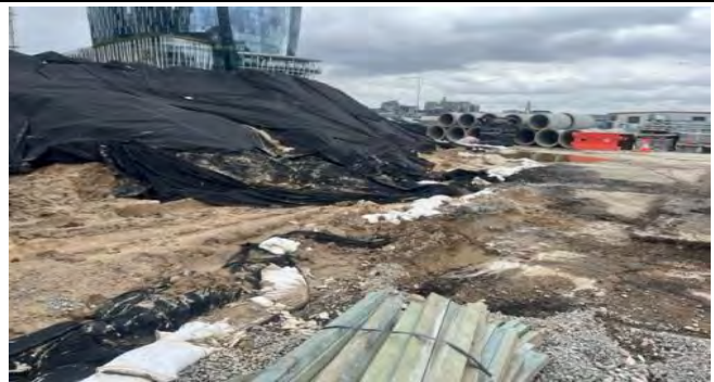
Controls for tunnelling spoil improved from inspection on 2/9/22 and later on 29/9/22
