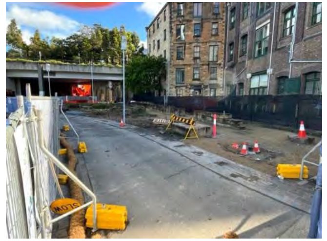
Tree removal works complete at The Cutaway
