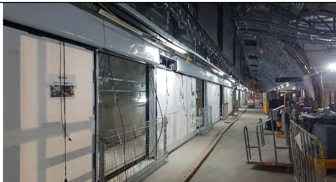
West Adit: Platform Sliding Door and cladding installation nearing completion
