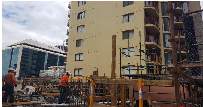
PSS - Level 6 FRP underway adjacent Princeton Apartments.
