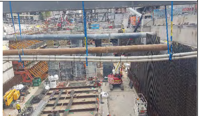
Hume St - Concrete Bridge removal completed
