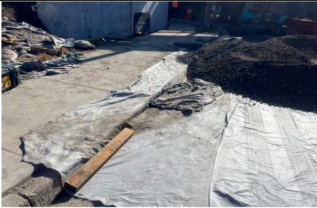
Wairoa Street Bridge, Campsie: Controls in place over road and drain during backfill of the retaining wall
