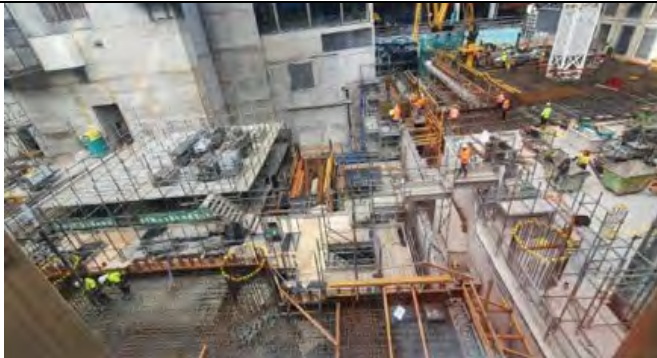
Victoria Cross South: Station Level B2 - concrete pour underway.
