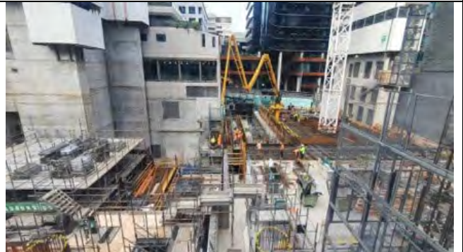
Victoria Cross South: Level B1 Carpark - concrete pour underway.
