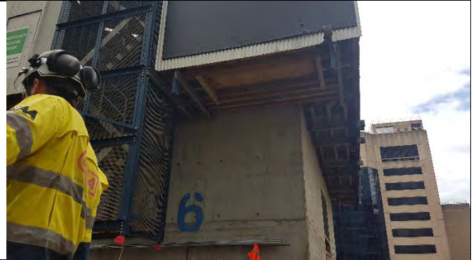
PSS: Core jump form at Level 7 - into OSD space.
