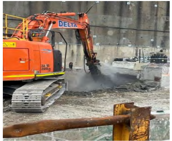
Demolition of the Hickson Road corbels
