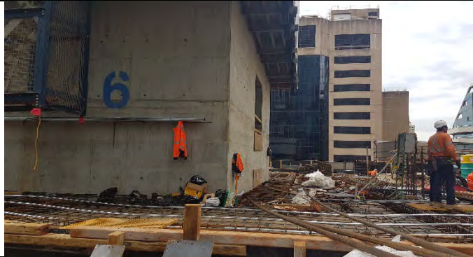
Pitt St South (PSS): Level 6 slab FRP.
