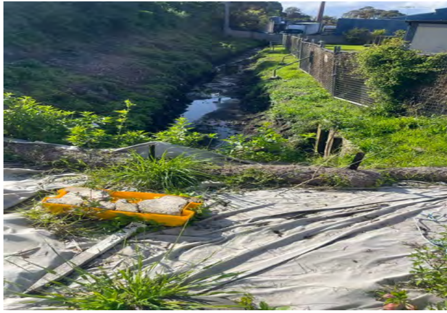
Victoria Road Bridge, Marrickville: Controls in place above culvert
