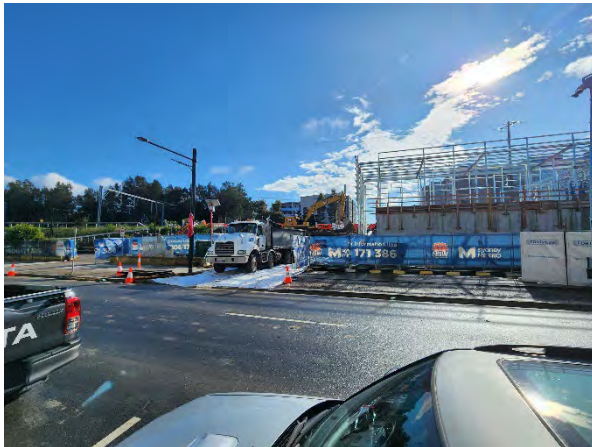
Canterbury MSB and loadout of spoil
