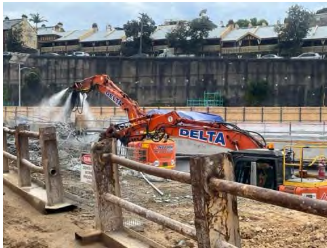
Demolition of the Shark's Fin headwall and capping beams
