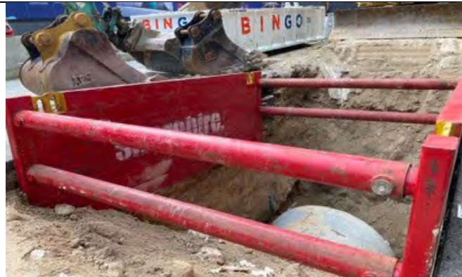
Denison St: Stage 3 stormwater works underway.
