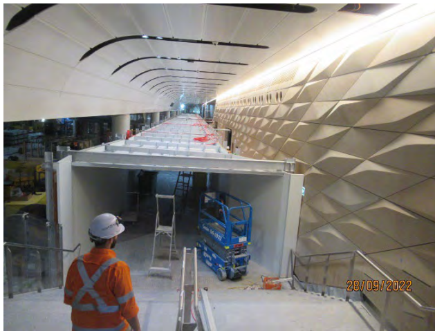
Construction of temporary pedestrian access in the North-South Concourse
