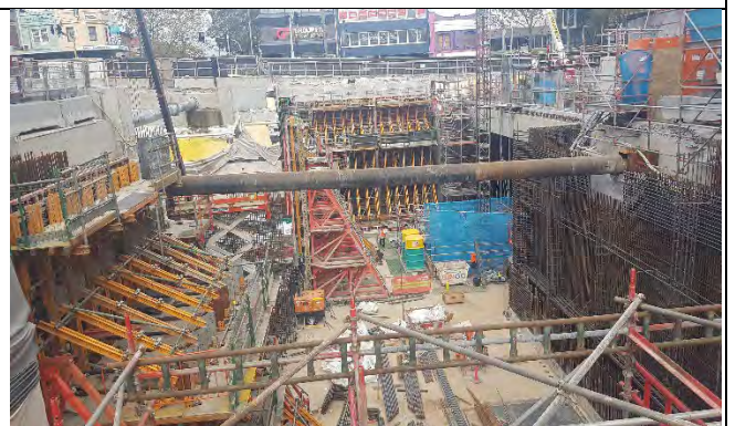
Site C view west – Perimeter wall shuttering and FRP
