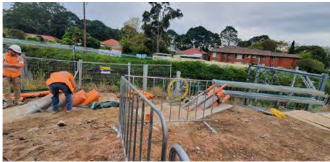
Dulwich Hill TSS – Man drilling conduits from TSS building
