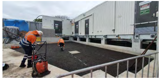
Dulwich Hill TSS- Asphalting works underway at TSS.
