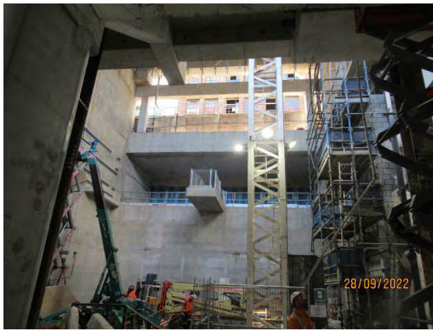
Eastern Entrance works
