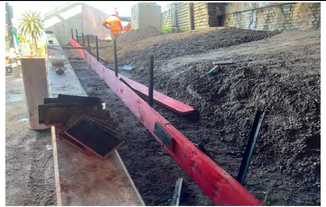
Wairoa Street Bridge, Campsie: Controls in place over road and drain during backfill of the retaining wall
