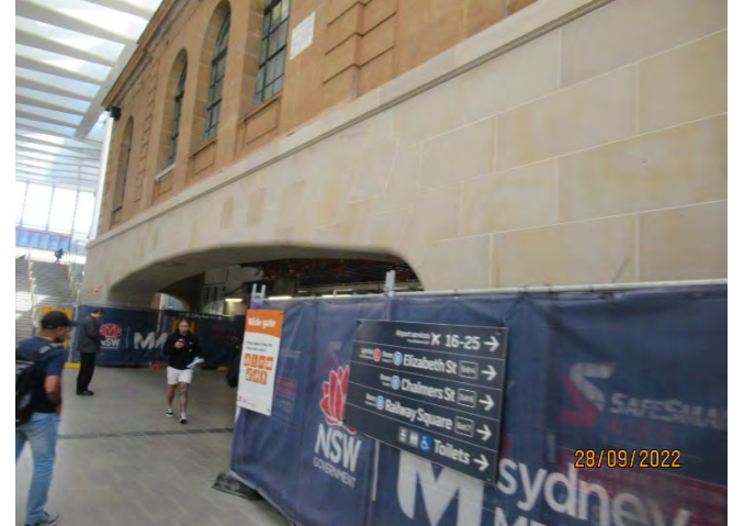
Northern Concourse: Completed cladding of the beam under the ICAC Building.
