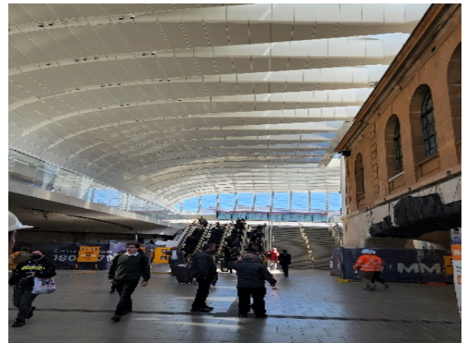
Northern Concourse: Ongoing cladding of the beam under the ICAC Building.
