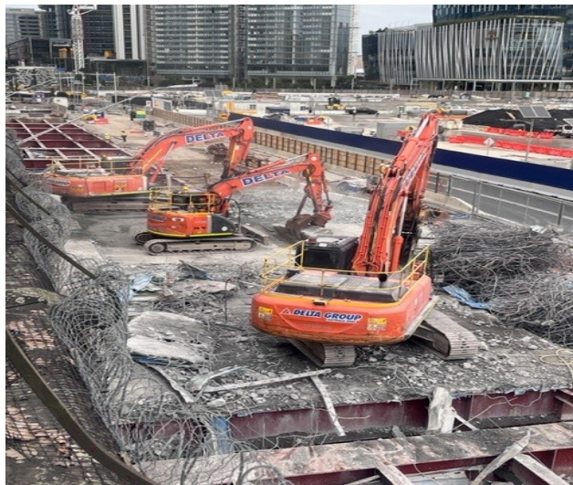
Demolition of the Hickson Road bridge deck and crane in place for transfer of steel beams OOH
