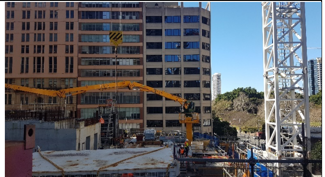
PSN: South-eastern Level 3 Slab completed.
