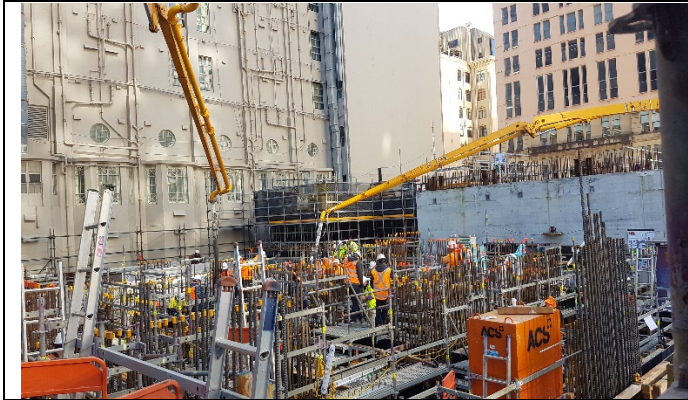
PSN south-eastern side: Central (OSD) kicker wall concrete pours from Level 3
