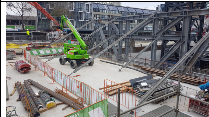
View Northwest - B/B0 central slab and steel trusses
