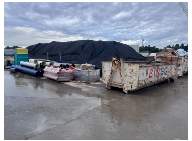
Rozelle tunnelling spoil – covered and controls in place
