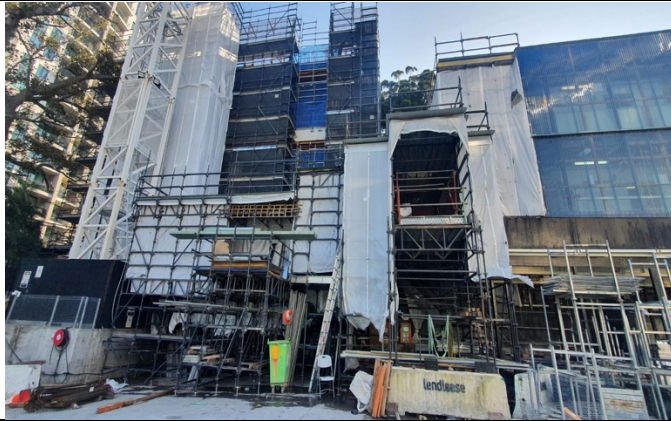
Victoria Cross North Shaft: Level 2 form works completed.
