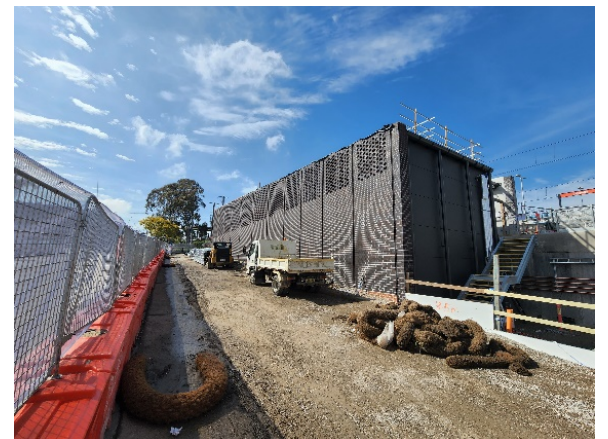
Lakemba– MSB and ESC maintenance undertaken during inspection.
