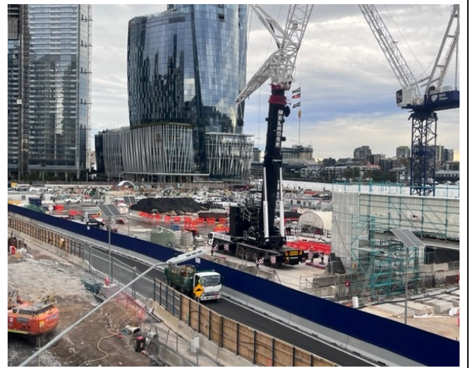
Demolition of the Hickson Road bridge deck and crane in place for transfer of steel beams OOH
