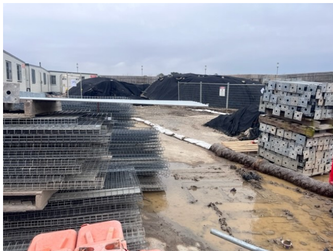
Covered stockpiles of hazardous waste awaiting load-out
