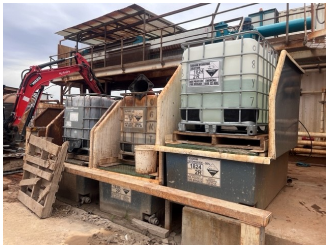
Hazardous chemical storage area adjacent to the WTP. Accumulated mud and debris observed.
