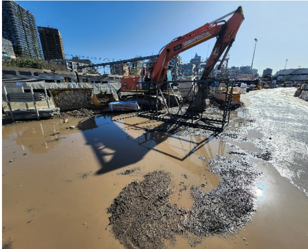
Water management required at the Sydney Yard
