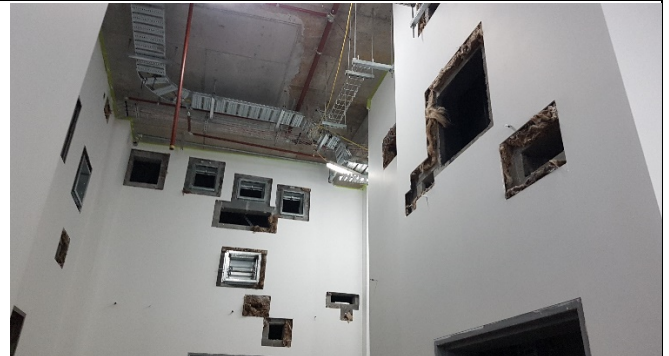
PSS B1 internal walls painted with HVAC penetrations
