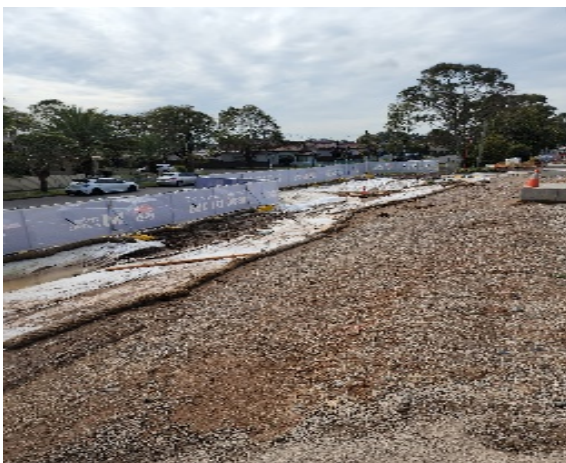
Punchbowl: Southern drainage works.
