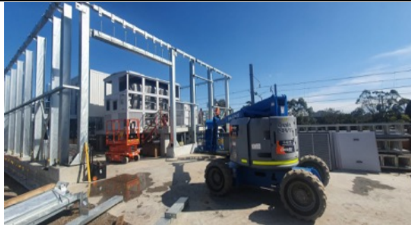
Lakemba TSS: Structural steel installation for TSS façade.
