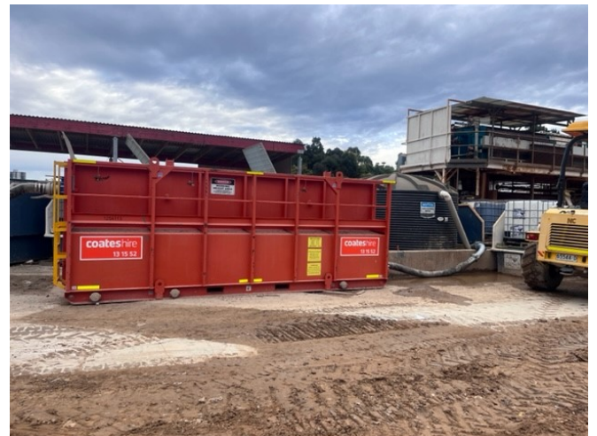
Sediment settling tank brought to site post-E107 incident on 13/7/22
