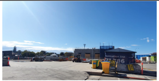
Chatswood Dive Site - Acoustic gantry shed removed (across WE05/WE06 possessions)
