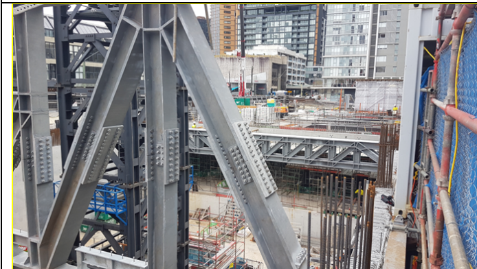
View north of B1/0 slab showing steel trusses in place
