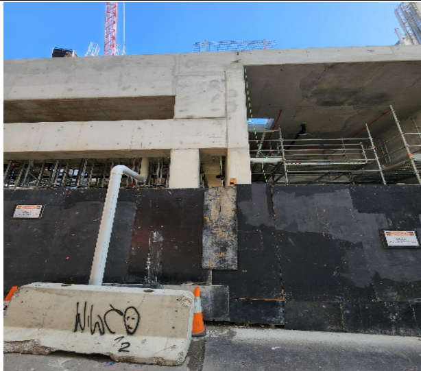
Eastern Entrance works (and noise monitor location)
