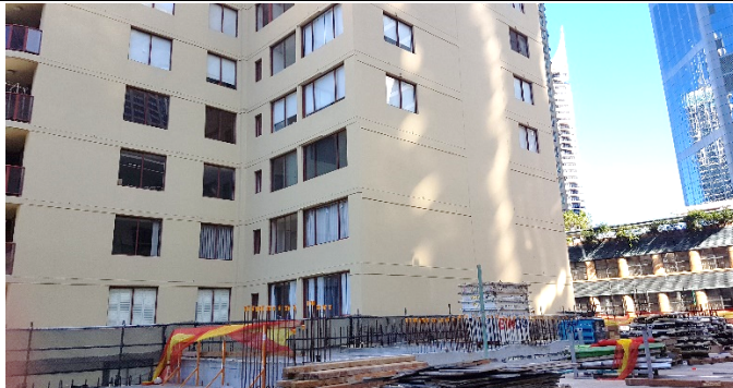
PSS - Ventilation shaft to Level 5 with Level 5 slab FRP underway.
