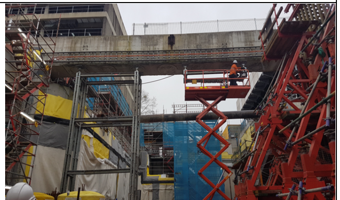
Site C view east – Capping beam prop installation ahead of removal
