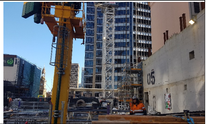
PSN south-western side: Level 5 FRP
