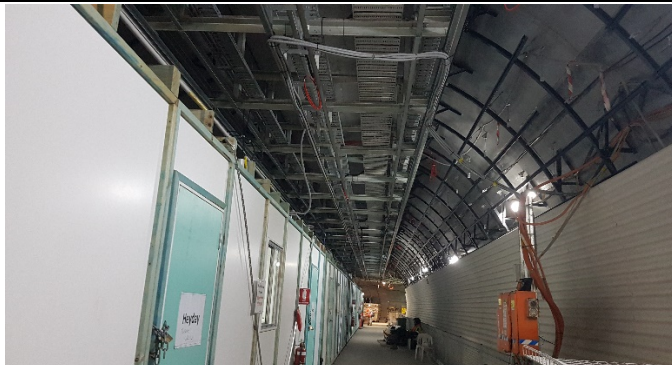
Northern Cavern: Services installation.
