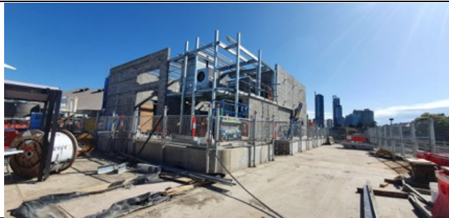
Chatswood Dive Site - Northern Dive Building blockwork progressing.
