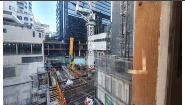
Victoria Cross South: Carpark jumpform is at Level 3.
