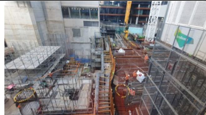
Victoria Cross South: Level B1 of Carpark - Steel tensioning works underway.
