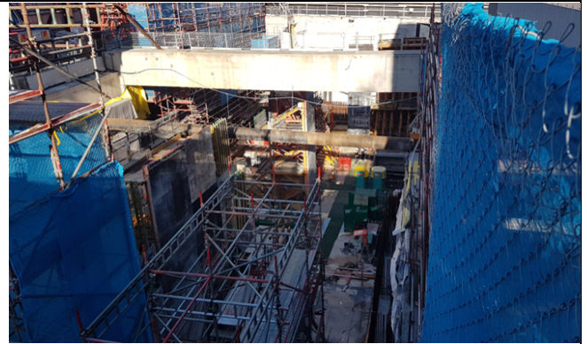
Site C view west– Capping beam remaining
