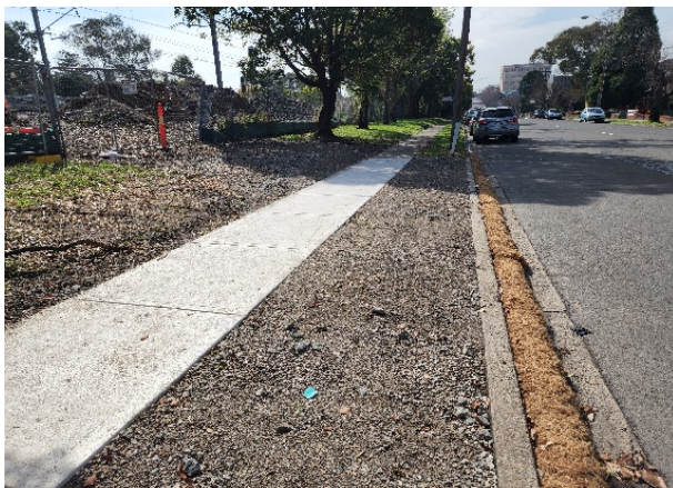
Lakemba – repair of footpath and rehabilitation of Council verge.
