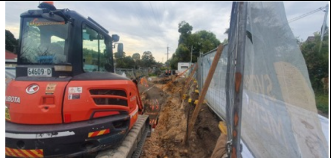
Dulwich Hill TSS: Bulk excavation for CSR package of works.
