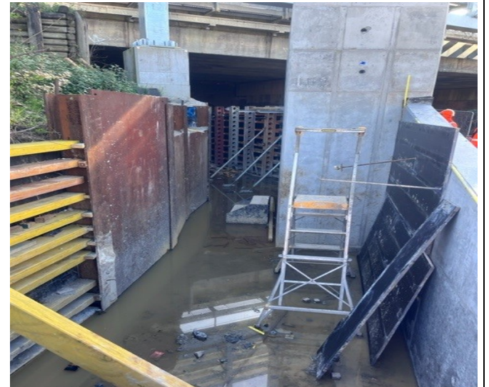
Wairoa Street Bridge, Campsie: Construction of the retaining wall was ongoing.
