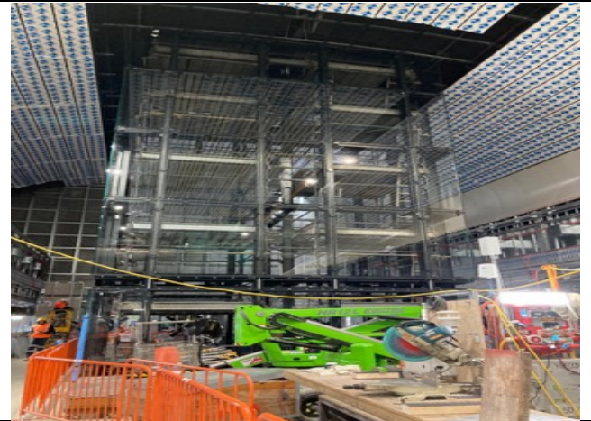
Station Cavern: Glass installation on lift.
