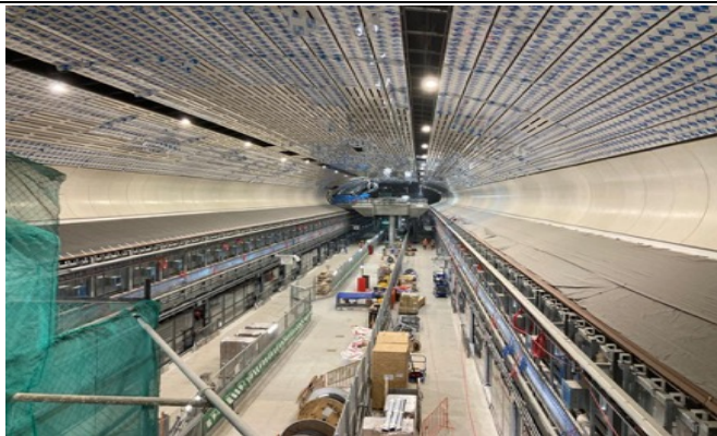
Station Cavern: Station fit out and GRC panels installation.
