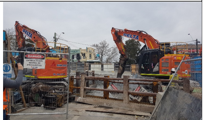
Hume St - Concrete Bridge tray removal with hammer
