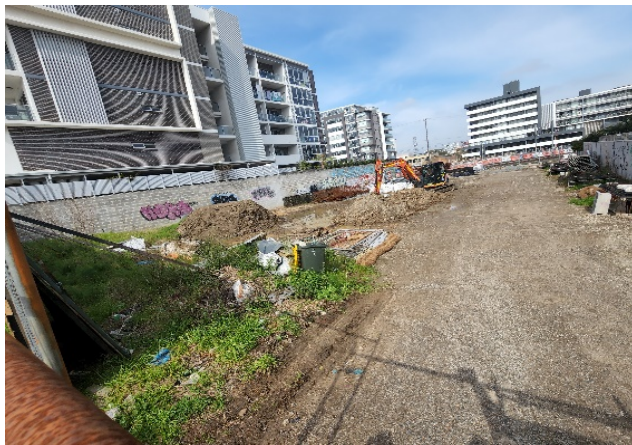
Canterbury 6 Broughton Street –ESC and stockpile management
