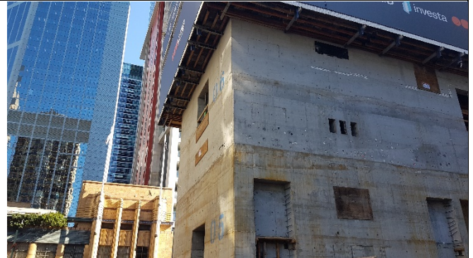
PSS: Core jump form Level 6 completed- into OSD space.
