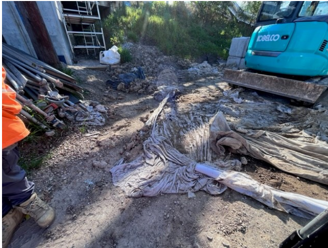
Wairoa Street Bridge, Campsie: ERSED controls requiring reinstatement and ongoing maintenance
