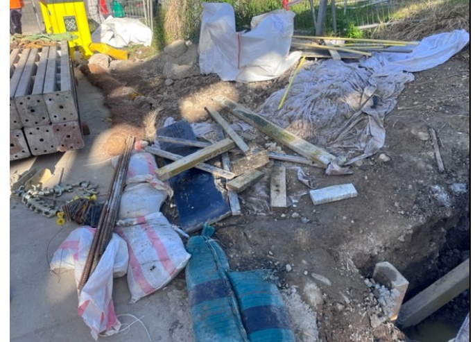
Wairoa Street Bridge, Campsie: ERSED controls requiring reinstatement and ongoing maintenance
