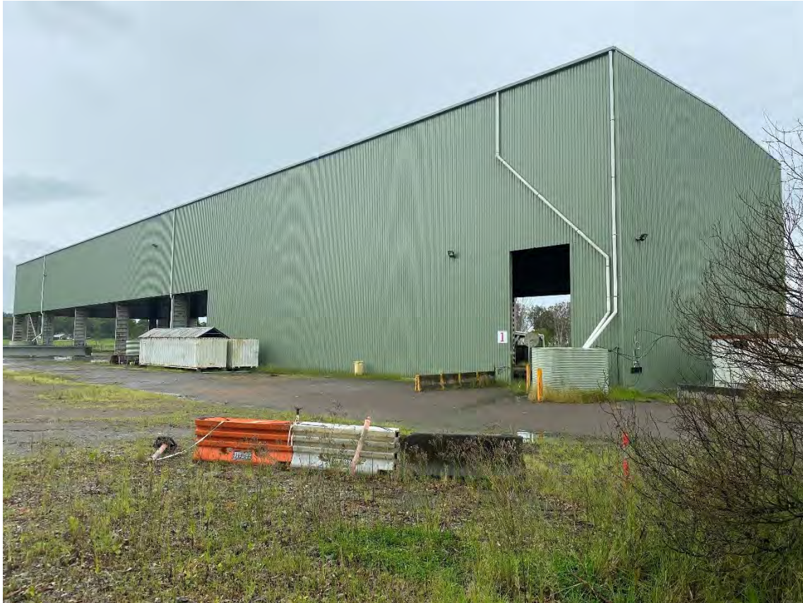
Figure 7-4: The Proposal site showing existing shed
