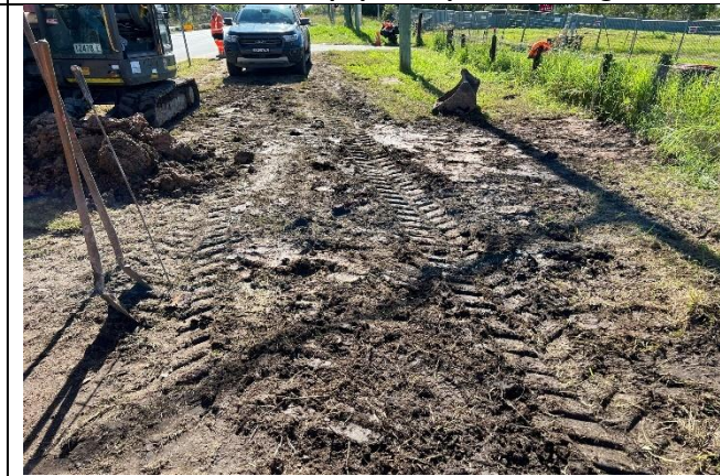
Power –Kent Rd trenching and HDD works
