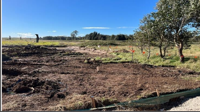
Elizabeth Drive view north: Area cleared, and subsurface preparation works underway.
