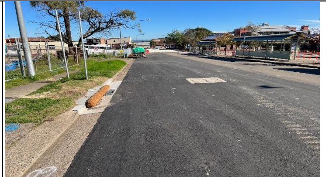
TBI Station Street West– Works completed
