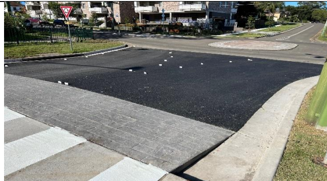
Philip and Lethbridge intersection re-sheeted
