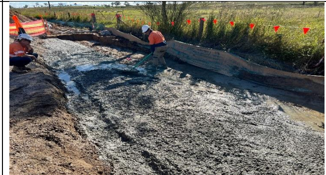
Elizabeth Drive: Services protection works.
