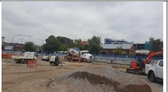
View northwest - Placement of temporary concrete stormwater diversion berm along Station St.
