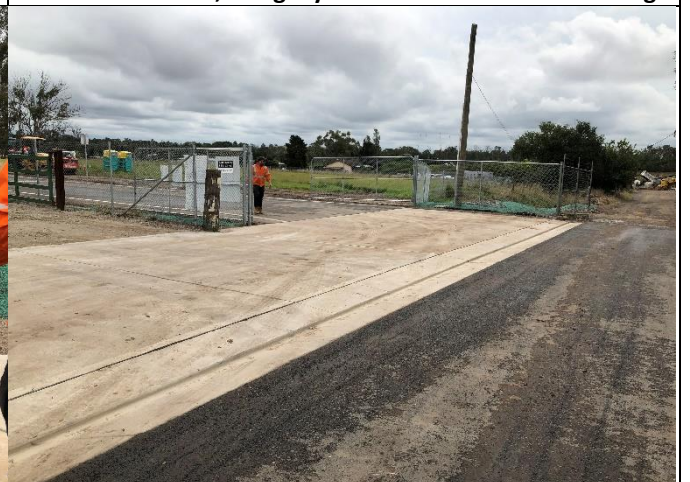
40 Derwent Road, Bringelly LIW view south – completed
