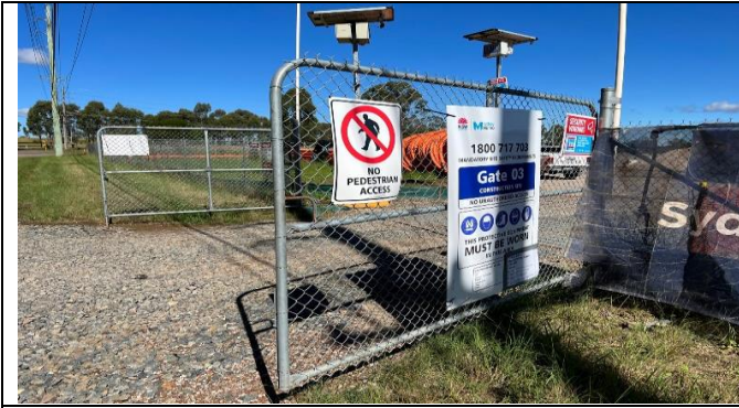
Power –Gipps Street compound gate signage per CoA E47
