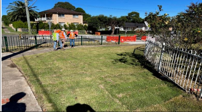
Philip and Lethbridge intersection works turfed.
