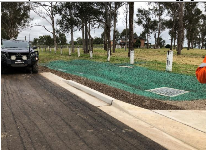
40 Derwent Road, Bringelly LIW view North – completed
