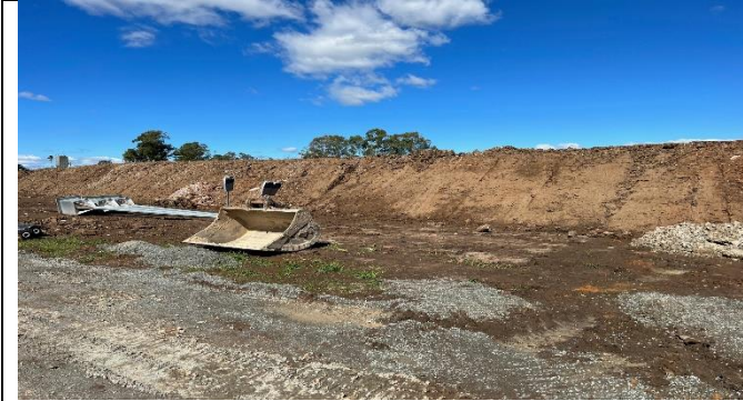
Power – Lawson Road compound southern bund
