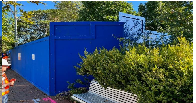
St Marys lift relocation – Hoarding view towards west.
