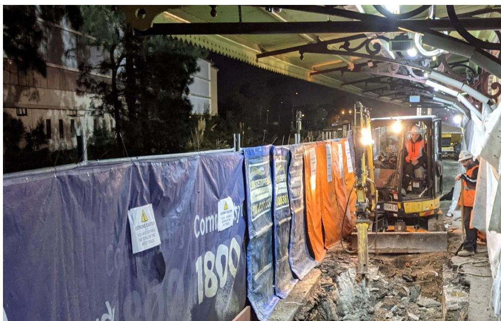
Marrickville station platform hammering (noise mats in use) – HSEJV supplied image
