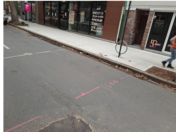
Route marking and minimum safe working distance check
