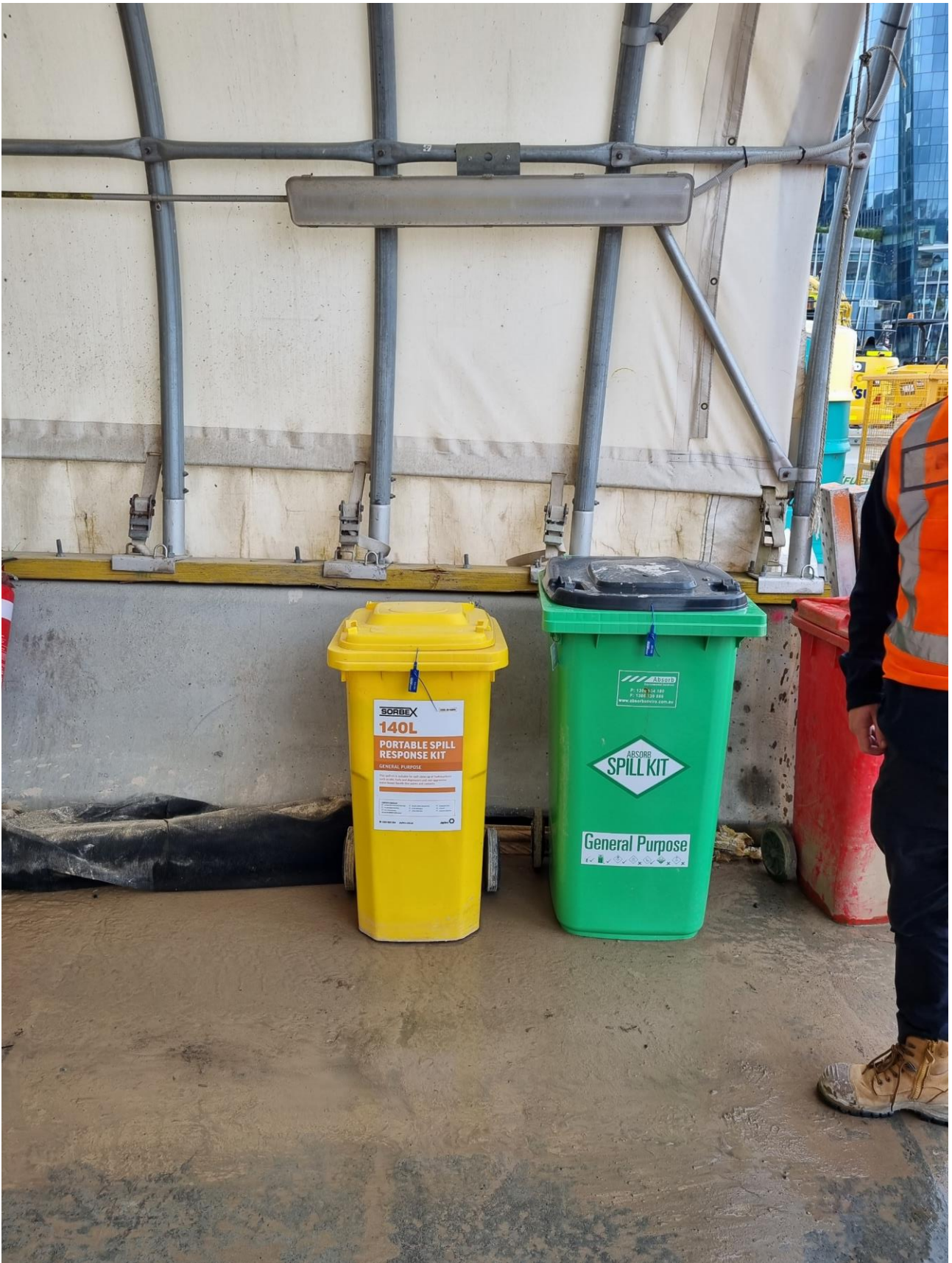
Plate 10 - Sealed spill kit containers in chemical store
