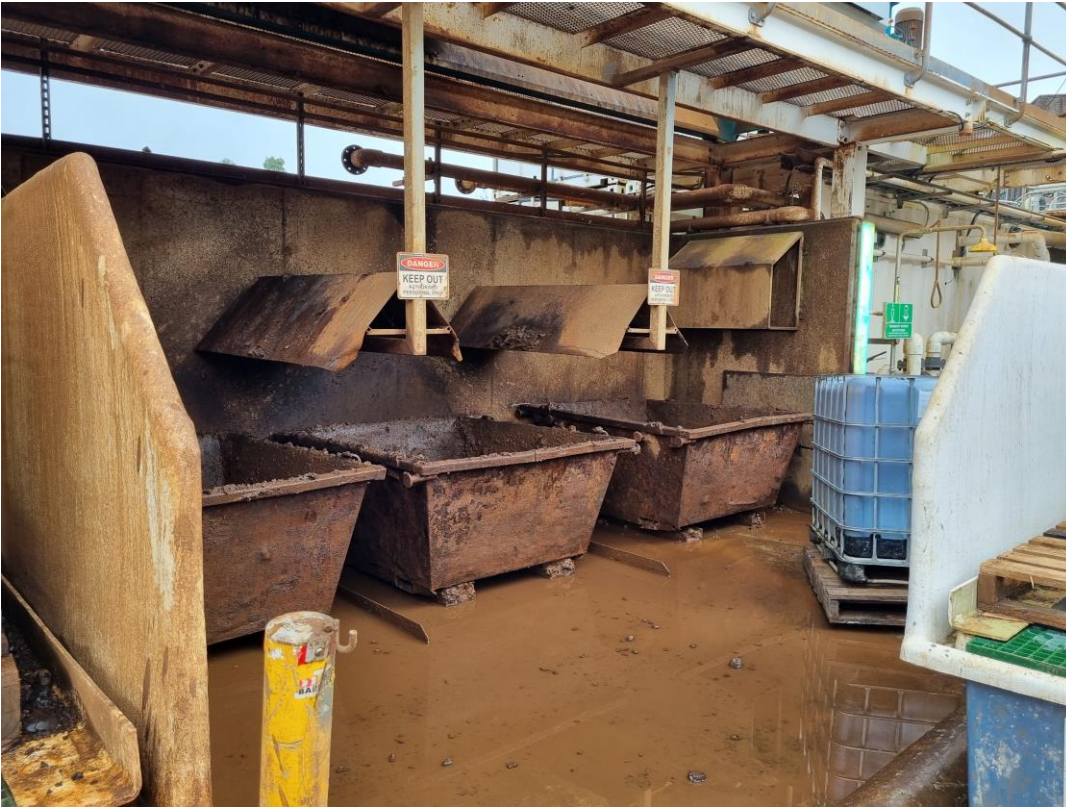
Plate 4 - WTP filter cake storage area well bunded
