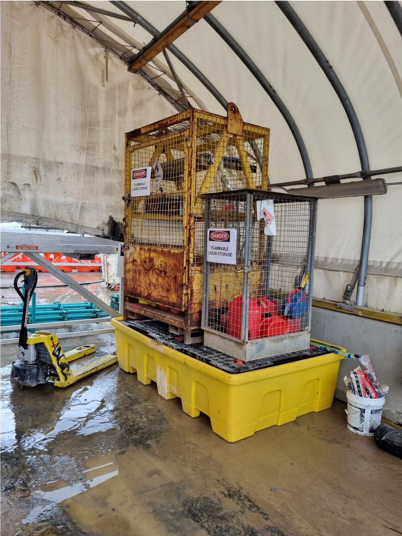
Plate 8 - Bunded and covered chemical store
