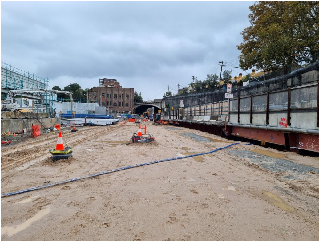
Plate 1 - Site stormwater being transferred via lay flat hose to WTP
