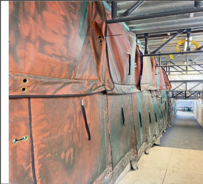
Victoria Cross North: Use of internal noise blankets observed.
