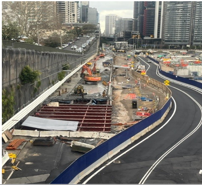
Hickson Road temporary road realignment and demolition of the old Hickson Road bridge deck
