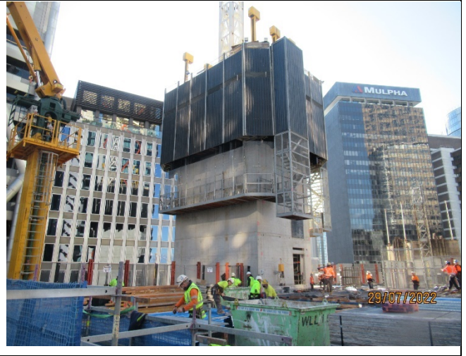
Martin Place North – Works well above Level 12 (above the SSI level).
