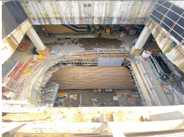
Last Mole Hole in Traffic Deck – air ventilation removed
