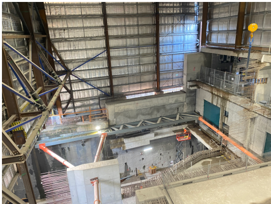
Campsie TSS: Concrete panel installation completed on TSS façade. TSS scheduled to be energised in August 2022.
