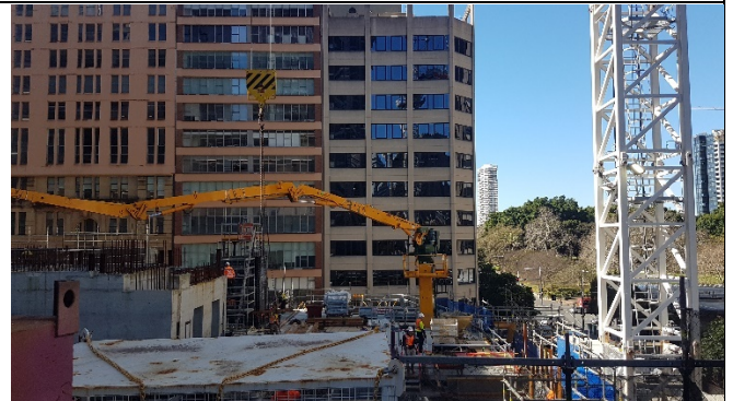
PSN: South-eastern Level 3 Slab completed.
