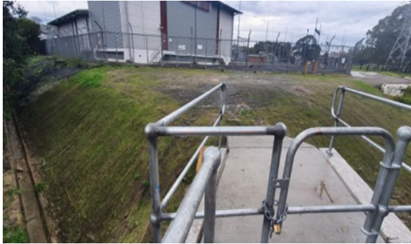
Pat O' Connor Reserve - Cable Bridge Site (Ausgrid side): Batter recently spray-grassed; some green growth observed on batter.
