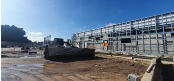
Southern Dive - Services Building: Cladding installed on section of Services Building; with steel installed for cladding installation on exterior of building.
