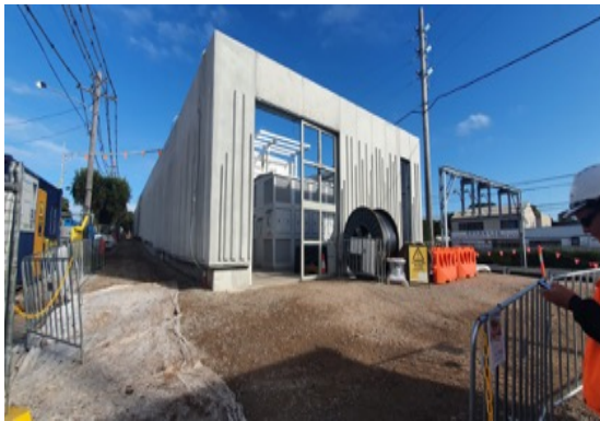
Campsie TSS: Concrete panel installation completed on TSS façade. TSS scheduled to be energised in August 2022.
