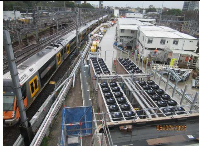
View from top of the Ventilation Building
