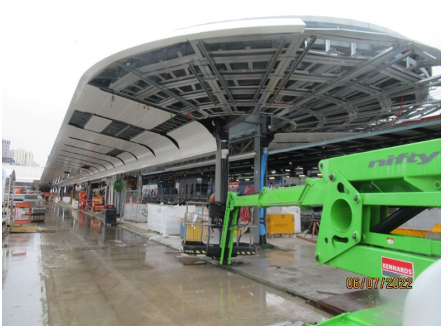
Canopy on Platform 14
