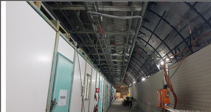
Northern Cavern: Services installation.
