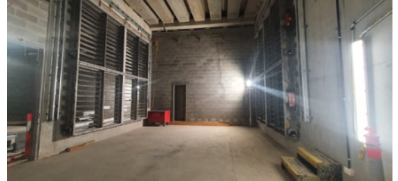
Southern Dive - Fan room: Noise dampeners pending installation in the Fan Room.
