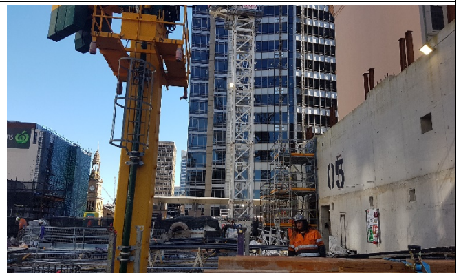
PSN south-western side: Level 5 FRP
