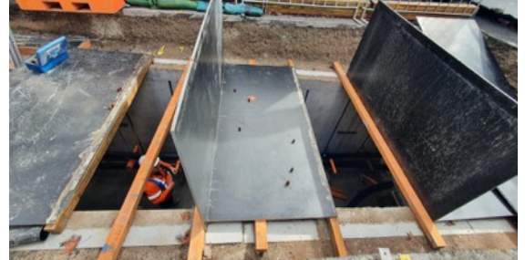
Southern Dive - Fan room: Noise dampeners pending installation in the Fan Room.
