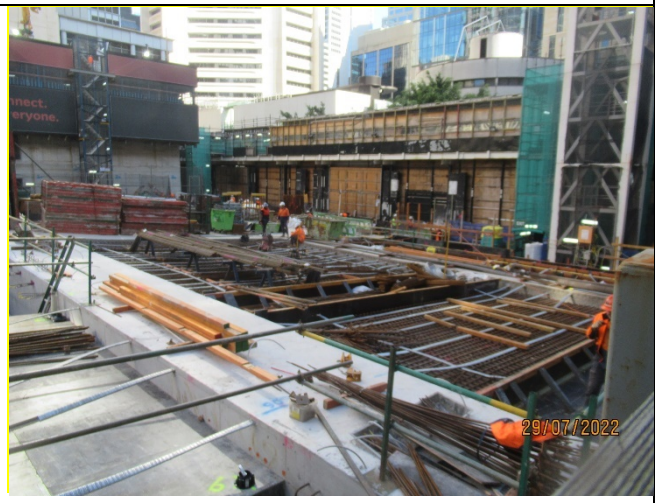
Martin Place South – FRP works ongoing
