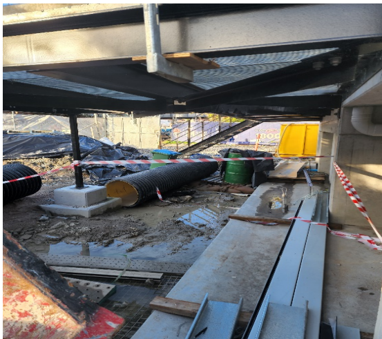
Marrickville MSB – Groundwater drums requiring appropriate bunding.
