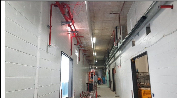
Level B3 Internal walls painting and services installation
