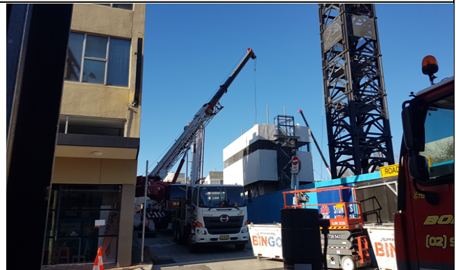
Clarke Lane South – Mobile crane operations in support of tower cranes
