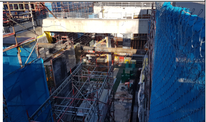
Site C view west– Capping beam remaining
