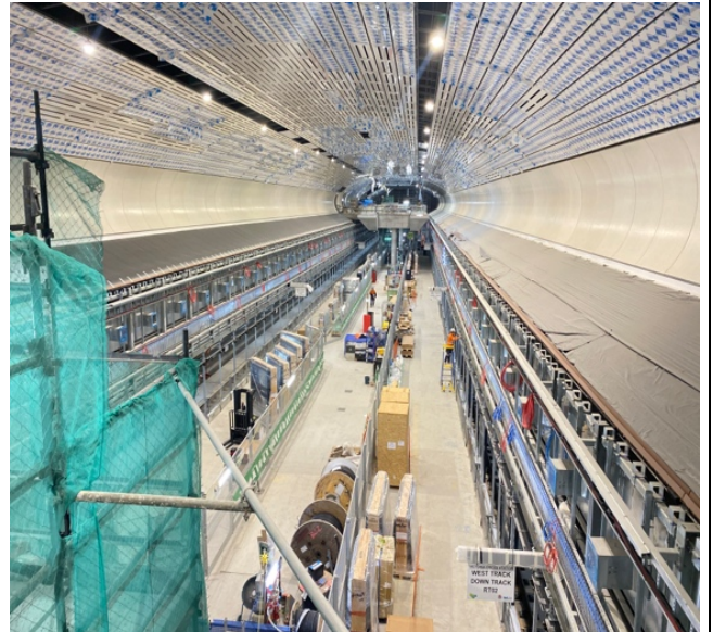
Station Cavern: GRC panel installation /station fit out
