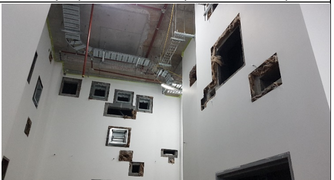
PSS B1 internal walls painted with HVAC penetrations
