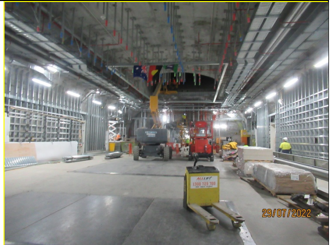
Caverns– ongoing fit out works.
