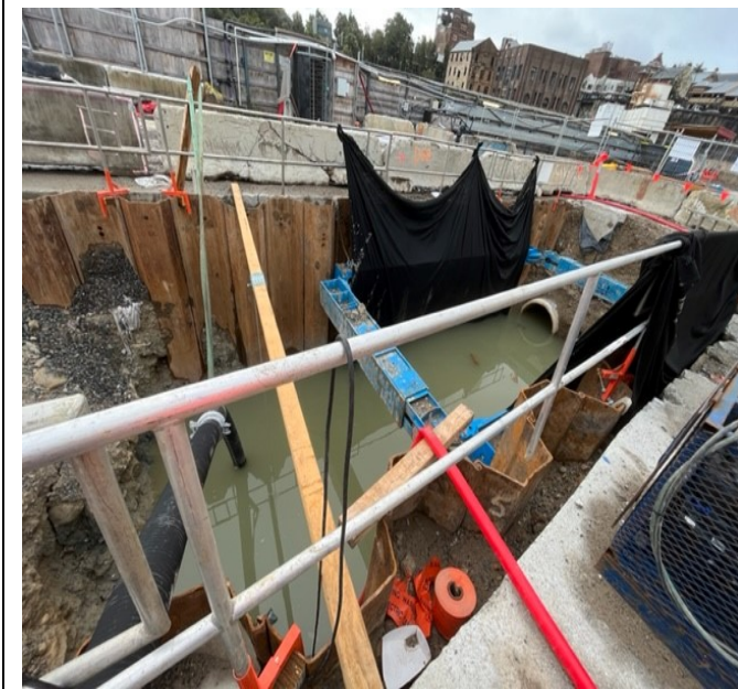
Trench from which dewatering occurred during incident on 13/7/22
