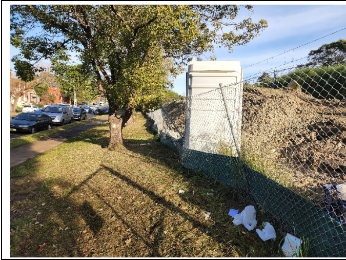
Lakemba – Rail segregation fence
