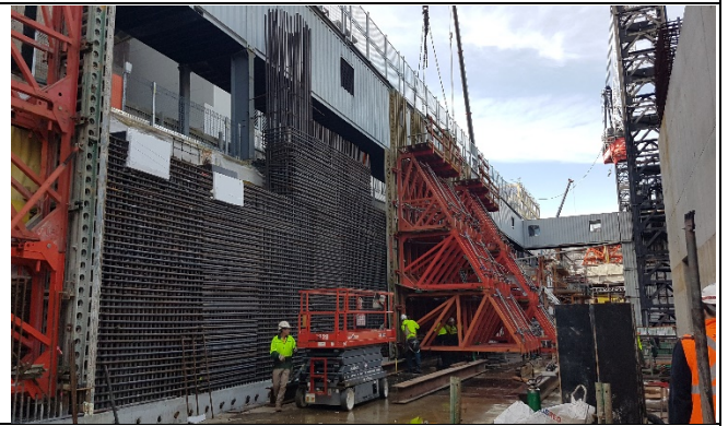
Level B2 view South - Slab Steel fixing and formwork
