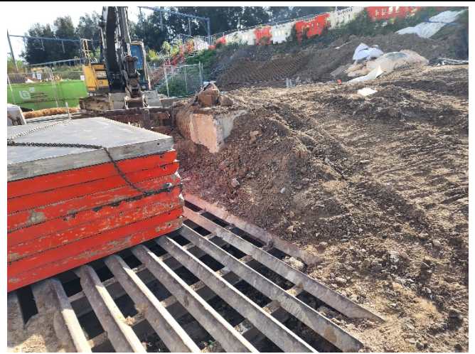
Canterbury MSB – rumble grids clean, spoil movement ongoing.
