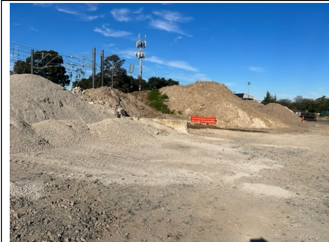
Belmore Triangle: Excessive stockpile height, no cover
