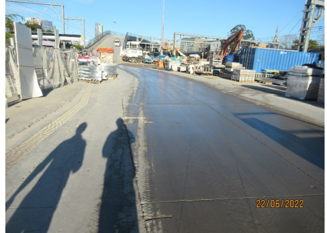
Sydney Yard – laydown and spoil management area
