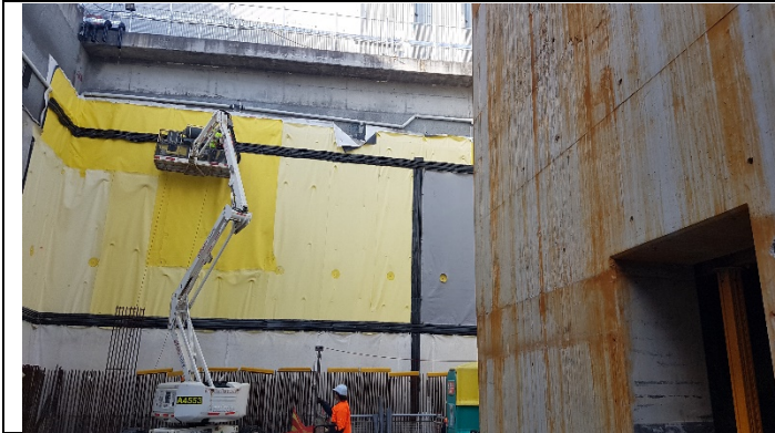
Level B2 South: Waterproofing repairs.
