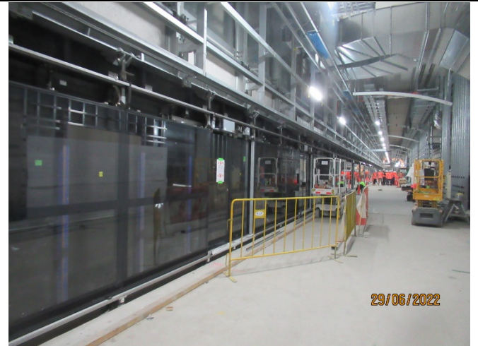
Stations – installation of sliding doors on platforms
