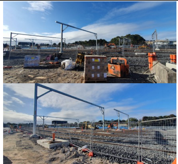
SMTF S: Rail works – resurfacing, rail adjustment and ballast placement
