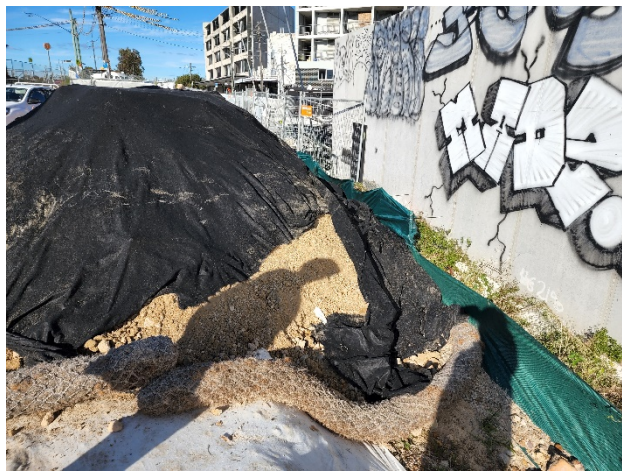
Dulwich Hill: Stockpile in drainage line
