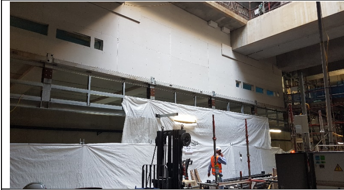
Level B4 - Over Track Exhaust (OTE) external cladding works
