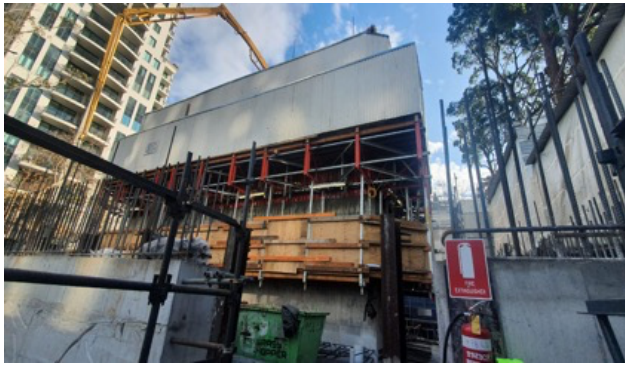
Station Cavern: Installation of lift risers.
