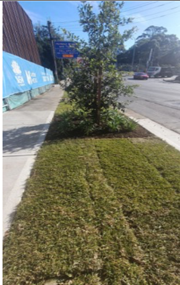
Artarmon TSS - Landscaping works completed
