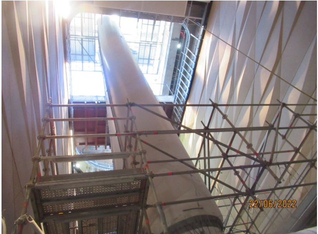
One ventilation removed from Mole Hole 3.
