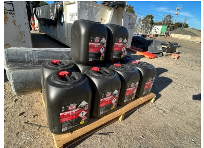
Belmore Triangle: HCL with no secondary containment
