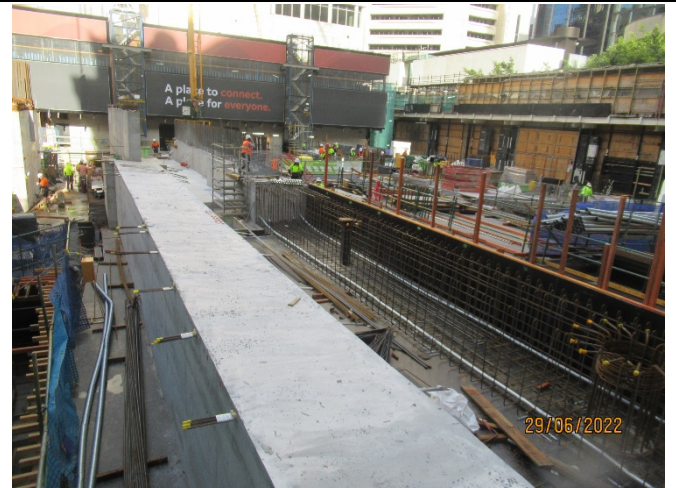
Martin Place South – FRP works ongoing
