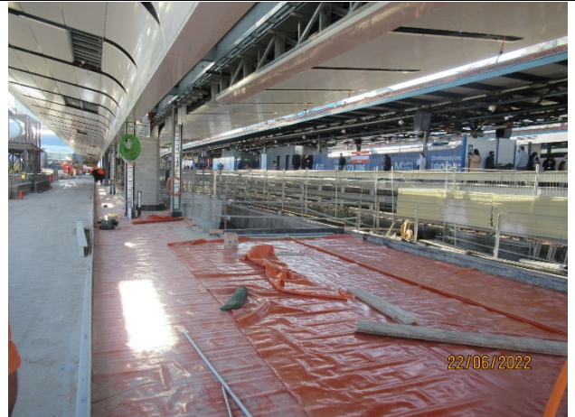
Traffic Deck and new canopies on Platforms 12/13 and 14.
