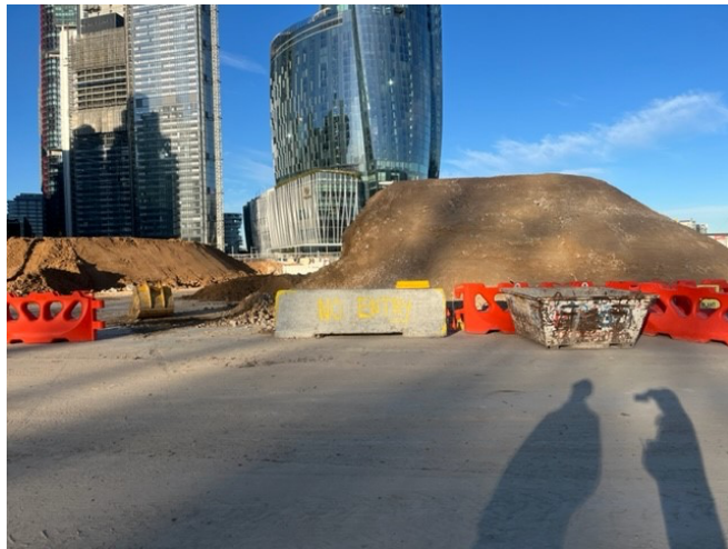
Stockpiles of tunnel spoil from Rozelle Interchange (to be covered after dust complaints)
