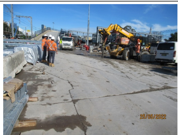
Sydney Yard – laydown and spoil management area
