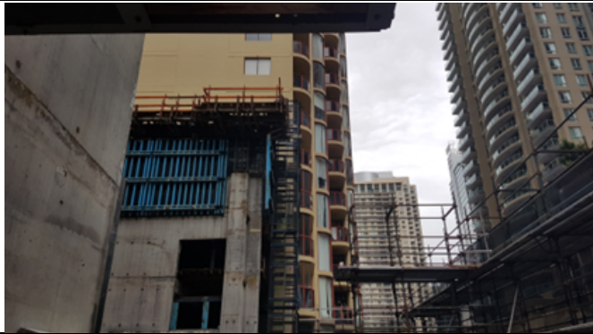
PSS - Ventilation shaft jump-form dismantle.
