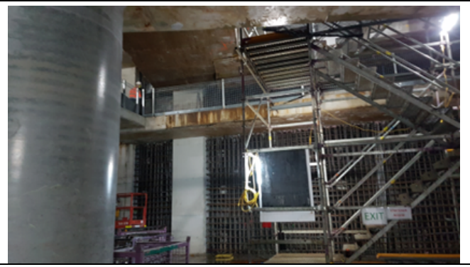
PSN: B2 Southern wall steel fixing for shotcrete
