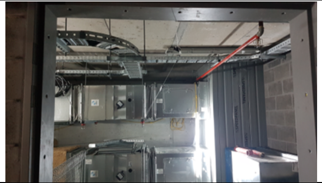
PSS B4 HVAC installation
