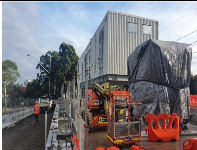
Punchbowl TSS: Modular buildings and transformers delivered/ installed during WE45 possession
