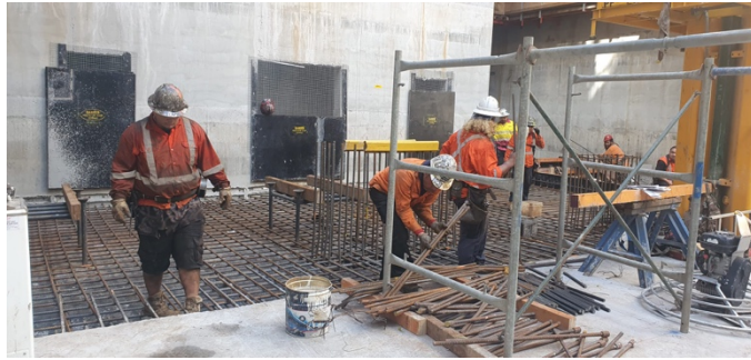
Victoria Cross North: Level B4 - Steel fixing works in progress
