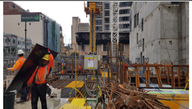
PSN: Southwest Level 2 FRP
