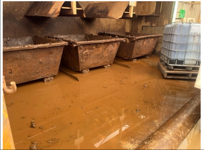
Filter cake receiving bay of the WTP
