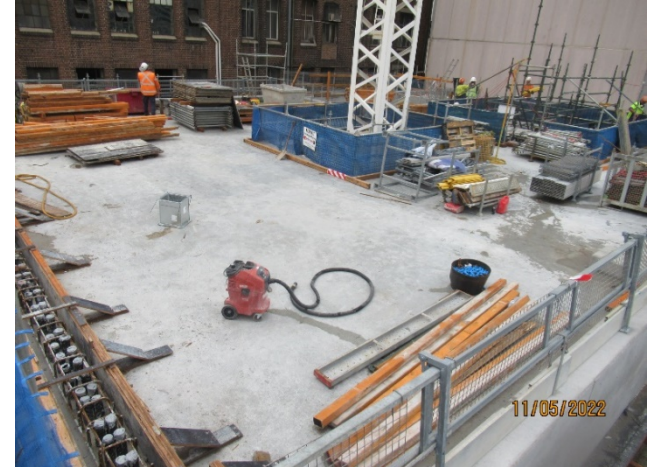
Concrete pour on roof of the Eastern Entrance
