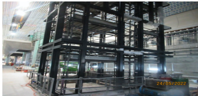
Station Cavern: Installation of lift risers.
