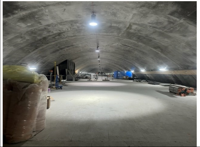
The air plenum above the crossover cavern
