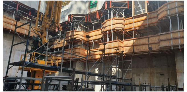
Victoria Cross North: Slip Form at Level B2
