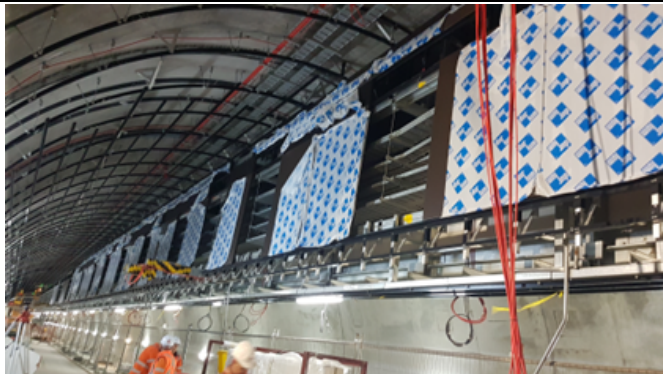
East Adit: OTE Cladding installation above platform doors
