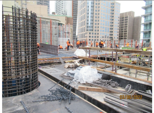
Martin Place North – Formwork for Level 8 (above the SSI level).
