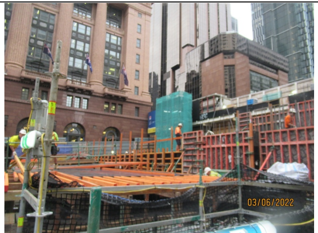
Martin Place South – FRP works ongoing
