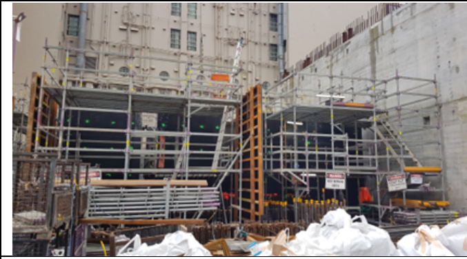
PSN south-eastern side: Central kicker wall FRP
