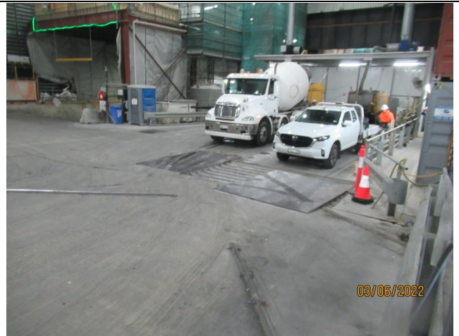
Bligh Street - Concrete Pumping
