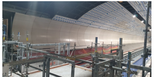
Station Cavern: GRC panel installation and cladding progressing.
