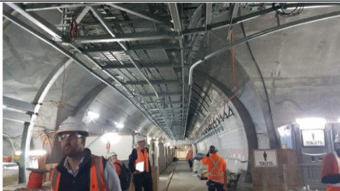
Southern Cavern: Services installation.
