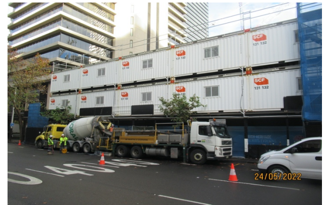
Victoria Cross South – Berry Street: Concrete pumping activities from Berry Street
