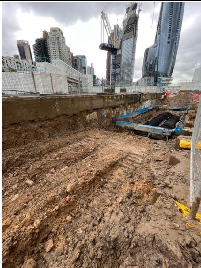
Pipe installation in the stormwater trunk main
