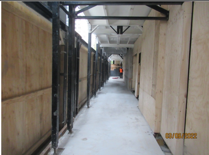
Martin Place North – new pedestrian footpath being constructed adjacent Elizabeth Street
