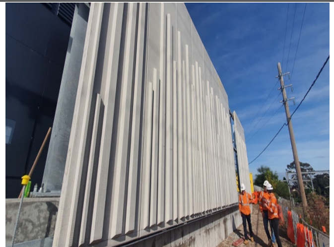
Campsie TSS: Façade installation commenced (6 concrete panels installed in WE45 possession).
