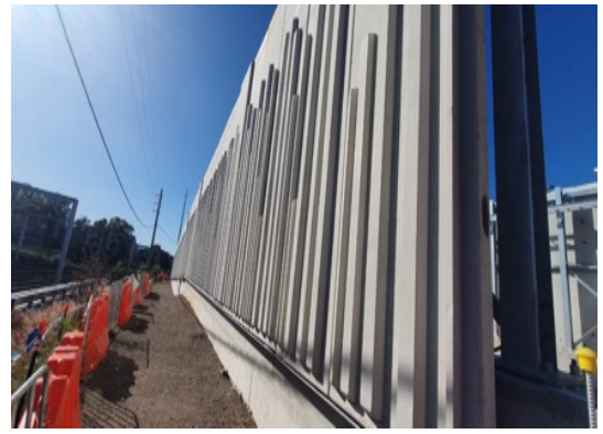
Campsie TSS - Concrete panels for façade installed
