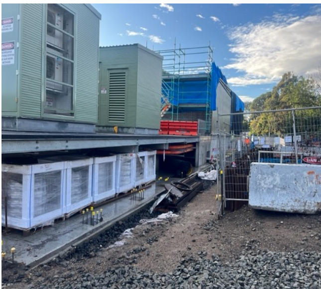
Marrickville MSB – Construction ongoing
