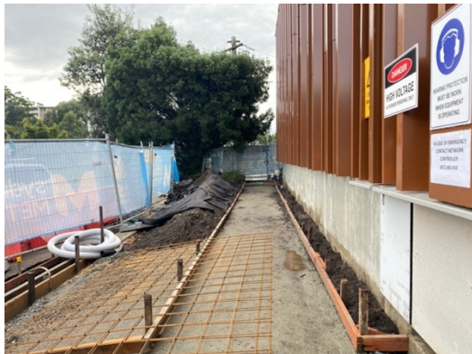
Artarmon TSS - Final landscaping underway.
