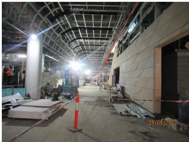
Fit Out in the North-South Concourse
