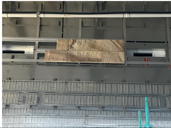
Sample of the platform wall cladding
