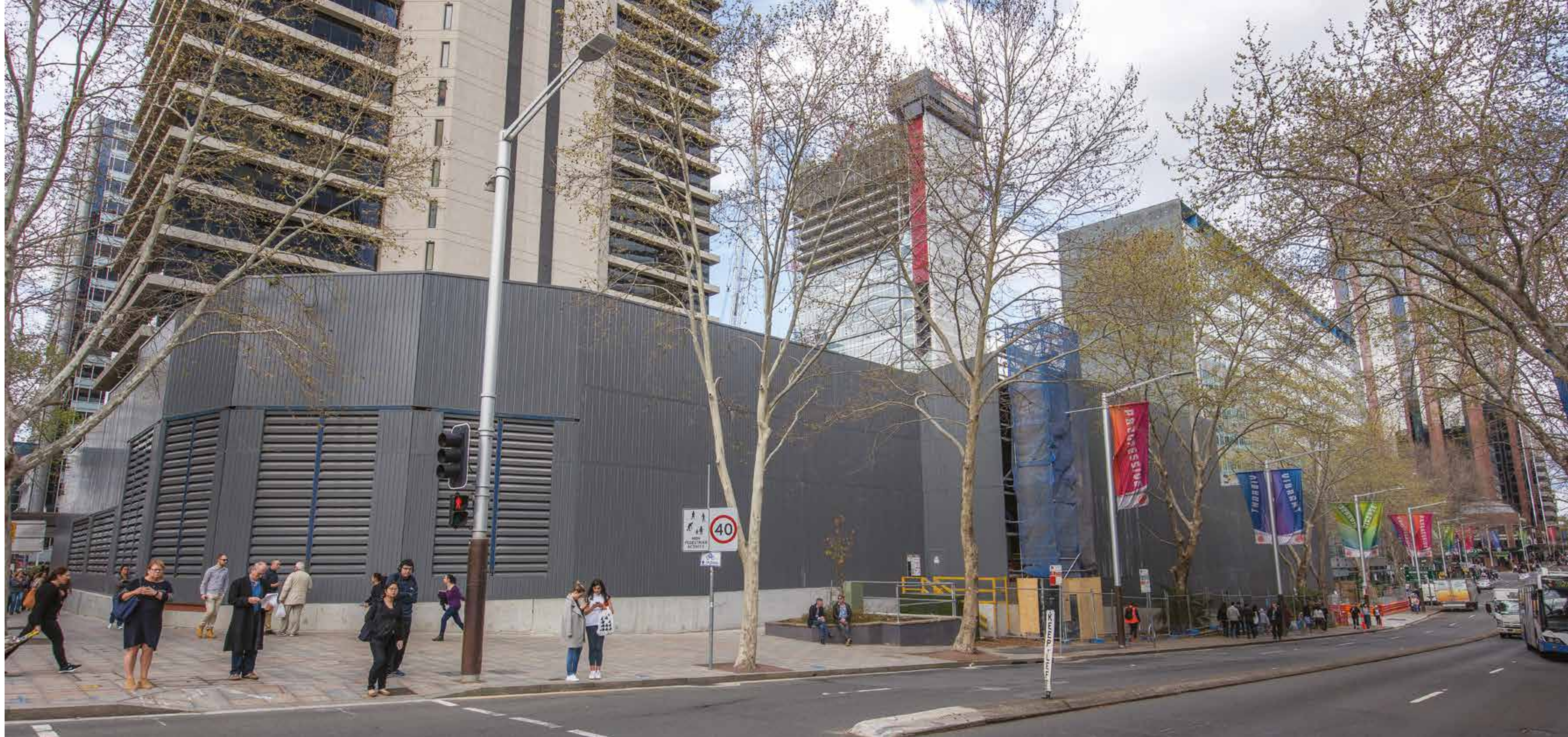
An acoustic shed used on the Sydney Metro City & Southwest project.
