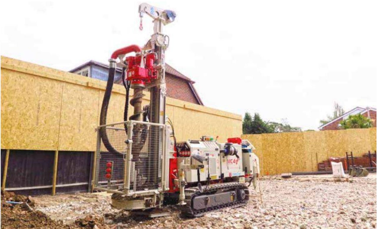
Figure 7 - Piling rig used for the works
