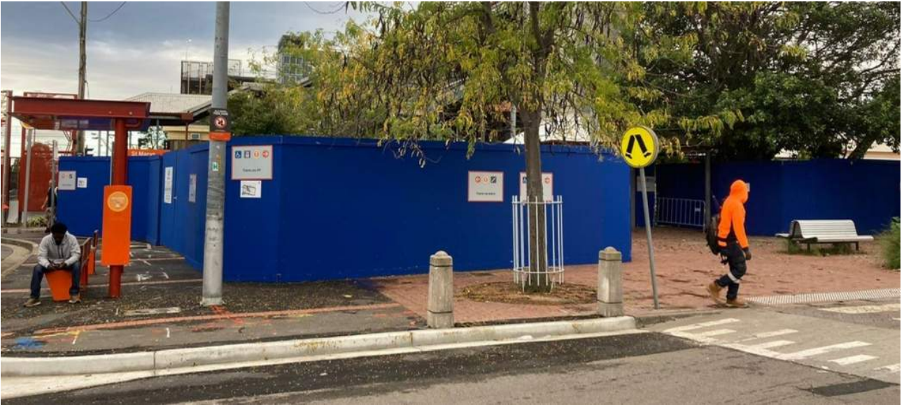
Figure 21 - Class A hoarding installed at St Marys Station
