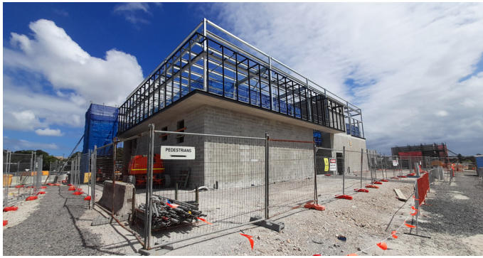
Fit-out of the administration building is now underway.
