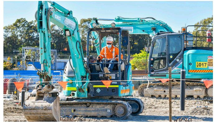
Extensive civil works were needed to install pipes and services.
