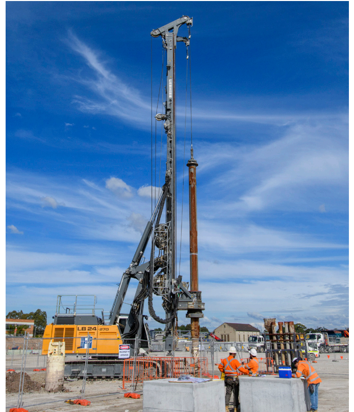
Deep piles were bored into the ground to support building foundations.
