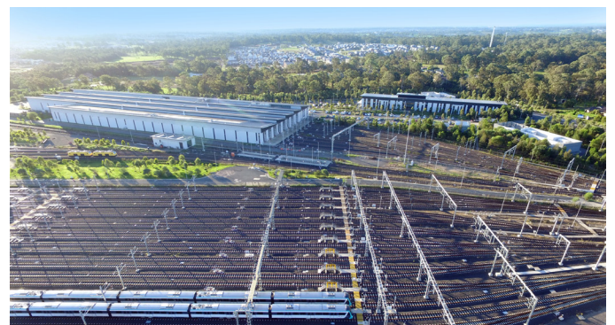
The expanded Sydney Metro Trains Facility North, at Rouse Hill.
