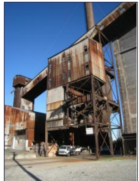
Figure 2: Coal handling plant from the north (Design 5:2011 Vol.2:19)
