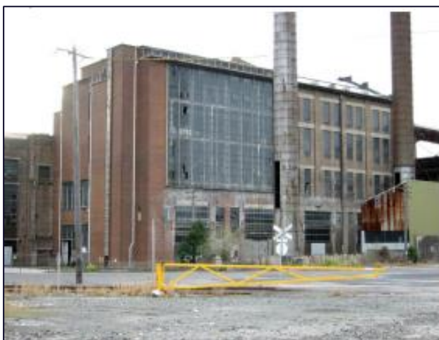
Photograph 1: Boiler House from the south east (Design 5:2011 Vol.2:19)
