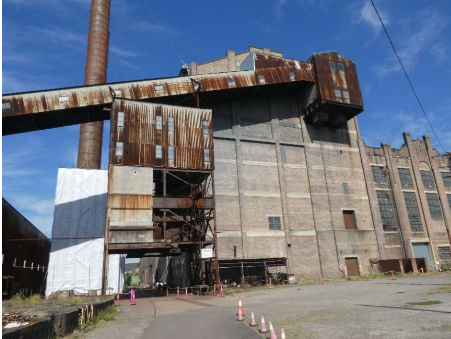
Figure 2: Northern side of the White Bay Power Station
