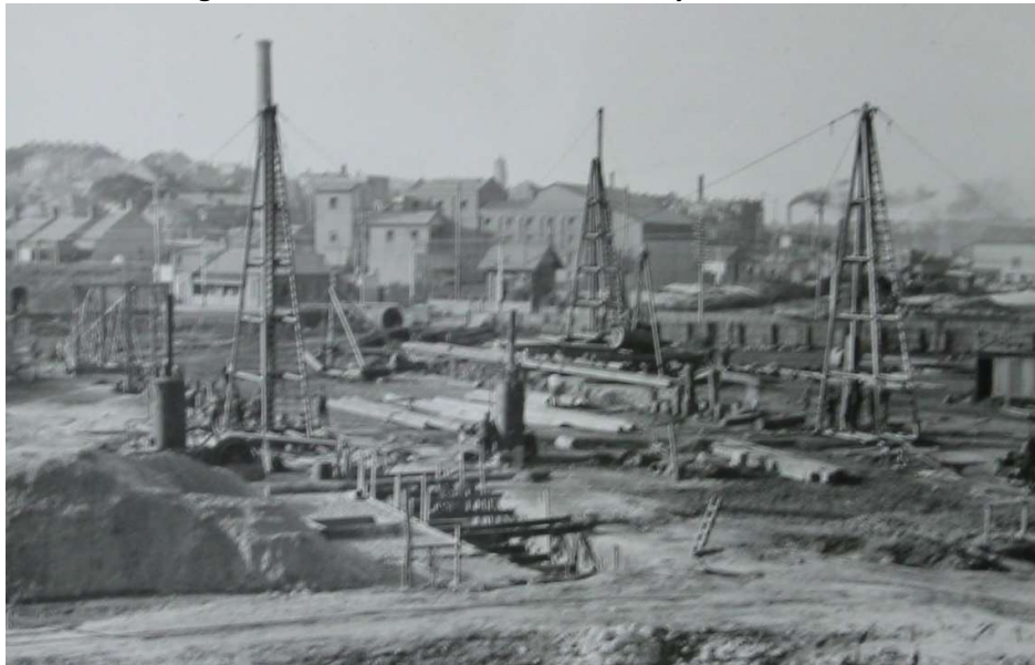
Figure 3: A 1912 photograph of piles being driven for the foundation of the White Bay Power Station
