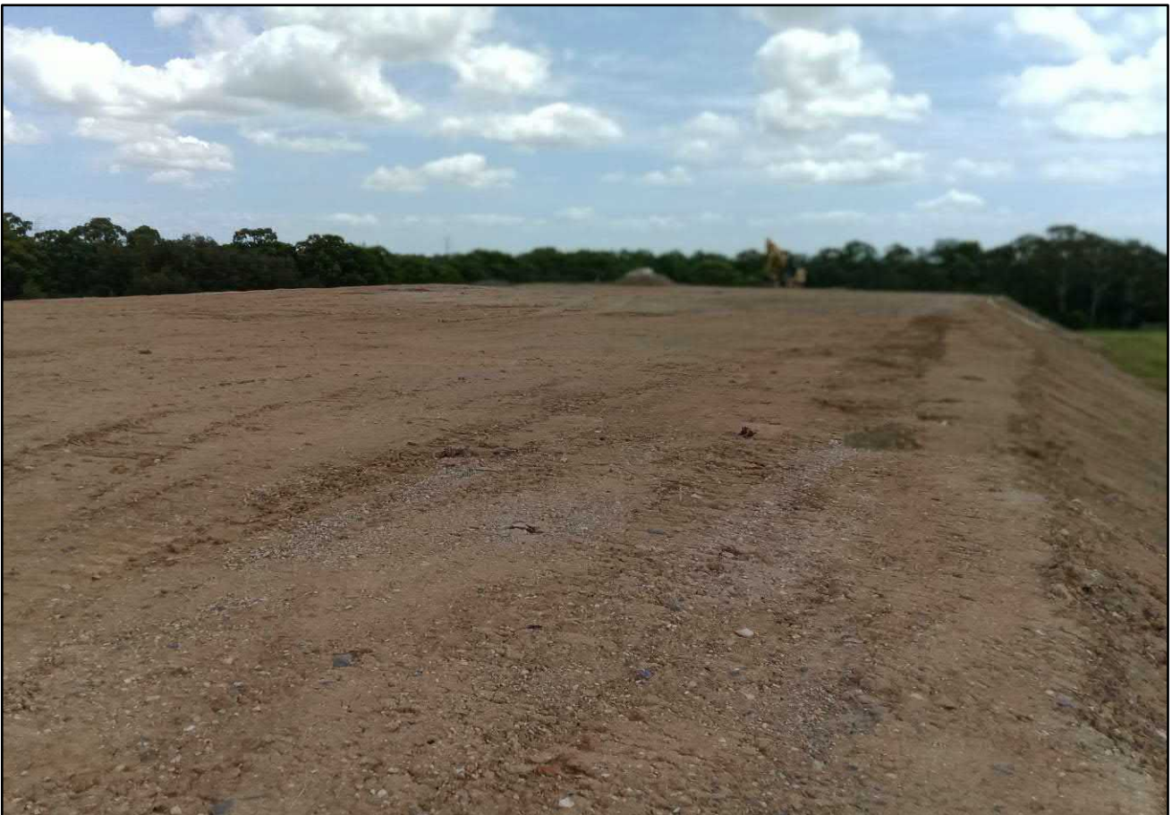
Photograph 10. Top of Area 7 Stockpile during the clearance inspection - facing east. Date: 14/02/2022.
