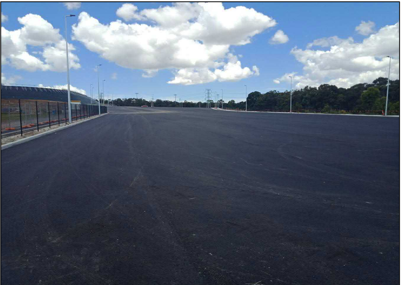
Photograph 4. Carpark D2 - facing east. Date: 02/12/2021.
