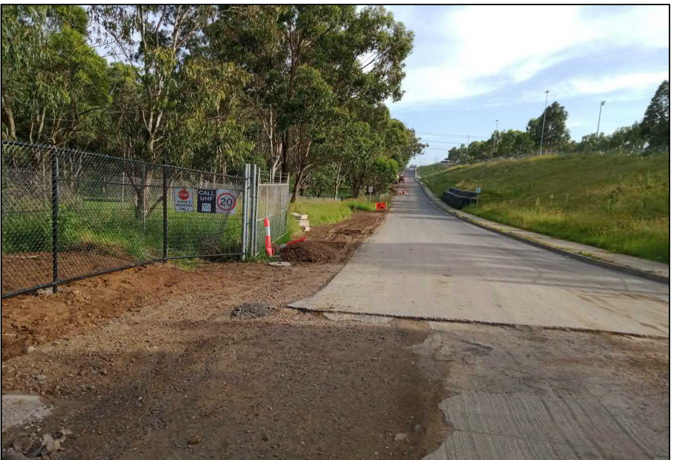
Photograph 8. Link Road during the clearance inspection - facing north. Date: 14/02/2022.
