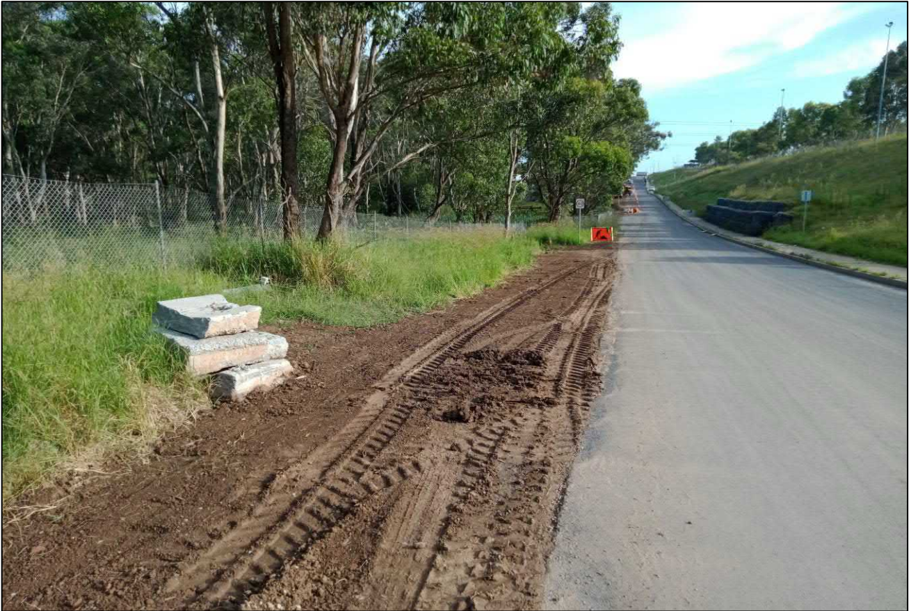
Photograph 9. Link Road during the clearance inspection - facing north. Date: 14/02/2022.
