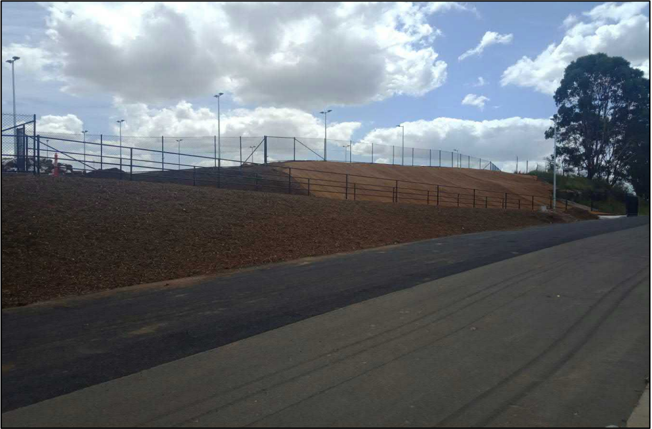
Photograph 5. Embankments of Carpark D1 - facing north-west. Date: 14/02/2021.
