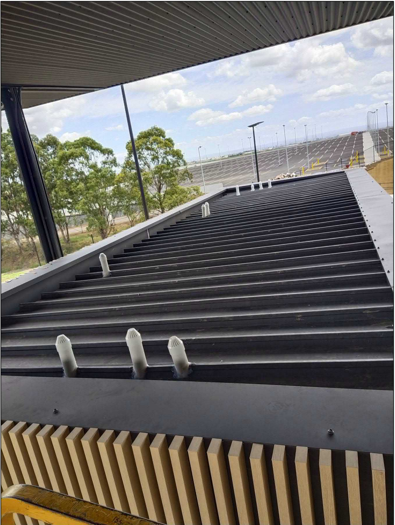
Photograph 13. The Northern Ticket Box retrofitted sub-floor vents. Date: 14/02/2022.
