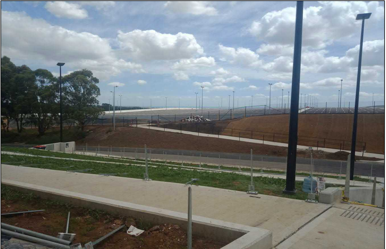
Photograph 3. Carpark D1 - facing west. Date: 14/02/2022.
