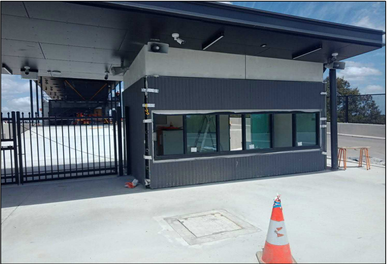
Photograph 7. Sydney Speedway Ticket Booth - facing south. Date: 15/02/2022.
