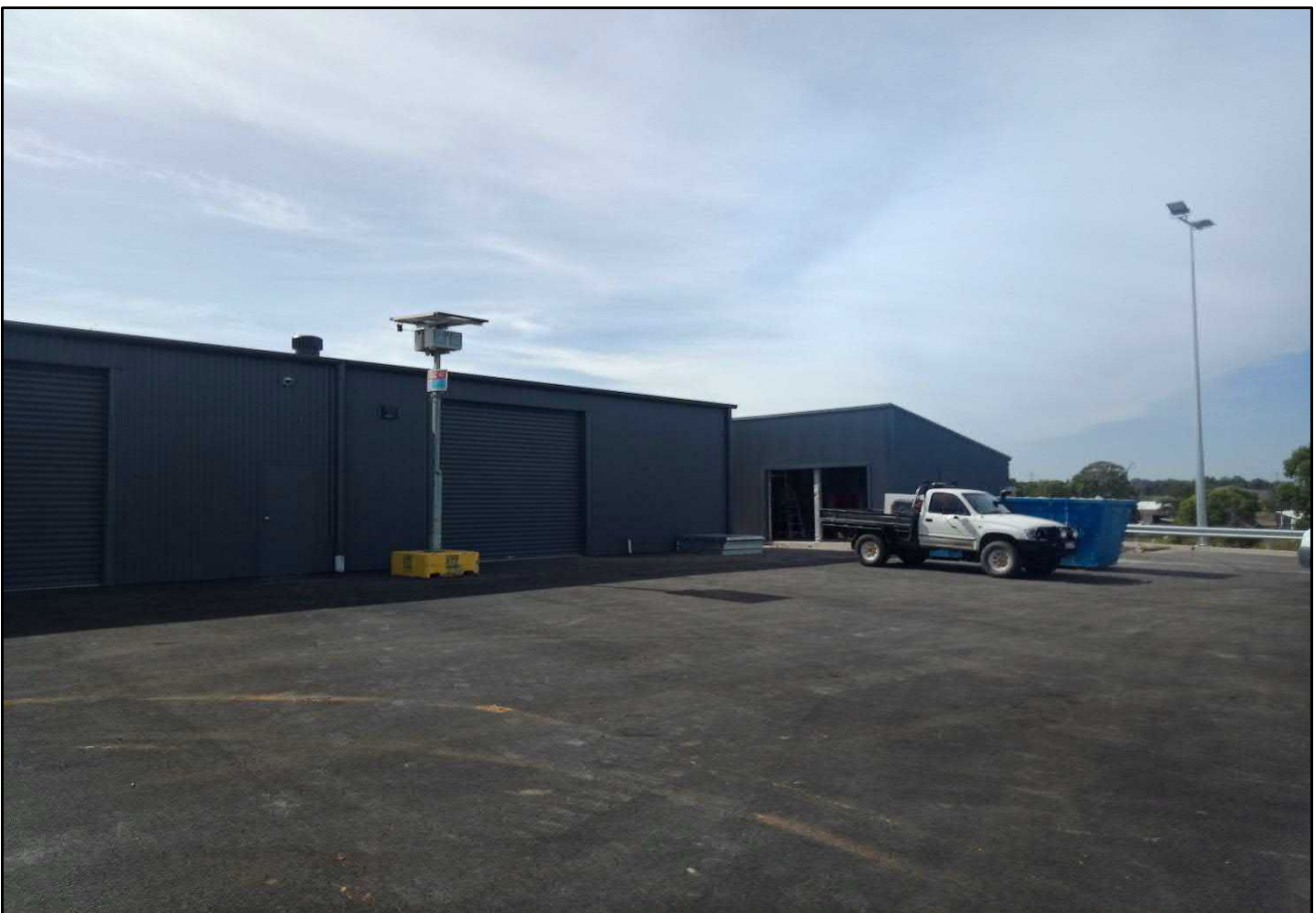
Photograph 12. Maintenance Shed and Fire Pump Room - facing south. Date: 14/02/2022.
