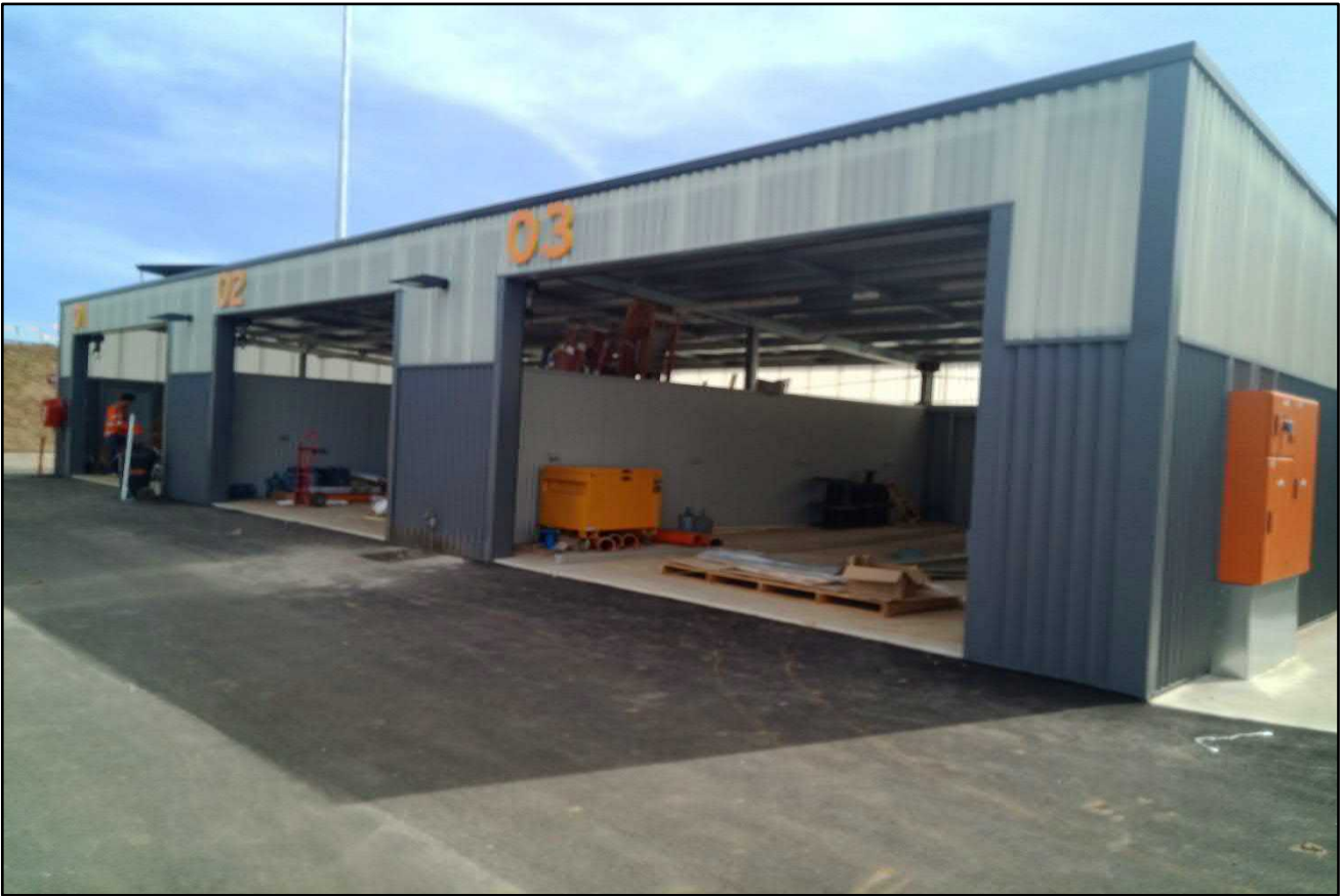
Photograph 9. Pit Garages 01, 02 and 03 - facing north Date: 14/02/2022.
