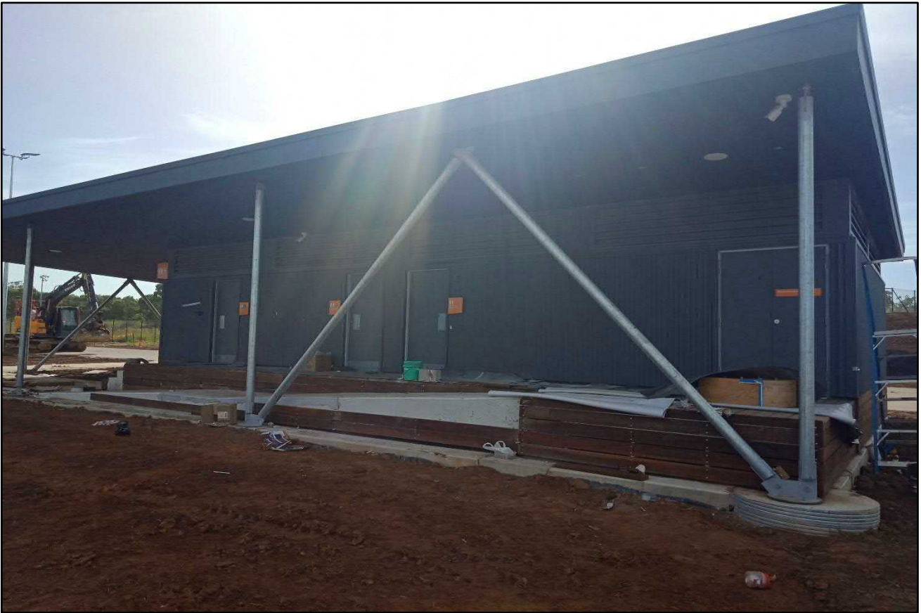
Photograph 11. Competitors Amenities Block - facing west. Date: 14/02/2022.
