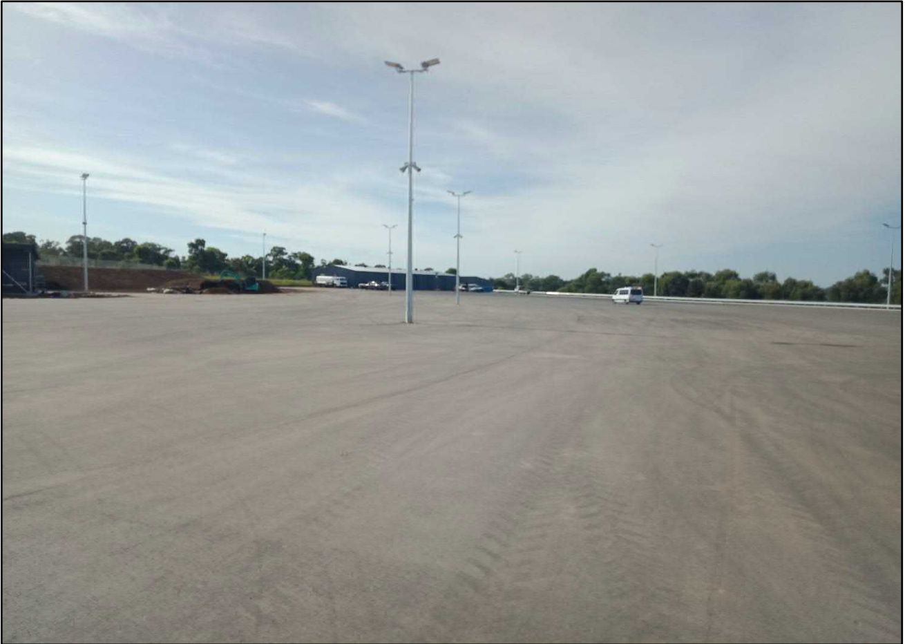
Photograph 13. Carpark B (area 6) - facing south. Date: 14/02/2022.
