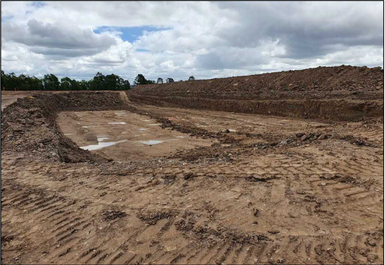
Photograph 1. Asbestos containment cell following bulk earthworks (as supplied by the client).
