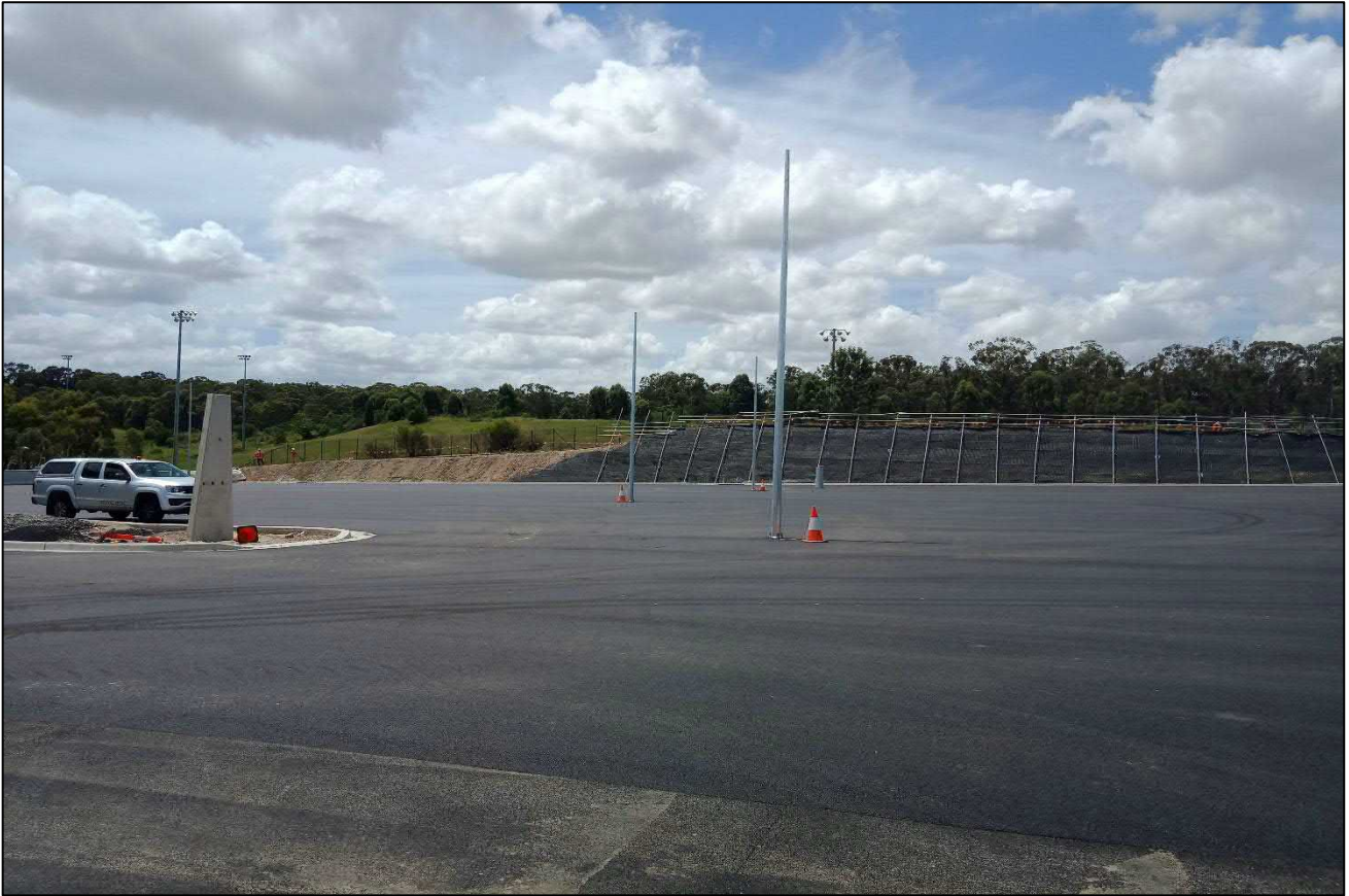
Photograph 5. South Carpark A (Area 4) - facing east. Date: 15/02/2022.
