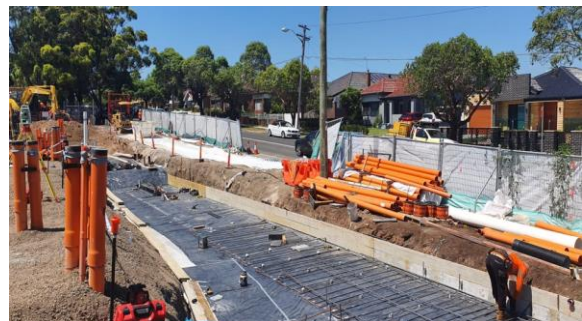
Punchbowl TSS – FRP works continuing.
