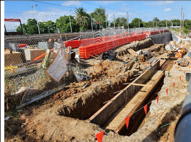
Lakemba MSB – stormwater / services connection works – 16/02/22
