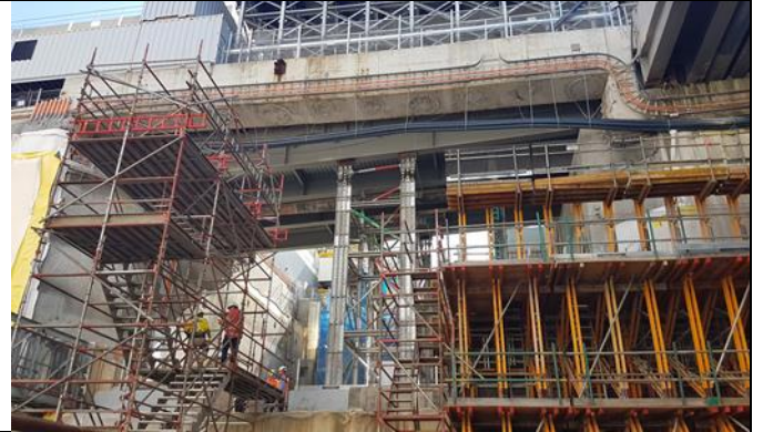
Site C – View east from station box level B3
