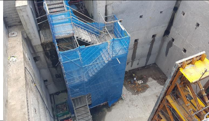
Site C – Area being prepared for detailed excavation
