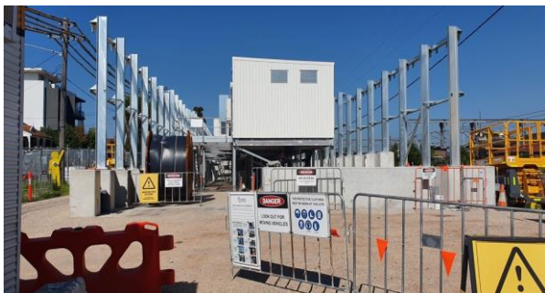
Campsie TSS – Steelwork in place for TSS facade installation.
