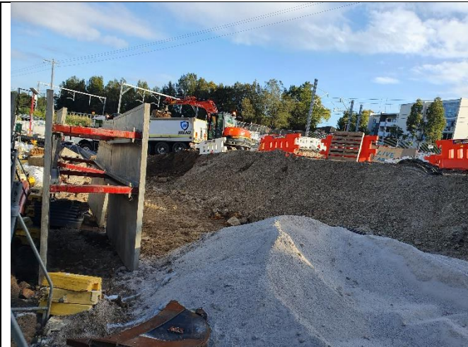
Canterbury MSB excavations – 16/02/22
