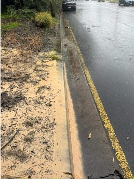
Sediment laden runoff identified under the Stacey Street Bridge after a large rainfall event (an incident was raised)
