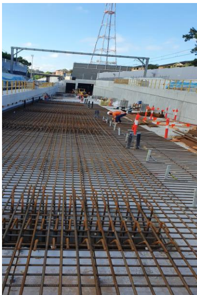
Northern Connection: Blinding completed and steelwork in progress for track
