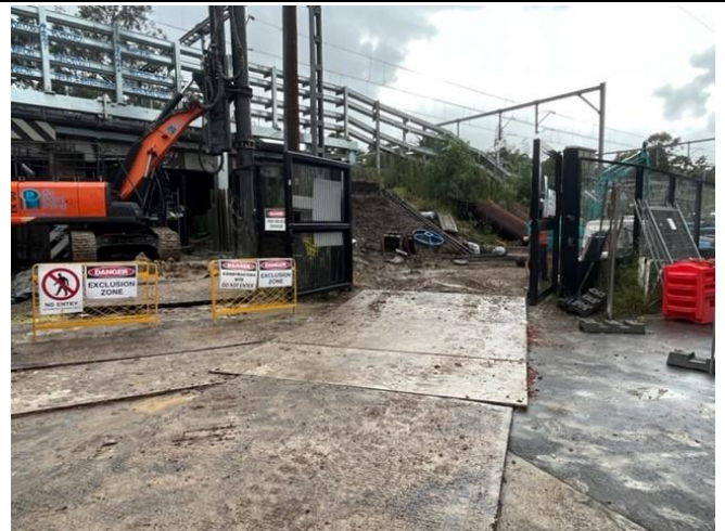
Piling for crash beams at Wairoa Street, Campsie
