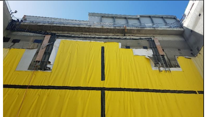
South tunnel portal ongoing waterproofing
