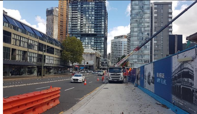
Pacific highway logistics lane in operation -view north
