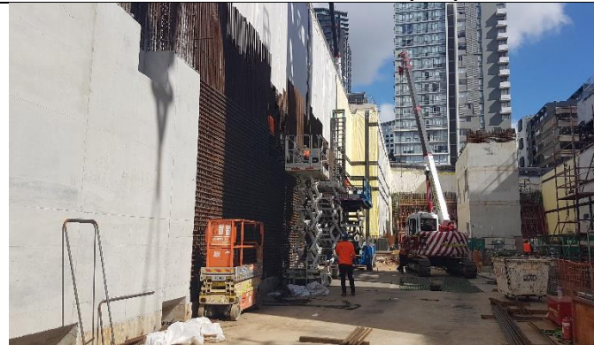
Site A view North with steel fixing & jump form removed
