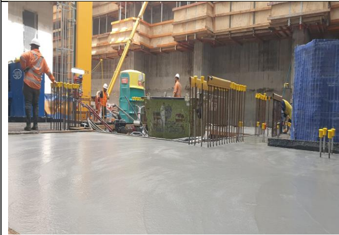
Victoria Cross North - Level B8 (Station) - Concrete pour for structural floor.
