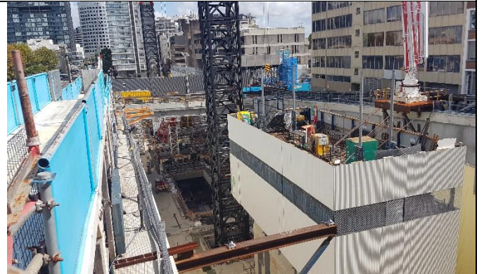
Site B - Jumpform at Level B1 looking North
