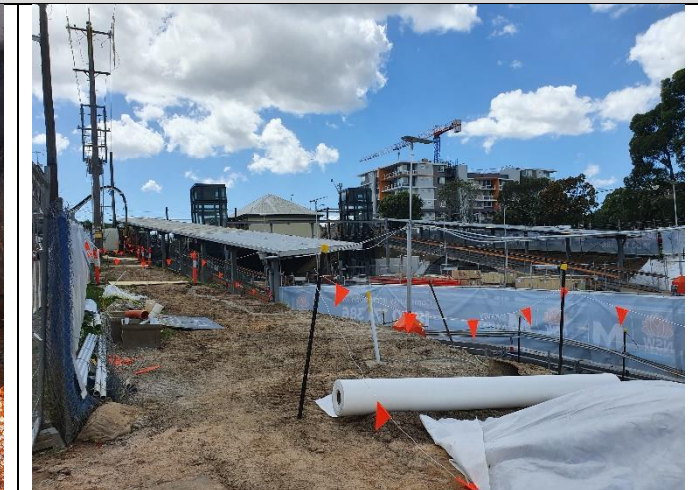
Wiley Park lift pits installed
