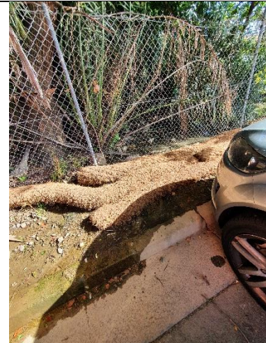
Lakemba The Boulevard Carpark swale exit – 16/02/22
