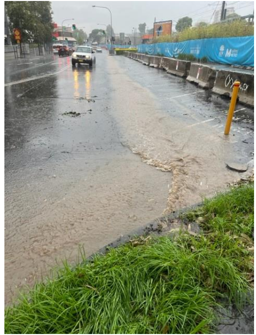
Sediment laden runoff identified under the Stacey Street Bridge after a large rainfall event (an incident was raised)
