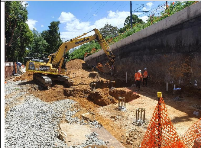
Hurlstone Park MSB excavation for stormwater connection
