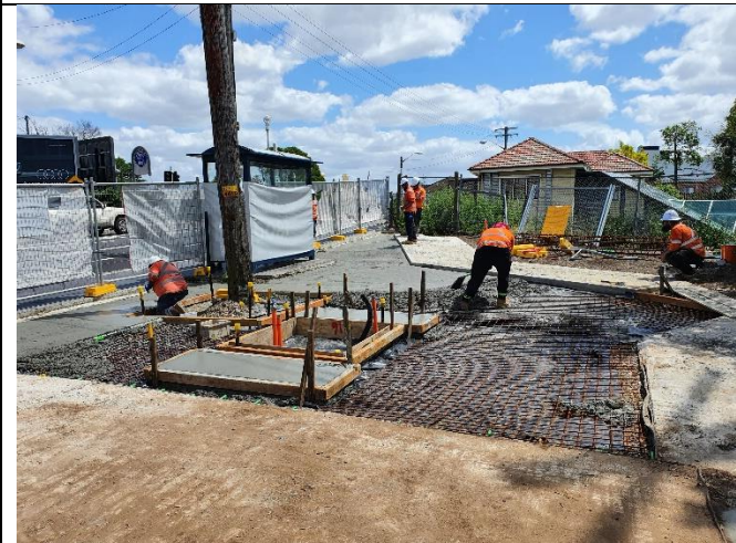
Belmore plaza concreting works
