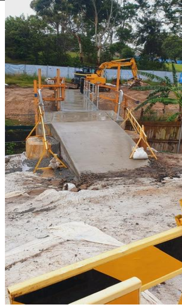
Pat O'Connor Reserve – Cable bridge nearing completion.
