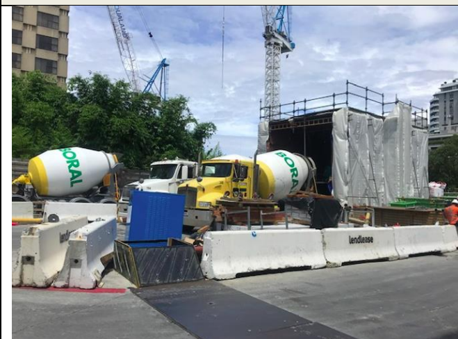
VCN - North Yard Area: Concrete truck deliveries in North Yard
