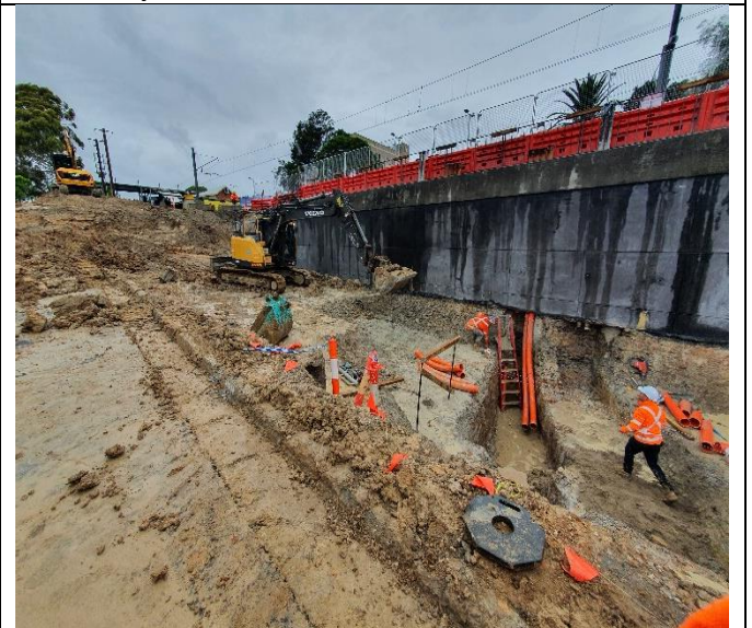
Lakemba MSB – stormwater connection excavation 19/01/22
