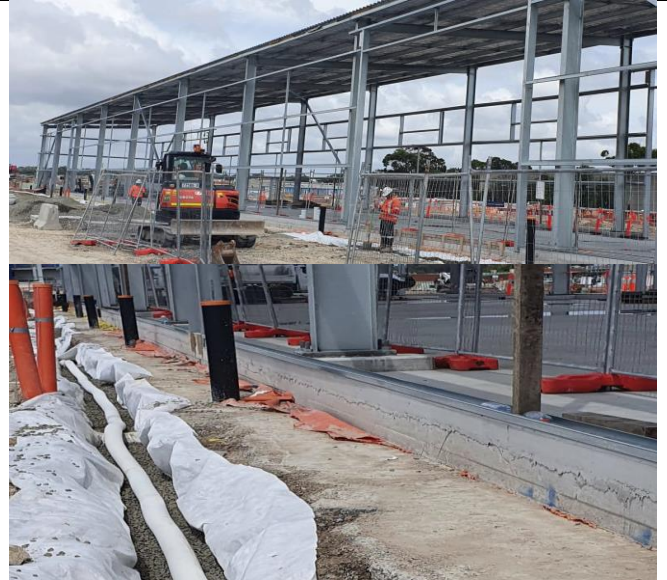
SMTF S - Covered Shed – sub-soil placement / drainage works underway
