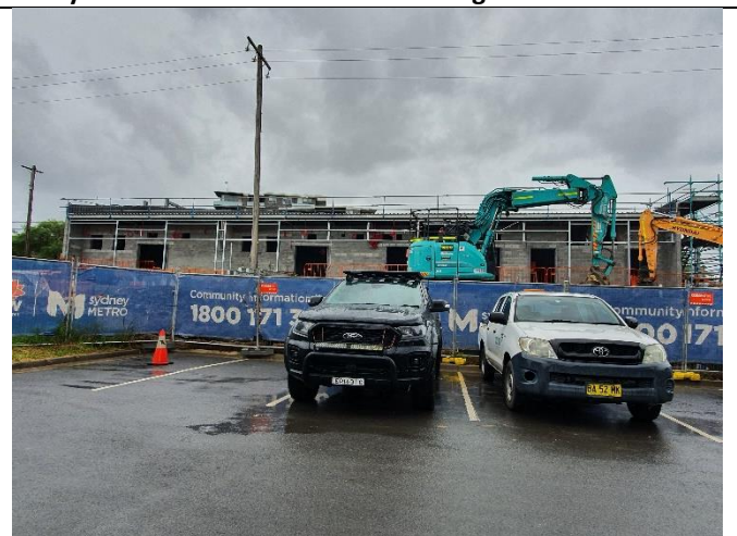
Punchbowl MSB construction
