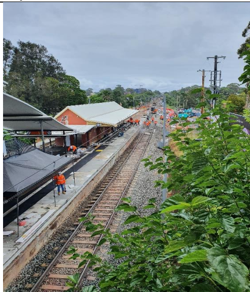
Lakemba Station – tiling works 05/01/22
