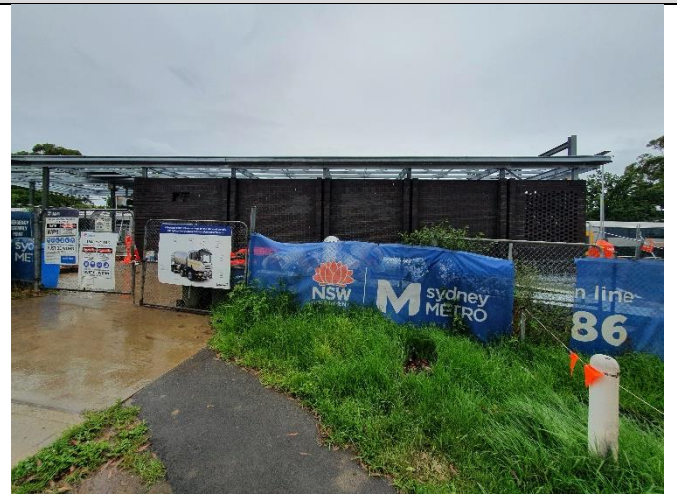
Wiley Park construction station awning
