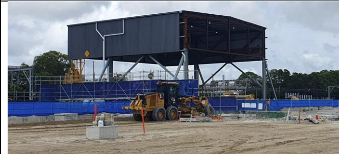
SMTF S - Stabling Yard – grading works in progress.
