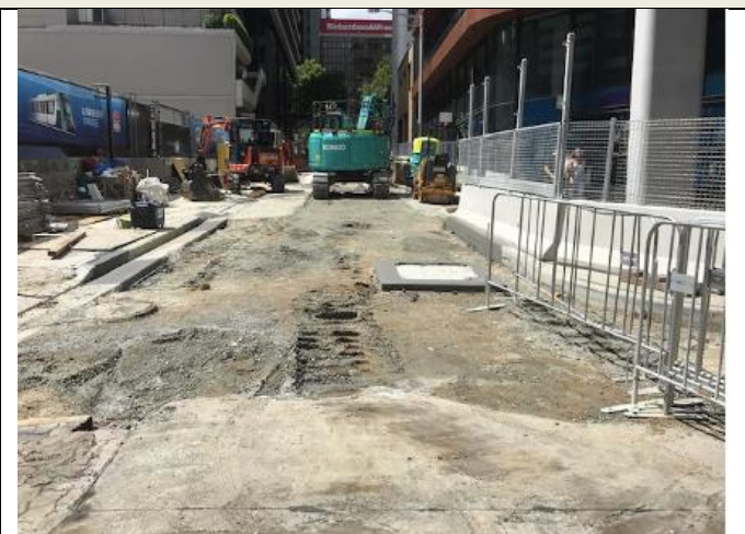
Denison Street - Stormwater works – Stage 3 area: backfilling and compaction works underway
