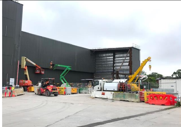
Northern Hub - CDS Yard: Gantry shed (south- eastern side) modification progressing.
