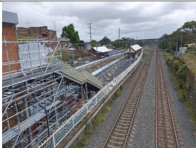
Hurlstone Park platform works
