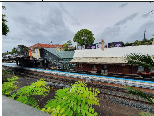
Belmore platform works
