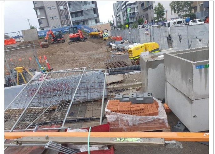
Canterbury MSB excavations 19/01/22
