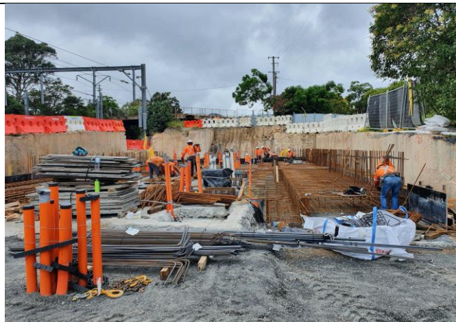
Canterbury TSS – CSR and FRP works continuing.
