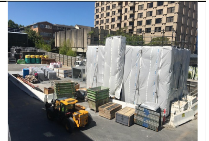
Over-Track Exhaust structure completed
