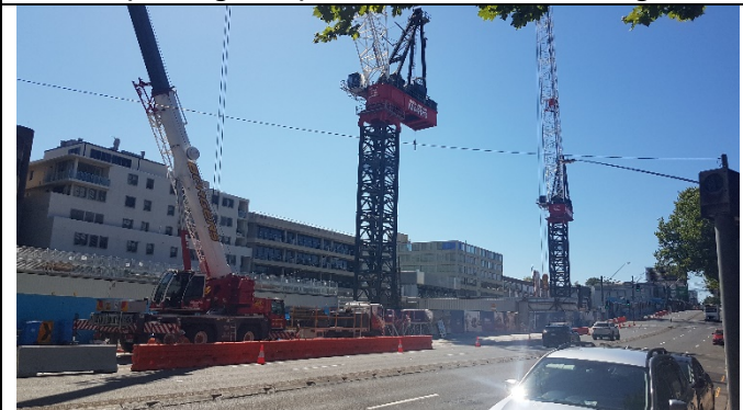
Pacific highway logistics lane in operation -view east
