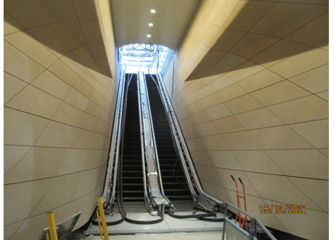
Fit out and façade placement for escalators to Platforms 16 and 17
