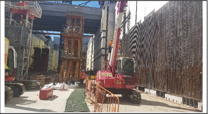
Perimeter wall steel fixing
