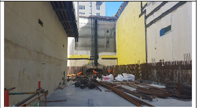
North tunnel portal ongoing waterproofing
