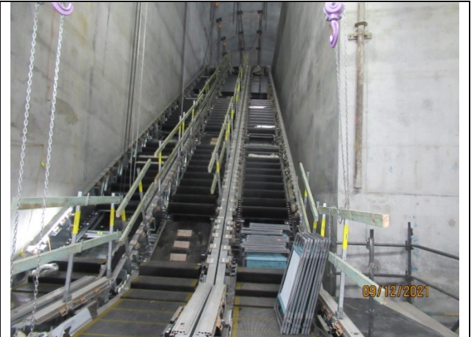
Escalators installed for access between ESR and Metro Station.
