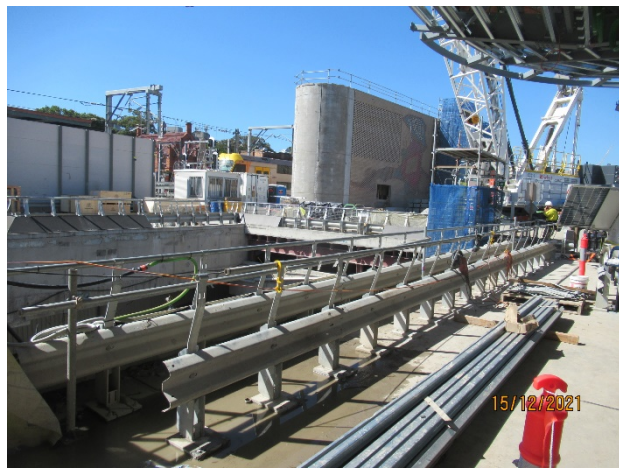
General works in the Metro Box area
