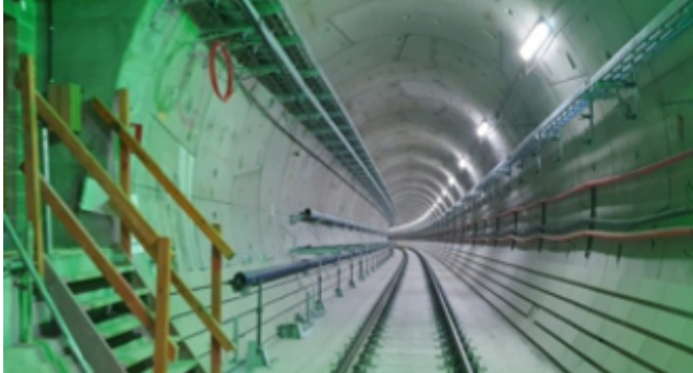
Tunnels - installation of mesh on walkway frame and installation of noise panels (for operational phase) on both walls continuing.
