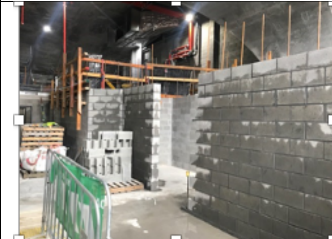
VCS South Back of House Area: Blockwork continuing.
