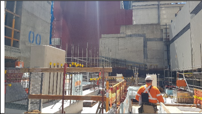
PSS -Various steel fixing and formwork at B01M level
