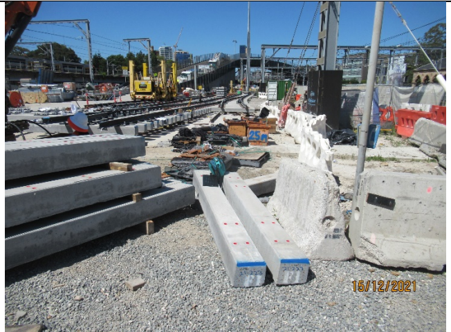
Assembly of turnout for tracks on new platforms
