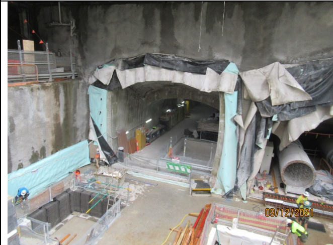
Martin Place South – Pedestrian Tunnel
