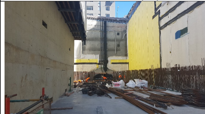
Level B3 (above girders) view North with steel fixing
