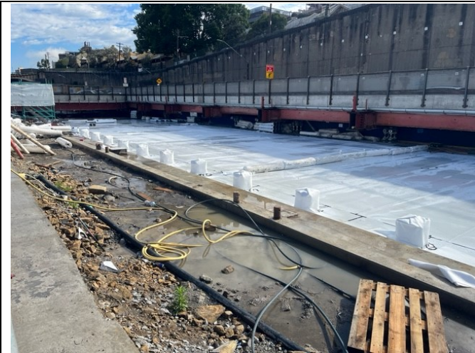
Waterproofing of the station box roof
