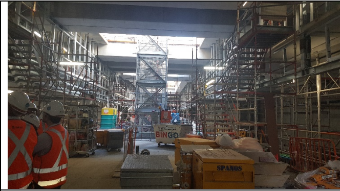
General view of station to north, from top of platform
