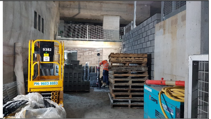
PSS B1 interior construction, including blockwork
