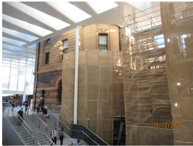
Ongoing works in the Northern Concourse
