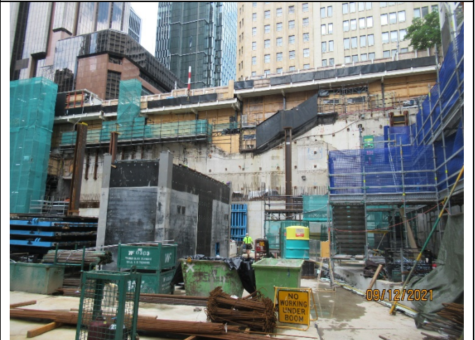
Martin Place South – ongoing FRP works
