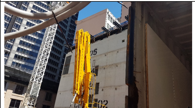
Pitt St North (PSN) Western core structure to Level 5
