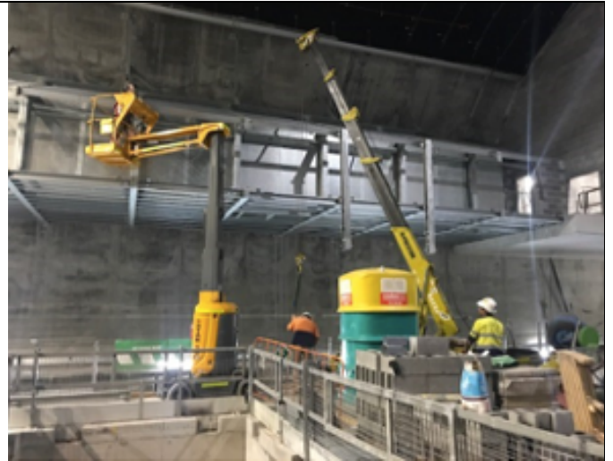
Eastern Cavern: Structural support installation work on OTE ventilation modules underway.
