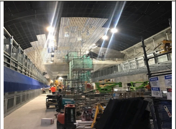
Cavern: GRC panel installation continuing on roof of cavern
