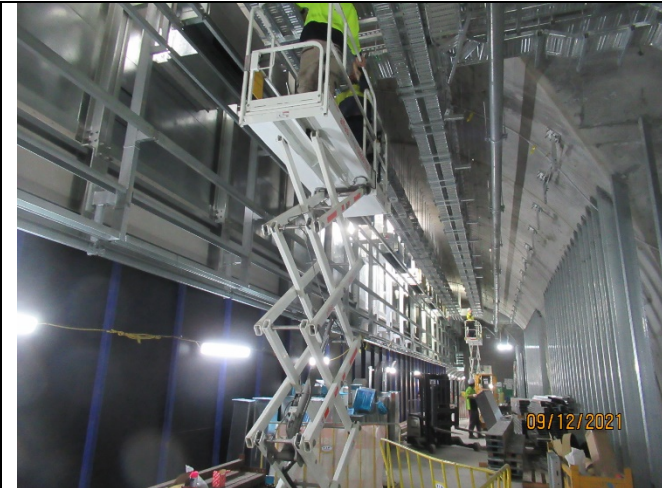
Platform Caverns – Fit out
