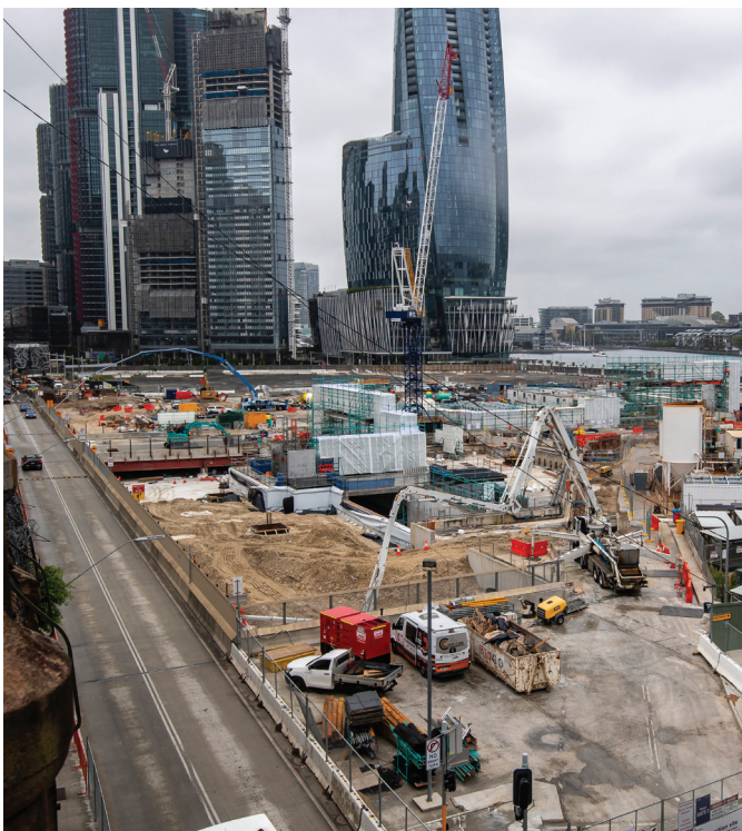
Removing the girders under Hickson Road
