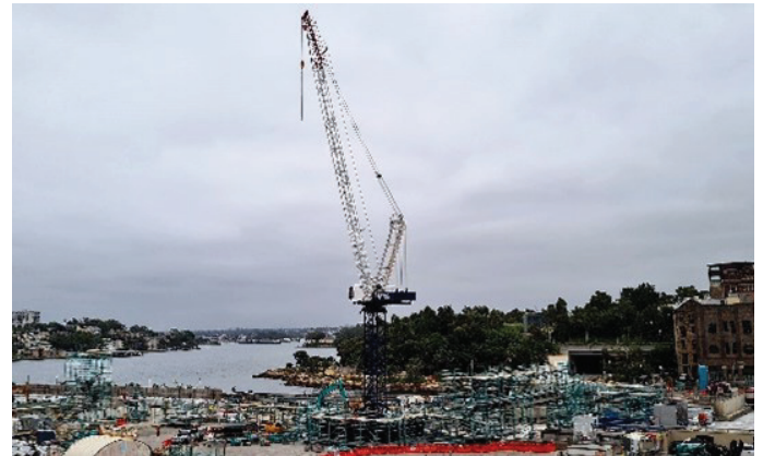
New tower crane for Barangaroo Station works
