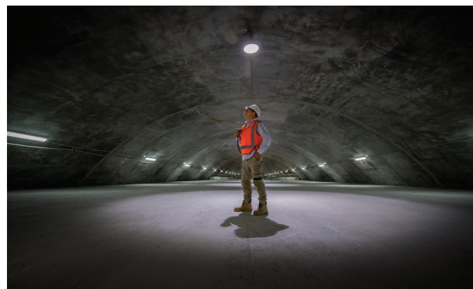
Site foreman Michael Richens admires the station box
