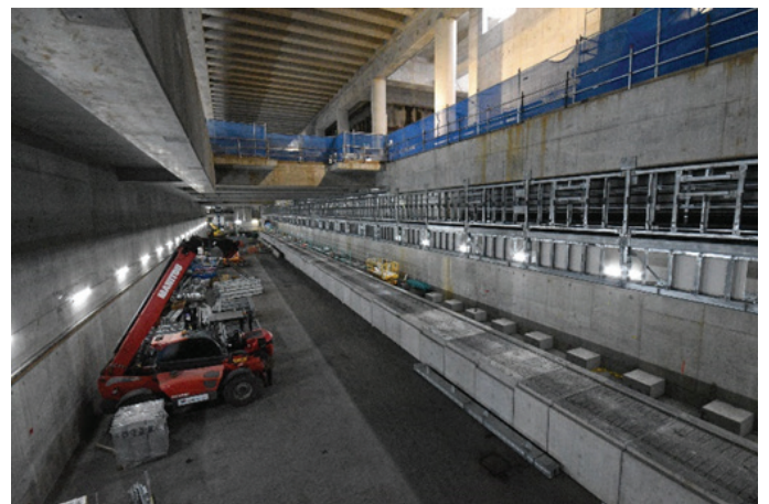
Installing overhead ventilation and platforms inside the station box
