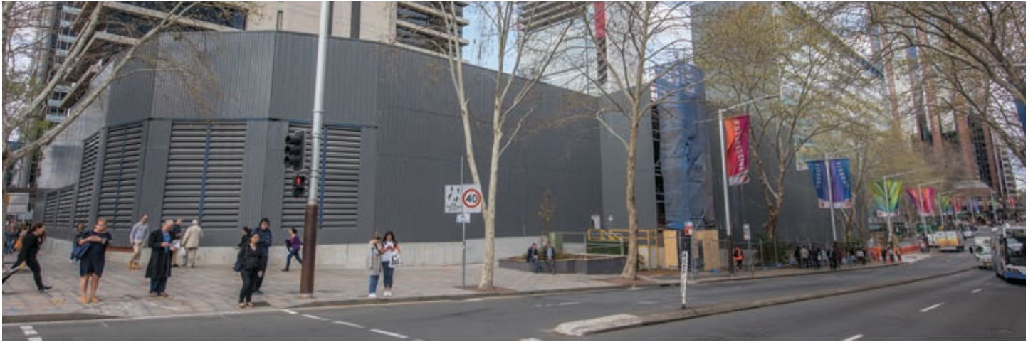
An acoustic shed at the Victoria Cross Station site in North Sydney.
