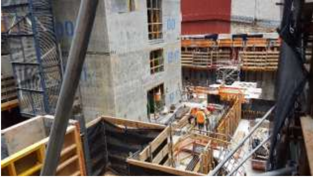
Various steel fixing and formwork at B01 and B01M level
