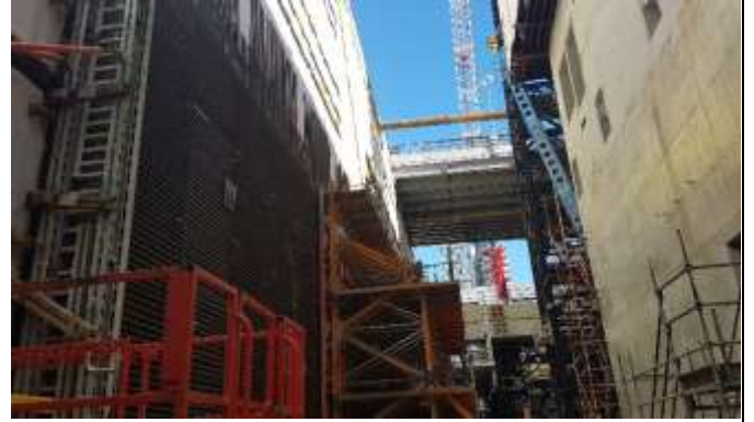
Ongoing wall steel fixing and shutter placement with Hume St above
