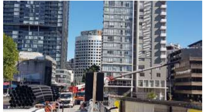
View North of delivery lane on Pacific Hwy (Site A)
