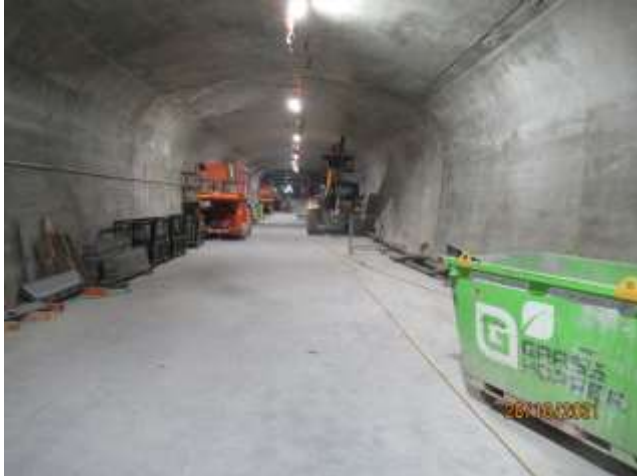
Pedestrian tunnel between MPS and MPN
