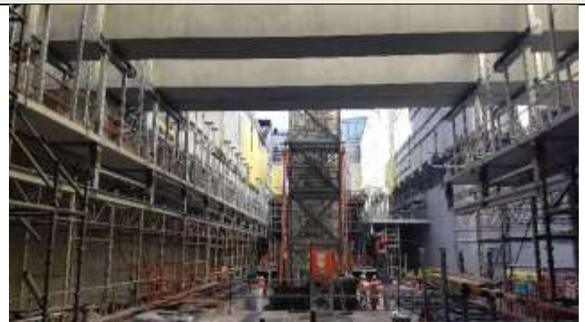
Precast girders in place view south
