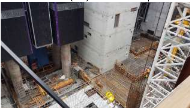
PSN eastern side: FRP at level B03
