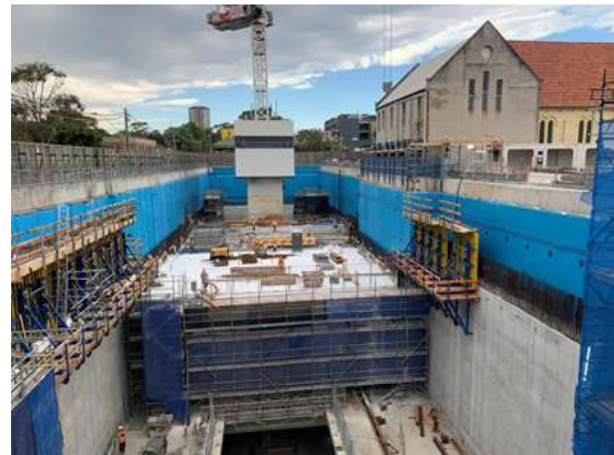
Steelwork, formwork and concrete pours ongoing at B2/B3 Levels
