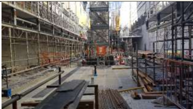
Platform and over track exhaust (OTE) structures to sides
