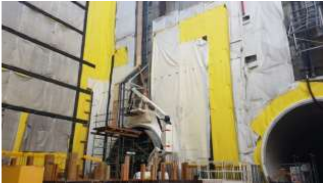
Waterproofing at southern tunnel portal
