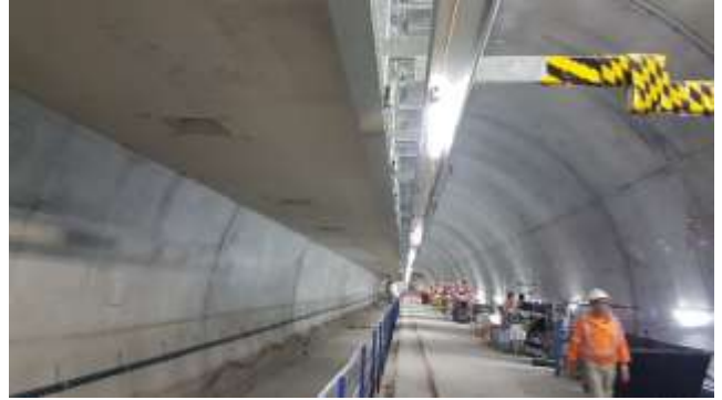
Western cavern track slab and platform with OTE on left
