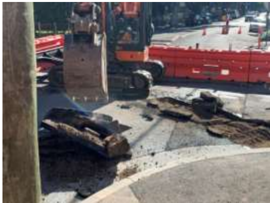
Trench alignment saw-cut and peeled up by excavator.
