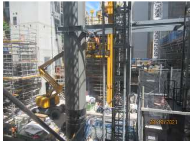
Columns and jump form above ground level at MPN.
