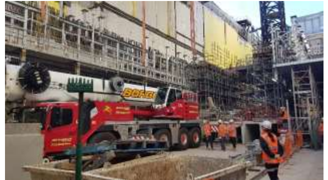
Construction of platform and OTE structure
