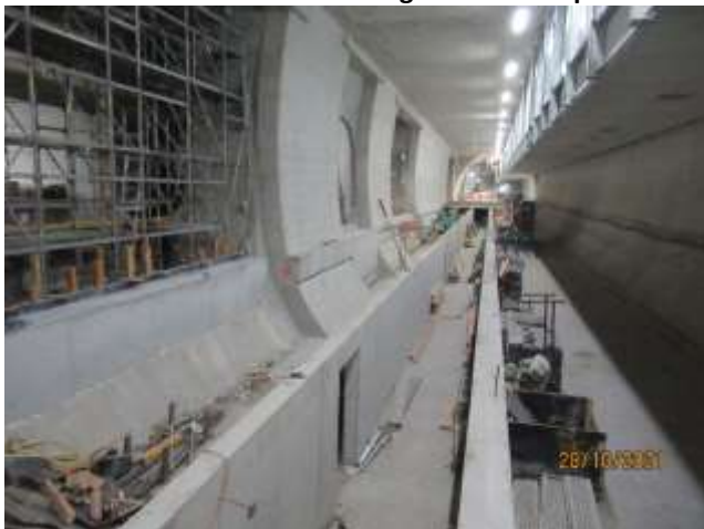
Platform construction in station cavern
