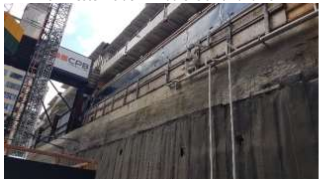
PSN Park St capping beam below hoarding, at street level
