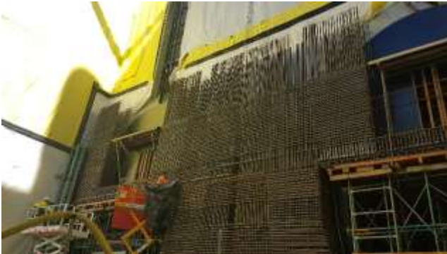
North tunnel portal steel fixing for perimeter wall
