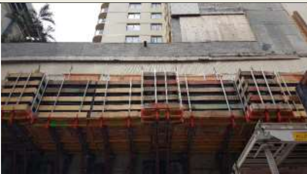
Pitt St South (PSS) Perimeter wall FRP to ground level
