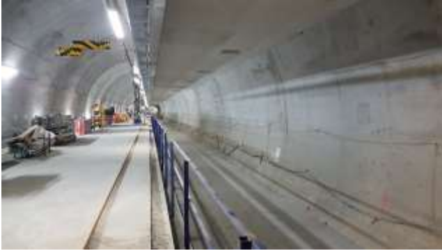
Eastern cavern track slab and platform
