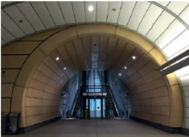
Macquarie Park Station. Services are concealed and integrated within the cavern structure, enabling the clean expression of the cavern form. Architect: Hassell Source: Cox Richardson
