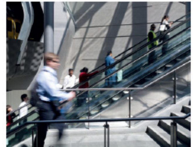
Chatswood Station, Sydney, NSW. Example of handrail and stanchion Architect: CoxDesignInc.
