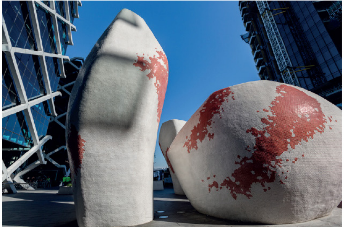
Sculptural plant extraction vents at One Shelley Street, Sydney. Artist: Anton James Source: TfNSW
