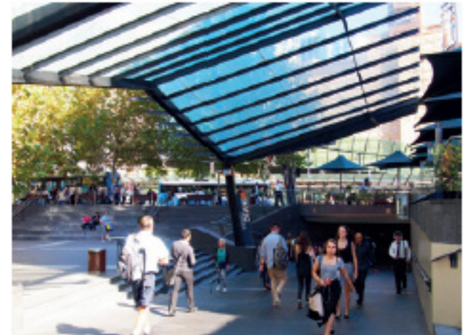
Design paths and ramps for access for all. All modal connections must be located in convenient, safe, well-lit areas with good natural surveillance. Source: AECOM.
