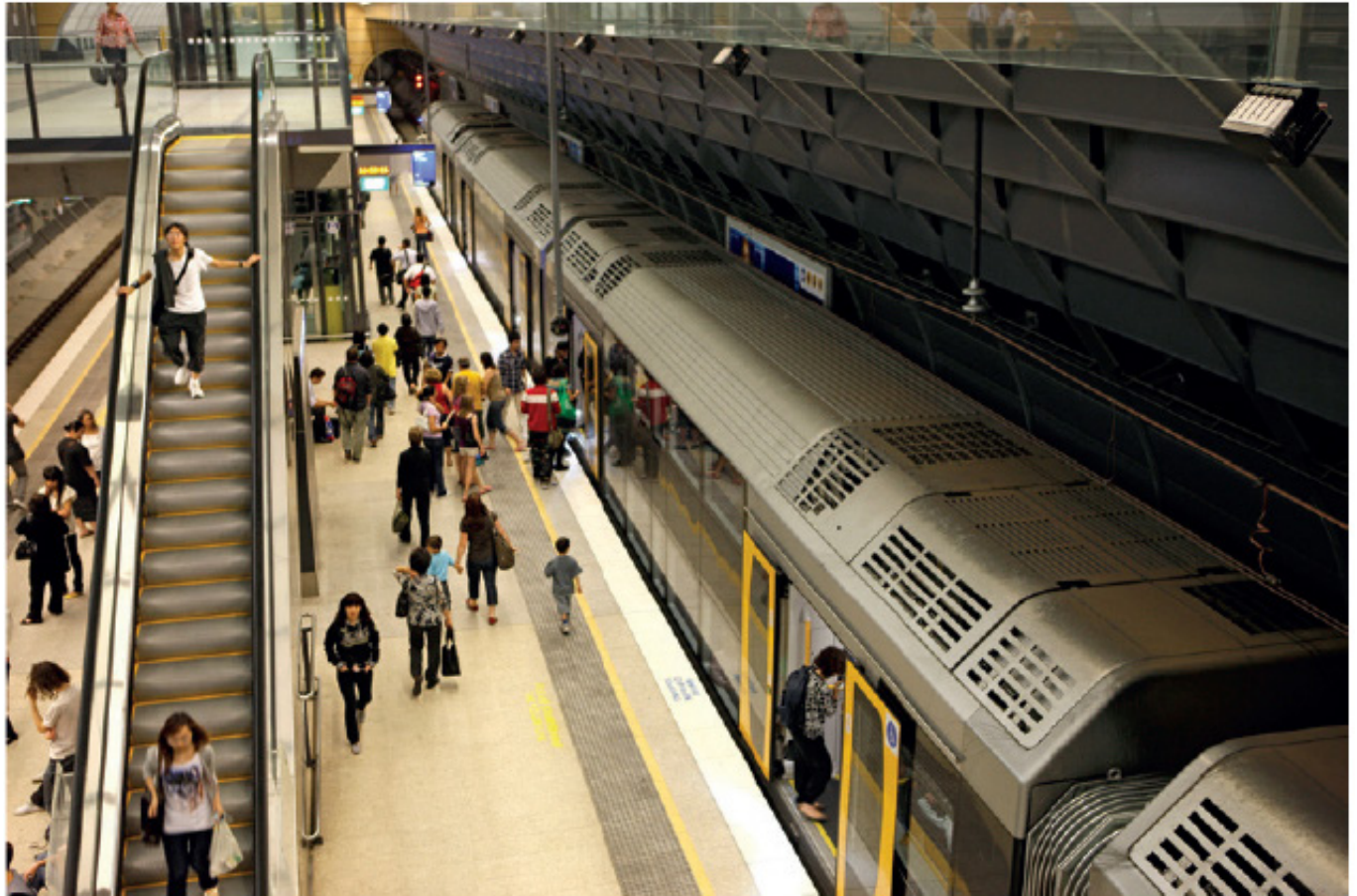
Macquarie Park Station. Clear sightlines and uncluttered spaces provide a safe and welcoming customer environment. Source: TfNSW
