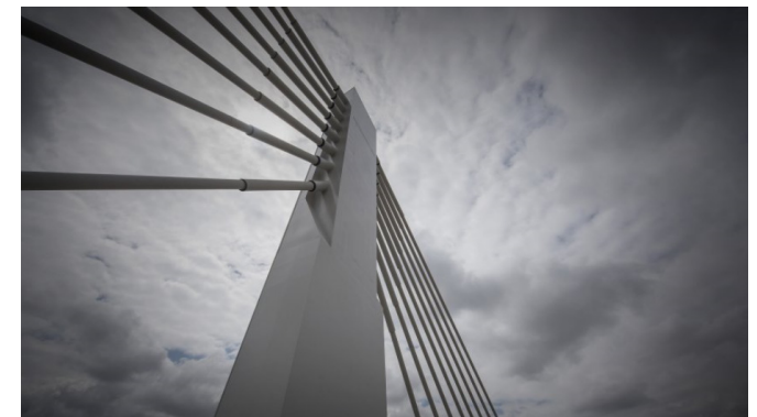
Skytrain bridge, Sydney Metro Northwest. Sydney Metro
