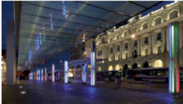
Britomart Transport Centre, Auckland. Lighting is designed to provide a safe, legible and comfortable environment for customers and users. Architects: Mario Madayag & Jasmax Source: Opus
