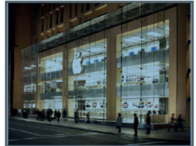
Glazed facades enable transparency and legibility. Architect: The Buchan Group Source: Apple
