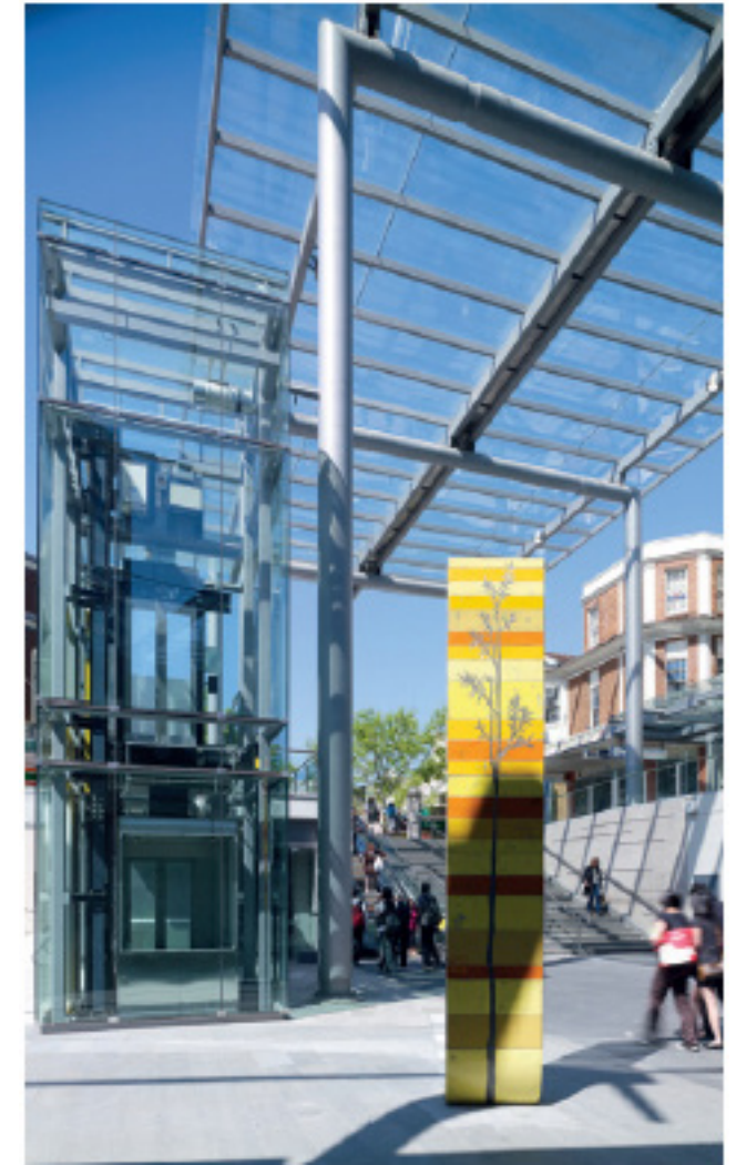
Chatswood Transport Interchange, NSW. Good example of a glazed lift and shaft Architect: CoxDesignInc. Source: Cox Richardson
