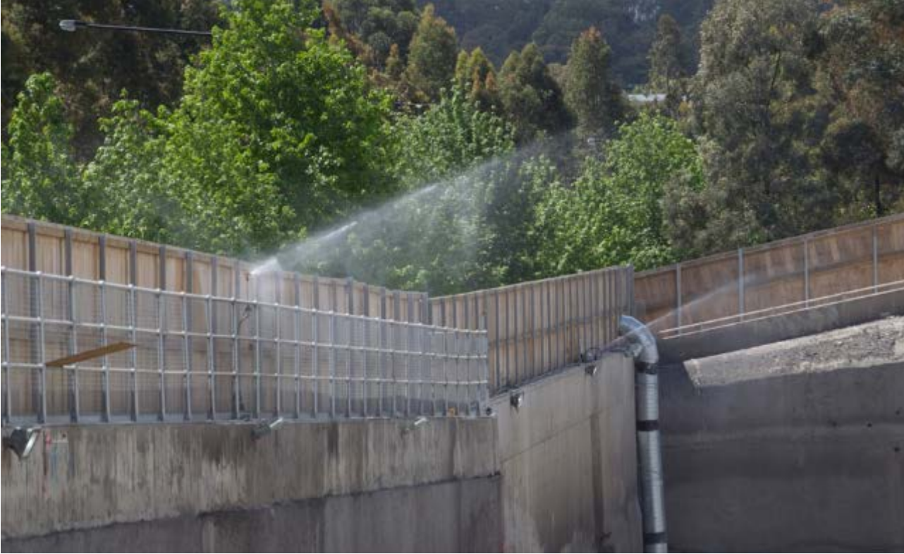
Figure 11 - Dust Mitigation at Norwest Station Site
