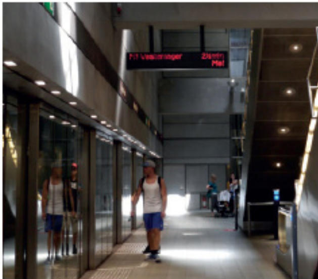
Copenhagen Metro, Denmark. Good example of full height PSD Architect: KHRAS Architects Source: Cox Richardson
