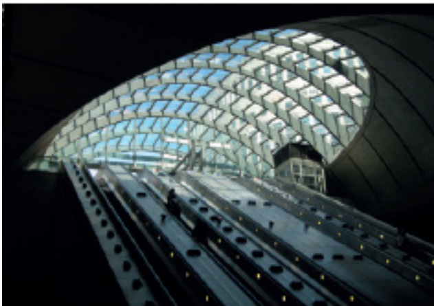
Canary Wharf Station, London. Natural light over entries and VT enhances wayfinding and creates a welcoming station environment. Architect: Foster + Partners Source: Cox Richardson
