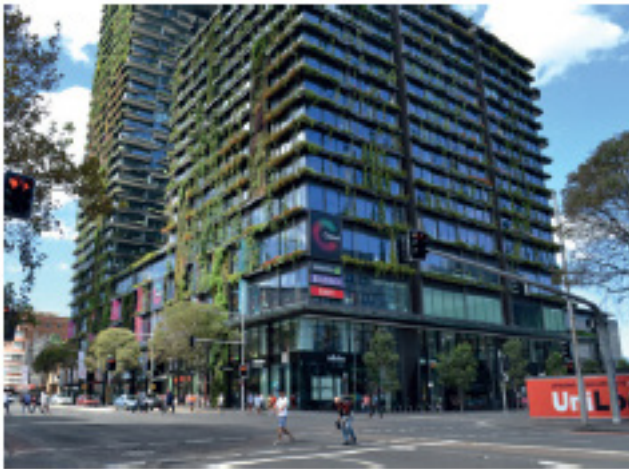
Central Park, Sydney. Landscaped facade treatment helps cool the microclimate. Architect: Jean Nouvel Source: Cox Richardson
