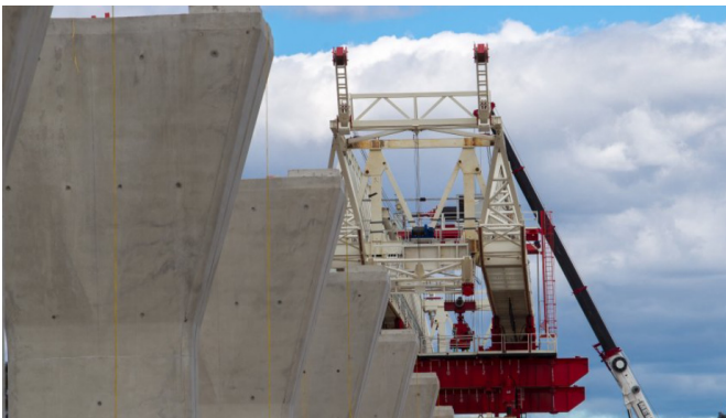
Viaduct piers, Sydney Metro Northwest. Sydney Metro
