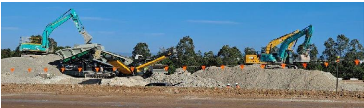
Screening of imported VENM tunnelling material.
