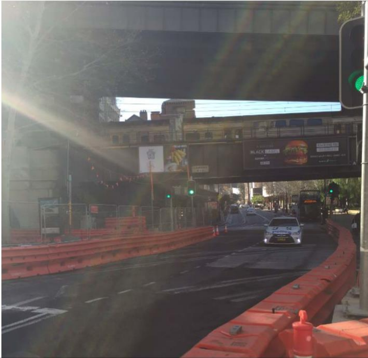
Alternate view of SLR works approx 50m south of Access point
