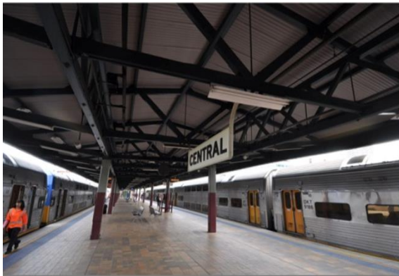
Figure 2: Typical original awnings on the Sydney Terminal platforms and the c.1998 brick paving tiles (Source: Rappoport, 2013).
